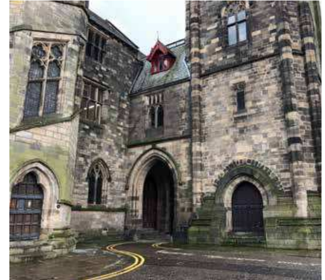
Existing door to south elevation of tower
