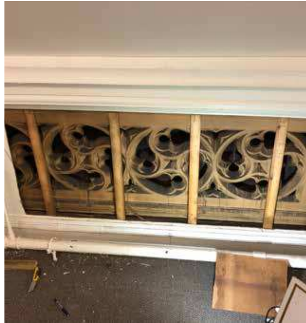
Original features within Bright Hall revealed during opening up works
