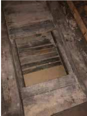
Opening up works reveal later plasterboard ceilings
