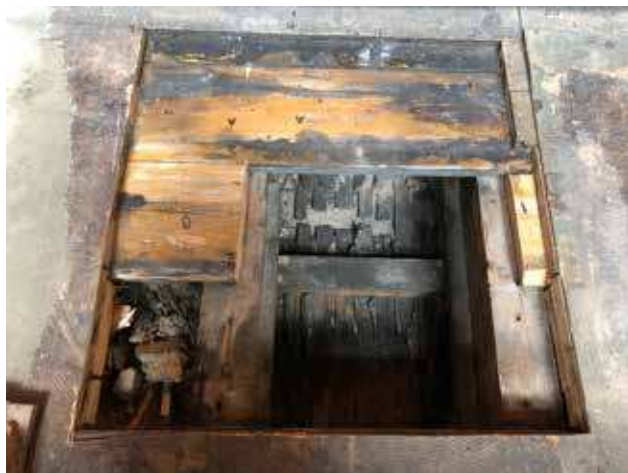
Opening up works
