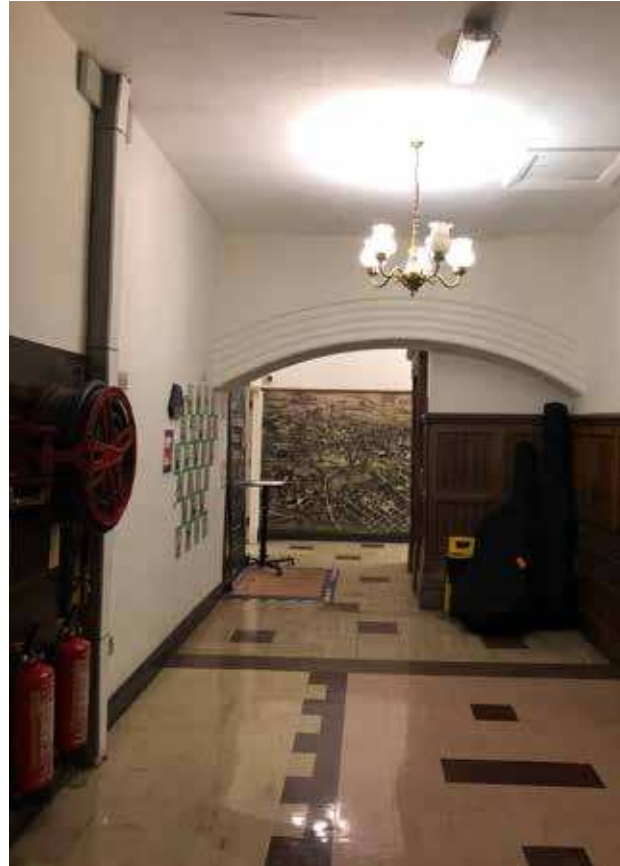
Existing lift has detrimental impact on Bright Hall features and spatial qualities
