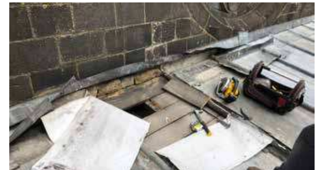
Opening Up works carried out to establish roof build up
