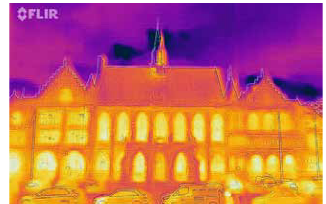
The above image shows the heat loss from the Great Hall roof
