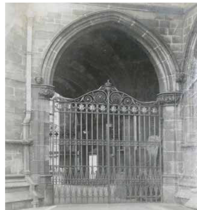
Former iron gates to porte cochere
