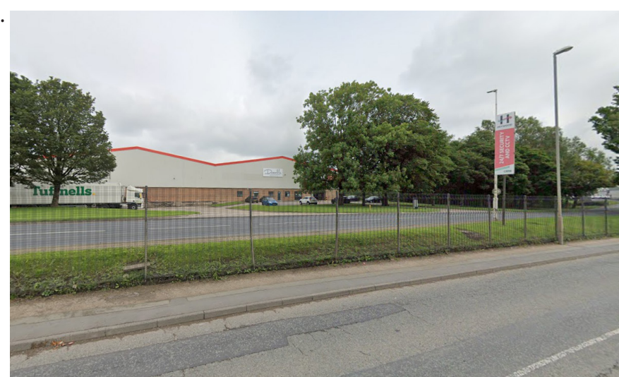
View north from Pilsworth Road across to existing industrial units
