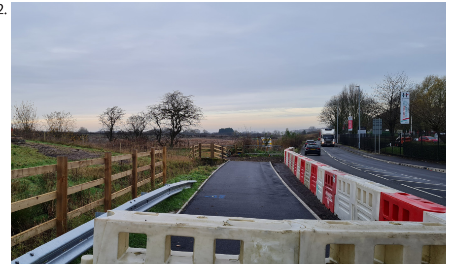
View south west along Pilsworth Road
