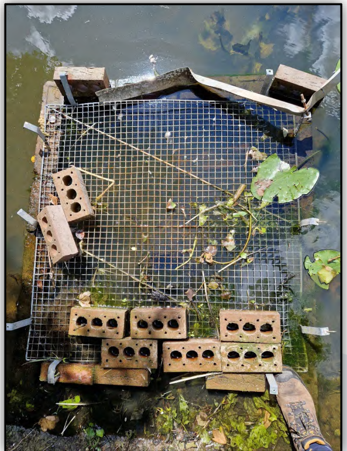
Fishery Lake Outfall Chamber & Pipe View
