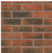
1 Red Multi Gilt Stock Brickwork
