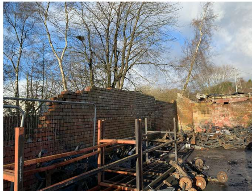
5. Demolition of existing building on site
