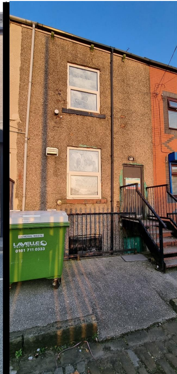
showing rear facade
