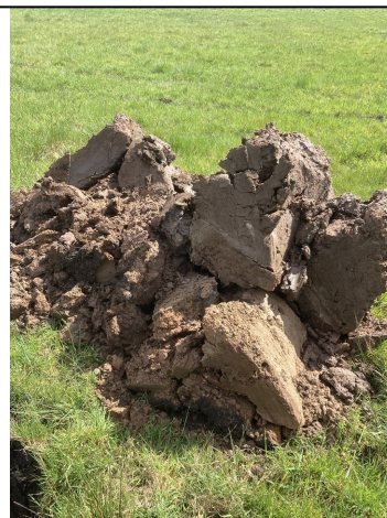
Trial Pit 125 Spoil
