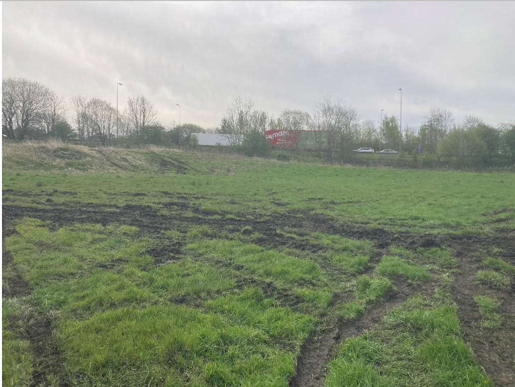
PLATE 5 SOUTH OF SITE POST WORKS
