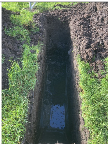
Trial Pit 115/ Soakaway 103
