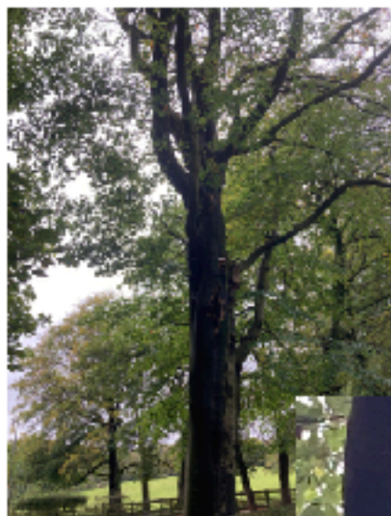
T1 showing Ganoderma, previous failed limb, rot and cavities
