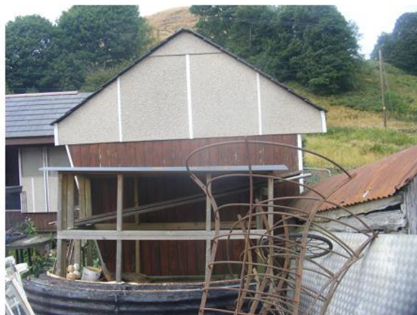
PHOTO 8 Eastern Gable of Pigeon Cote
