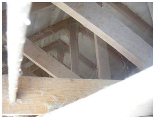
PHOTO 10 Underside of Pigeon Cote Roof
