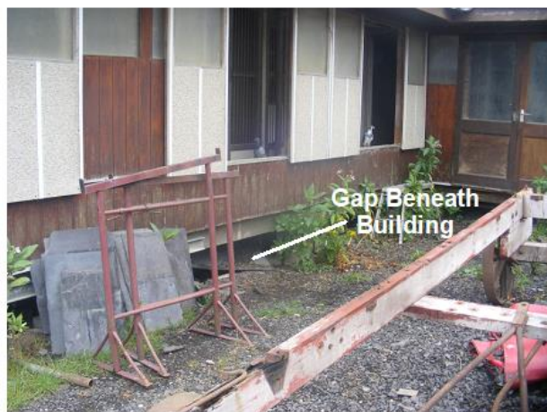
PHOTO 6 View Along Southern Elevation
