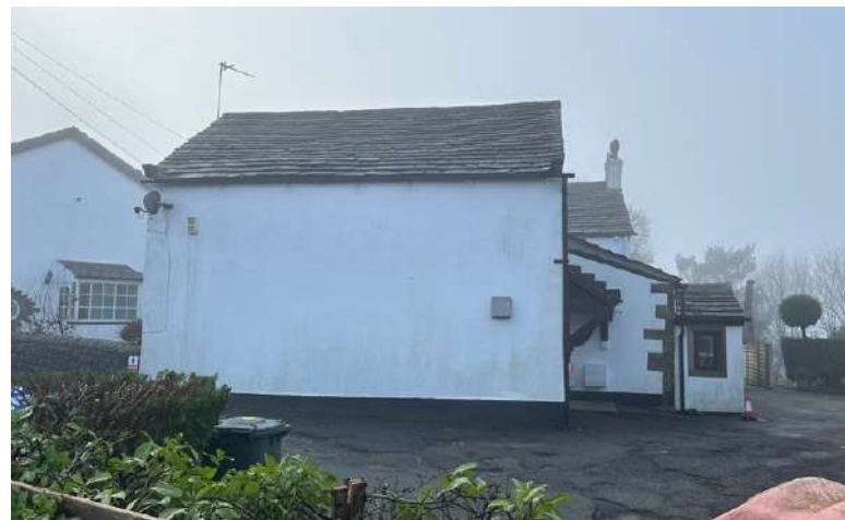
Figure 4.2: Side and Rear Elevation to Wildhouse Farm (2023)
