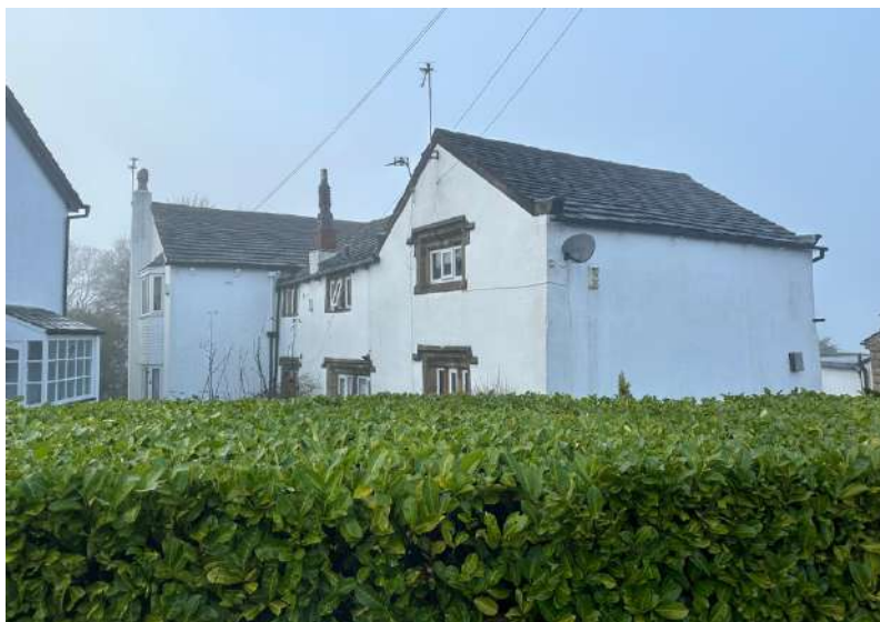
Figure 4.1: Front Elevation to Wildhouse Farm (2023)
