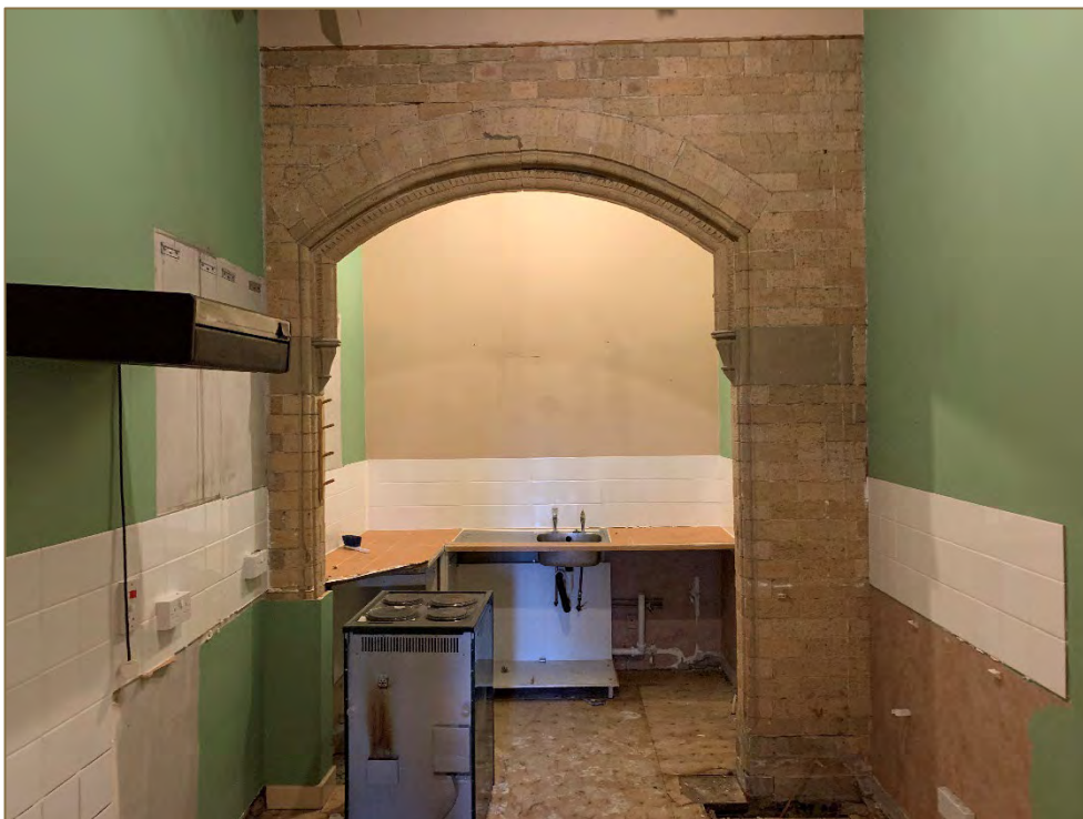
Photograph 42: View of first-floor internal kitchen.
