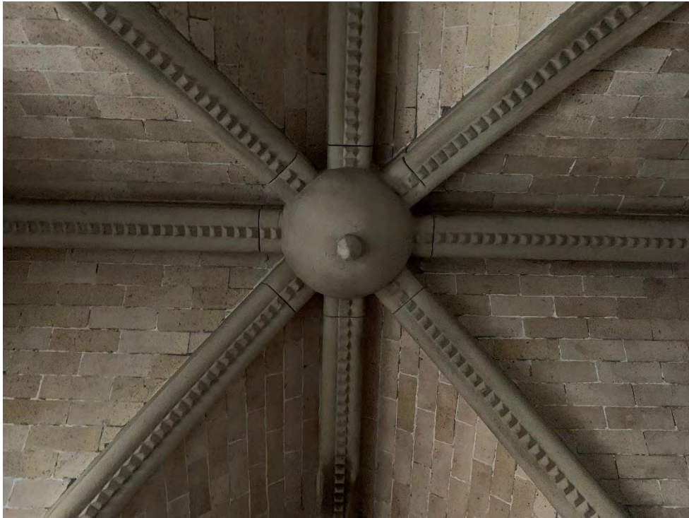
Photograph 37: View of vaulted ceiling.
