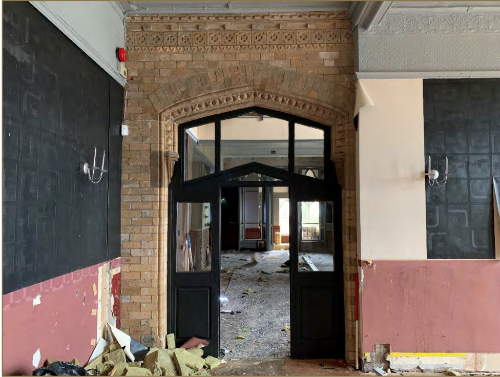
Photograph 31: View of eastern doorway into function room.
