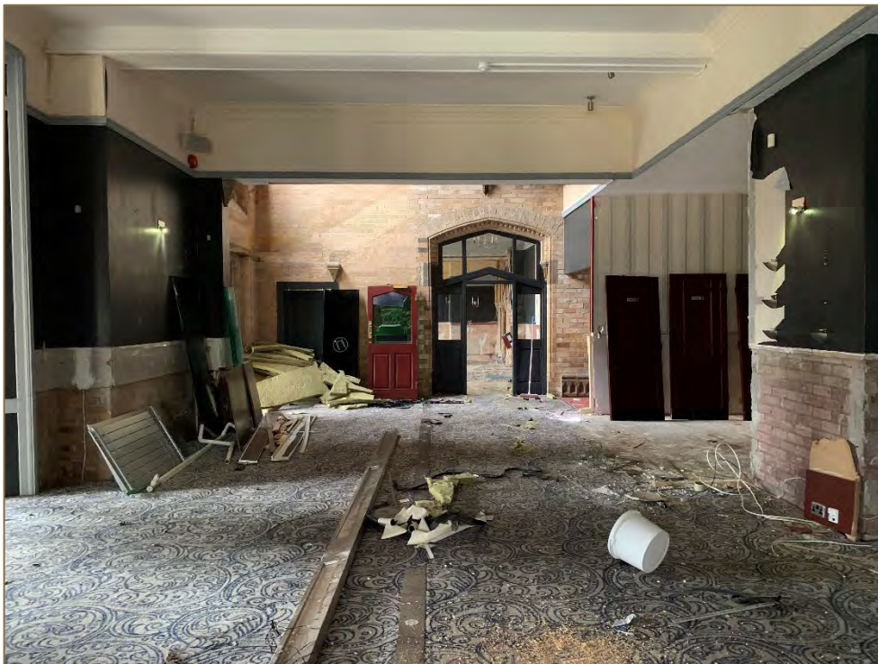
Photograph 30: View across internal dining room west.
