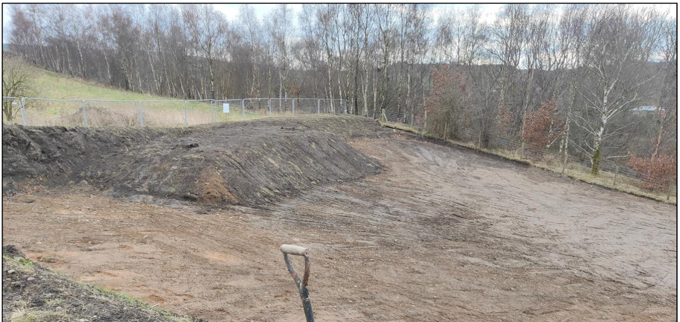
Photograph 1: General site arrangement and topsoil stockpile on site.
