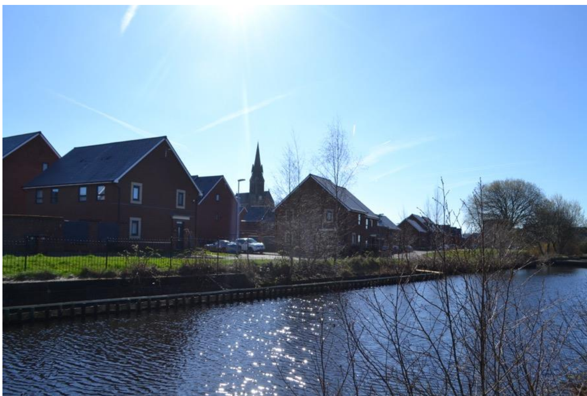
Plate 28: Sightline to the south-east from the Rochdale Canal towpath. The Church of St Martin (Grade II, NHLE ref. 1203230) is prominent in the sightline.
