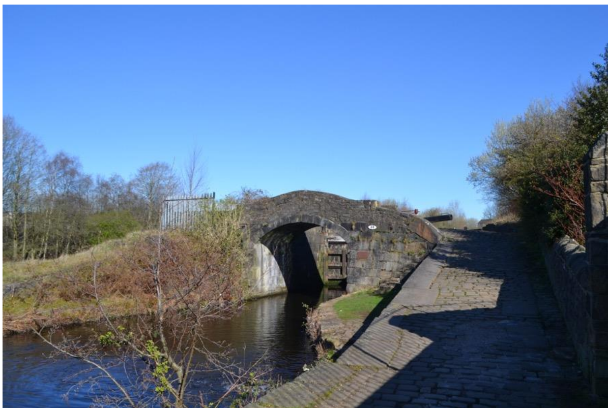
Plate 33: Sightline to the north-west towards the Rochdale Canal Lock No. 52 and Towpath Bridge (Listed Building Grade II, NHLE ref. 1038295)
