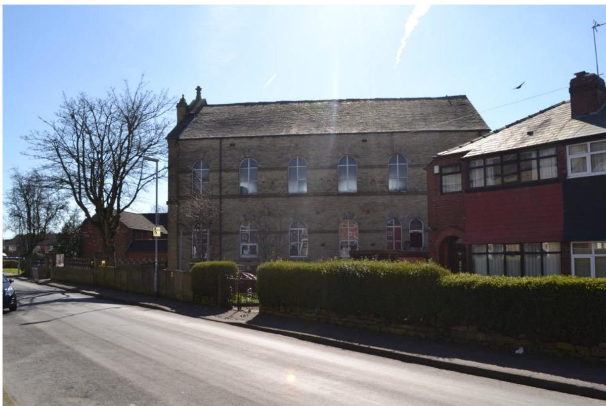
Plate 59: Sightline to the south-east from Heywood Road towards the north-east facing elevation of United Reform Church, Heywood Road (Grade II, NHLE ref. 1084281). The proposed development would have no visual influence on this sightline.
