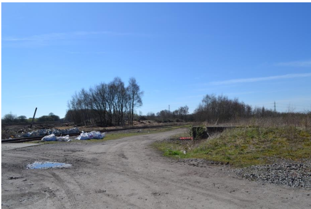
Plate 17: Sightline to the south-west across the Site showing concrete structure (platform).
