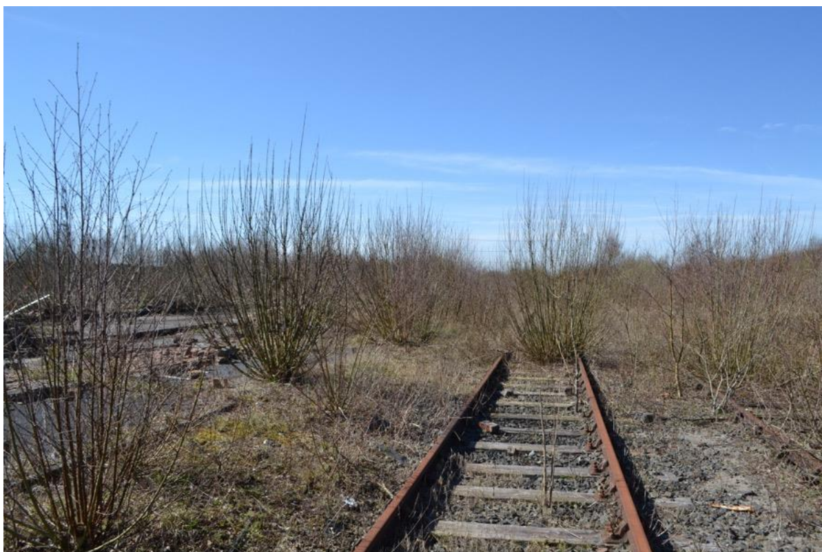
Plate 7: Sightline to the west across the Site highlighting surviving rails and sleepers.
