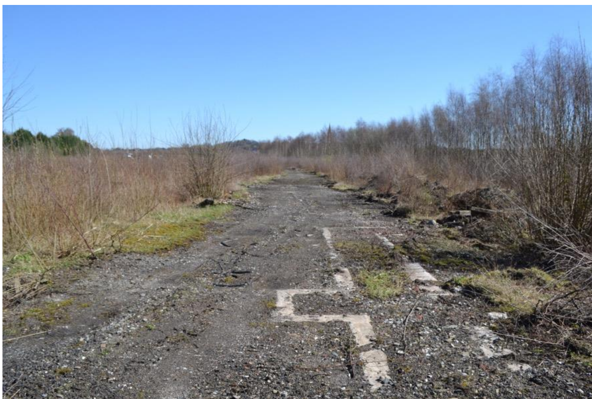
Plate 10: Sightline to the east across the Site showing outcropping relict foundations
