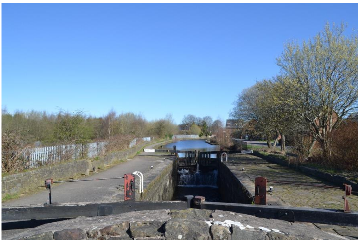
Plate 31: Sightline to the north from the Rochdale Canal Lock No. 52 and Towpath Bridge (Listed Building Grade II, NHLE ref. 1038295)
