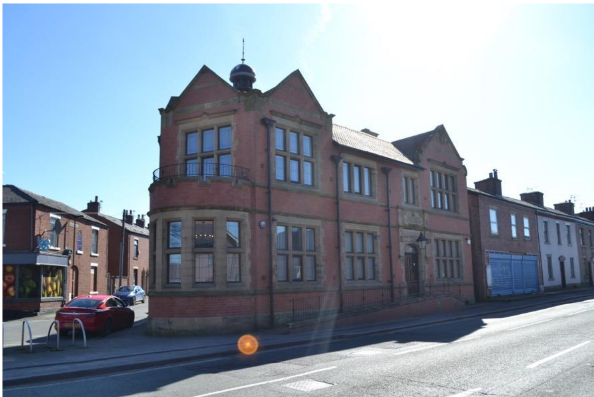
Plate 52: Sightline to the south-east from Manchester Road within the Castleton South Conservation Area towards the Carnegie Library (Non-Designated Heritage Asset)
