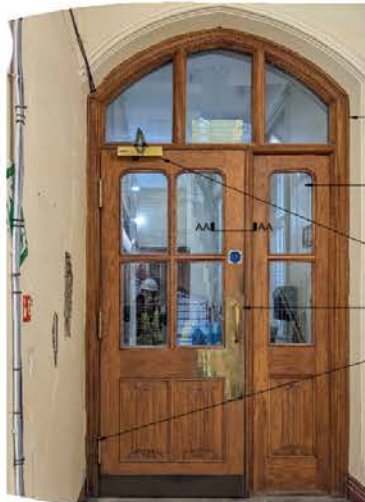
View from Stair F10
