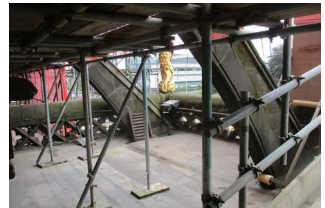
4.16b Porte Cochere roof
