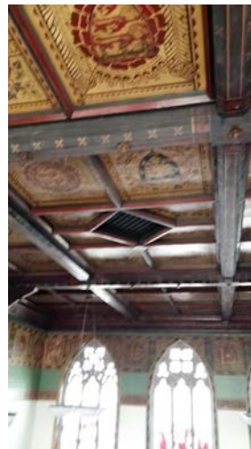
4.23 Existing Council Chamber ceiling looking to gallery
