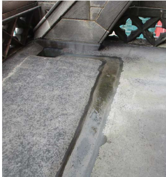
4.16c Porte Cochere roof
