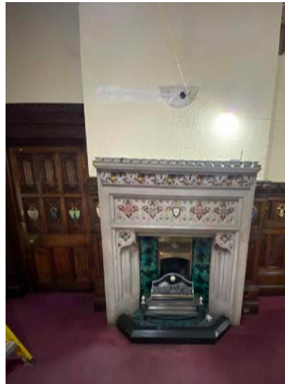
4.27 Mayors Parlour - existing condition
