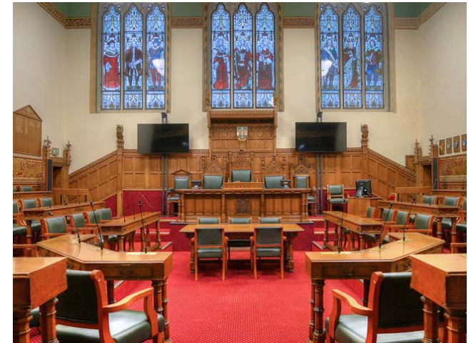
4.20 Existing Council Chamber looking to the dais
