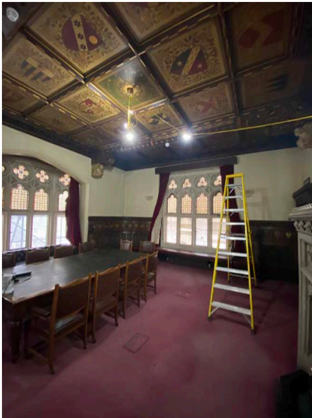
4.26 Mayors Parlour - existing condition
