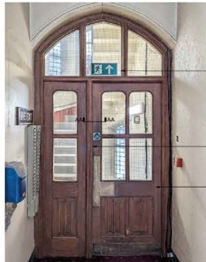
View from Lobby F11c
