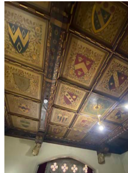
4.30 Mayors Parlour - existing condition
