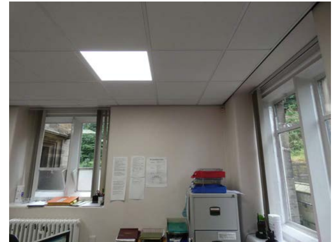
4.3 View south showing suspended ceiling
