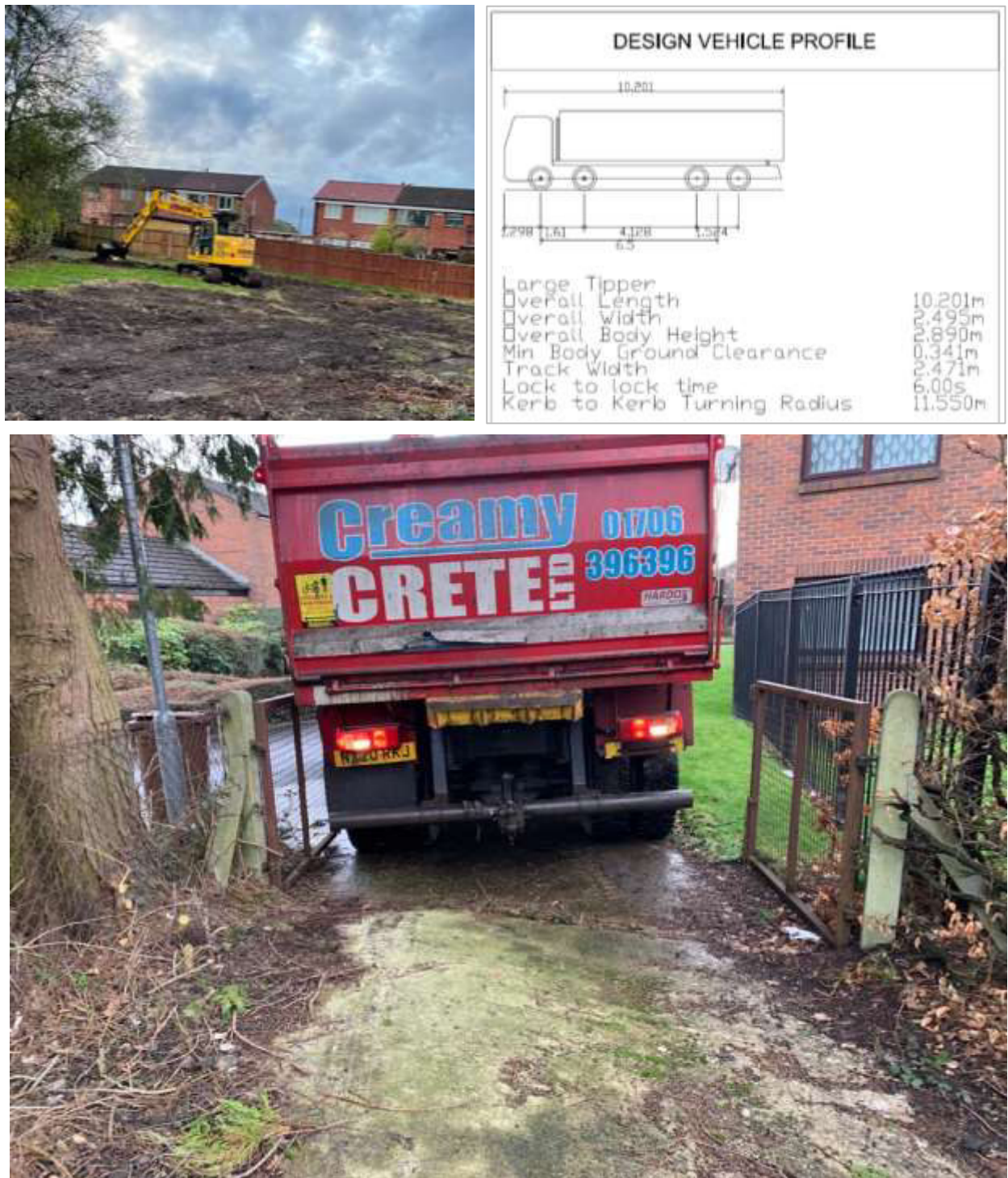
Figure 3 – Photo of Excavator and Tipper On-Site and Construction Vehicle Specification
