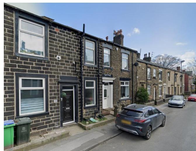
Hare Hill Road facing East – Traditional features, sandstone walls.
