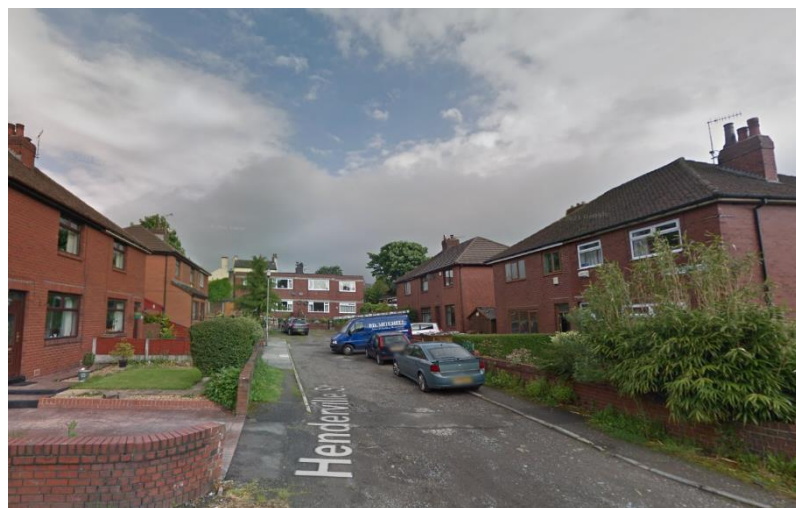
Henderville Street to the North of the application site – Red brick and modern features.
