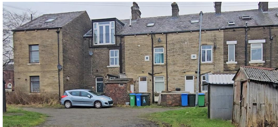
View North from application site – continuous row of linear built form.
