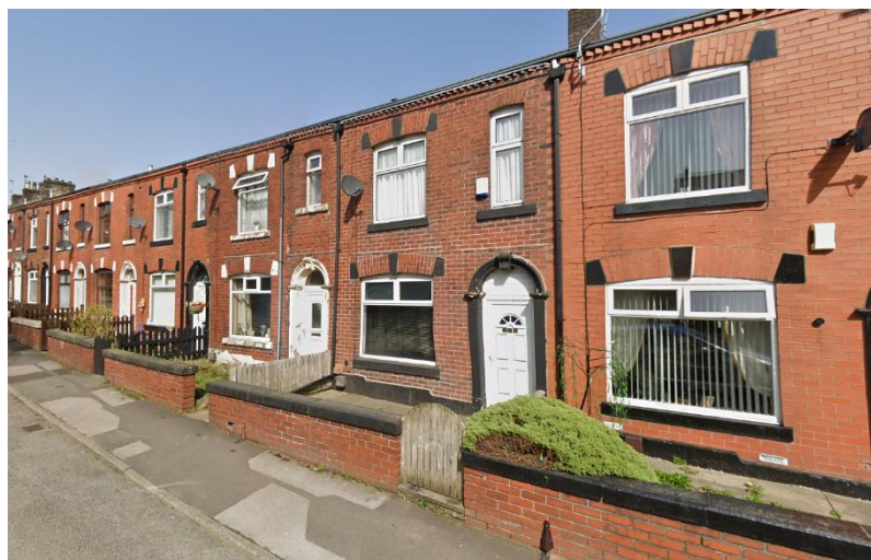
Hare Hill Road facing North – Traditional features, red brick walls.
