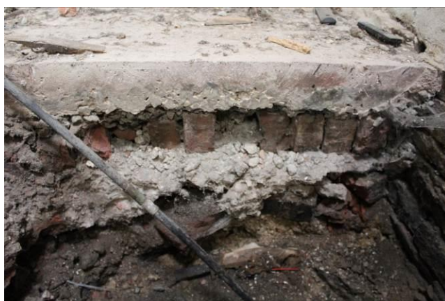
Photo 16: Interior of Barn B, Floor detail, looking SW and downward
