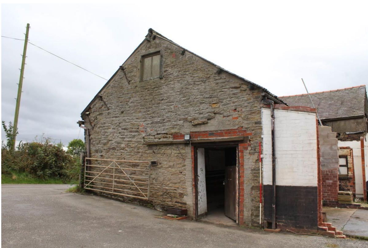
Photo 7: Detail side elevation of Barn A; a window, beams support and doorway with remnants of a sliding door brackets, looking S
