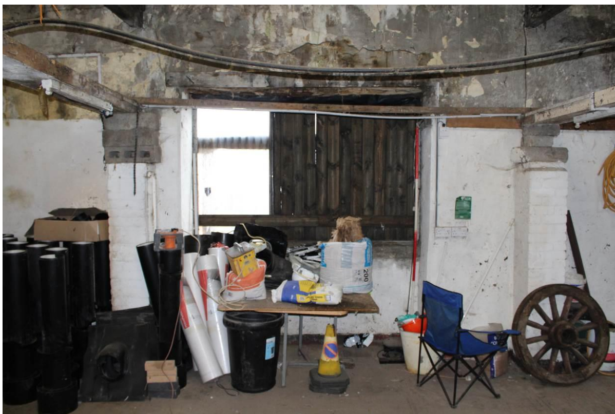
Photo 14: Interior of Barn B; Note blocked up opening, and elevated brick plinths looking NE
