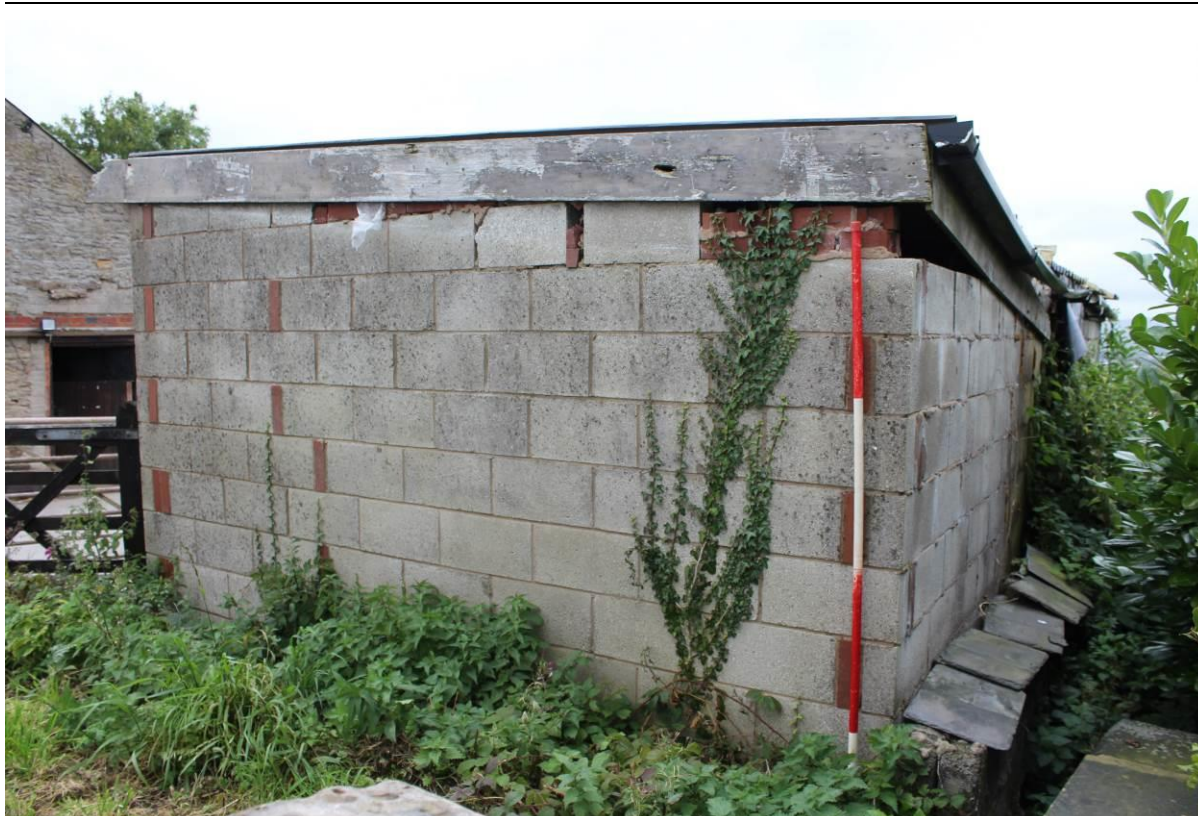
Photo 44: General View of Stable Block B; side and rear elevation, looking NW
