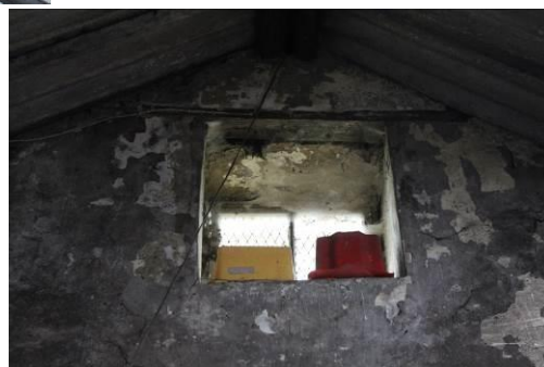
Photo 13: Interior of Barn B; note window detail on Barn B, looking NE
