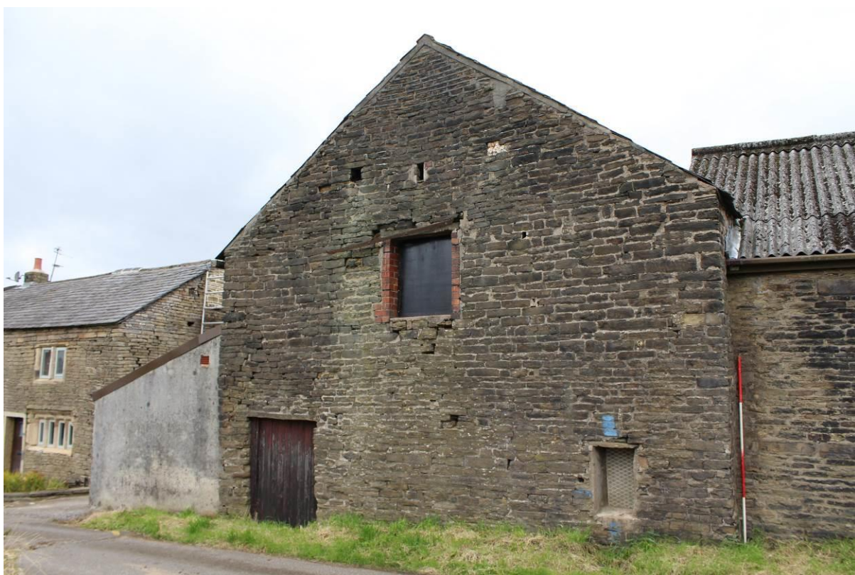
Photo 4: Front elevation of Barn B, looking NW
