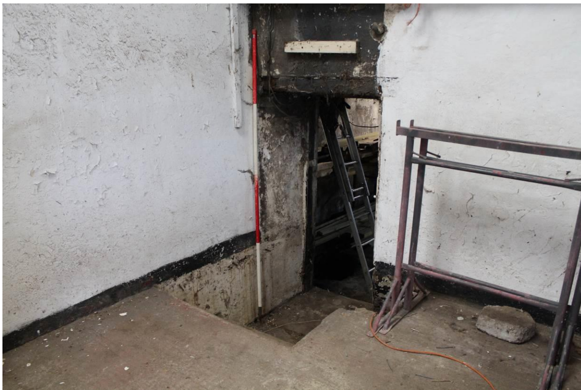
Photo 20: Interior of Barn B, looking toward Barn A, looking SW
