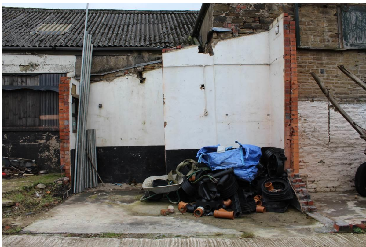
Photo 11: Rear elevation of Barn A; showing extensions partially demolished, looking SE
