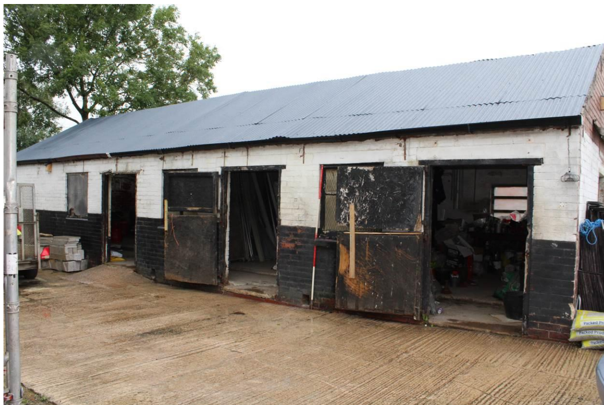
Photo 34: General View of Stable Block A, looking SE
