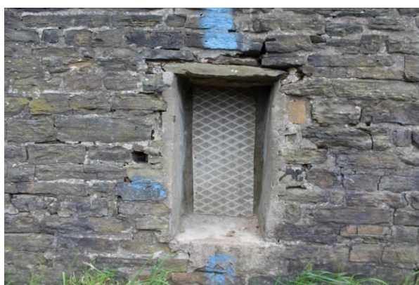
Photo 5: Detail on front elevation of Barn B; a row of ventilation holes, a boarded-up sliding door hatch, a window and a planked door, looking NW
