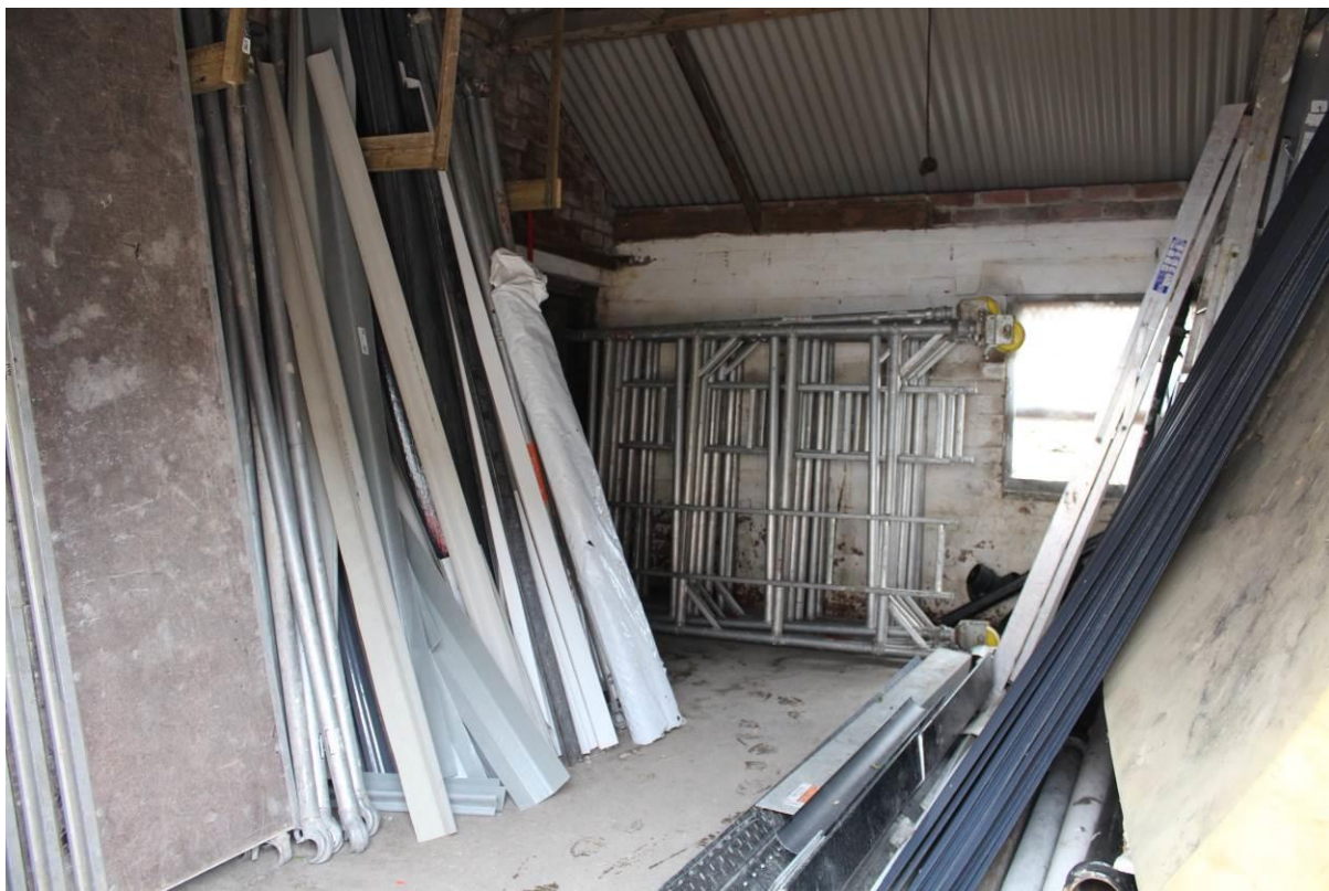
Photo 39: Interior of Stable Block A, looking NW
