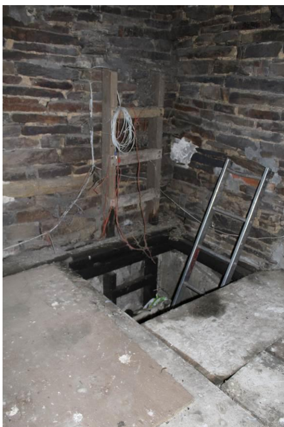
Photo 33: Interior of Barn A: General view of First Floor; showing access point; hatch and ladder, looking SE
