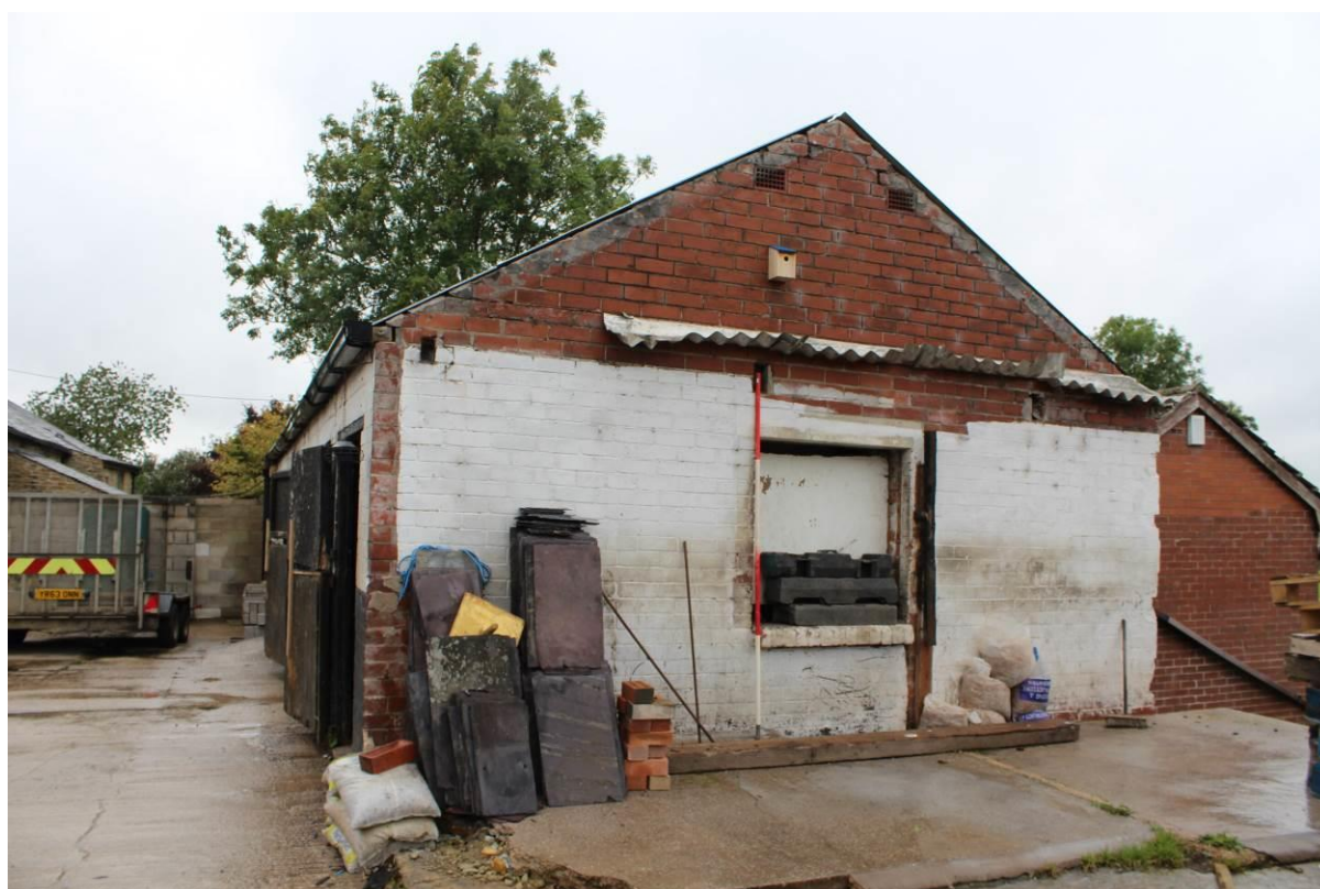
Photo 35: Side elevation of Stable Block A; showing extensions partially demolished looking W
