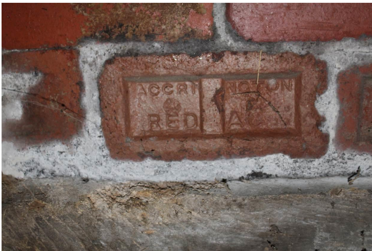
Photo 24: Interior of Barn A; blocked door detail with closeup of the upper course of bricks, looking NE
