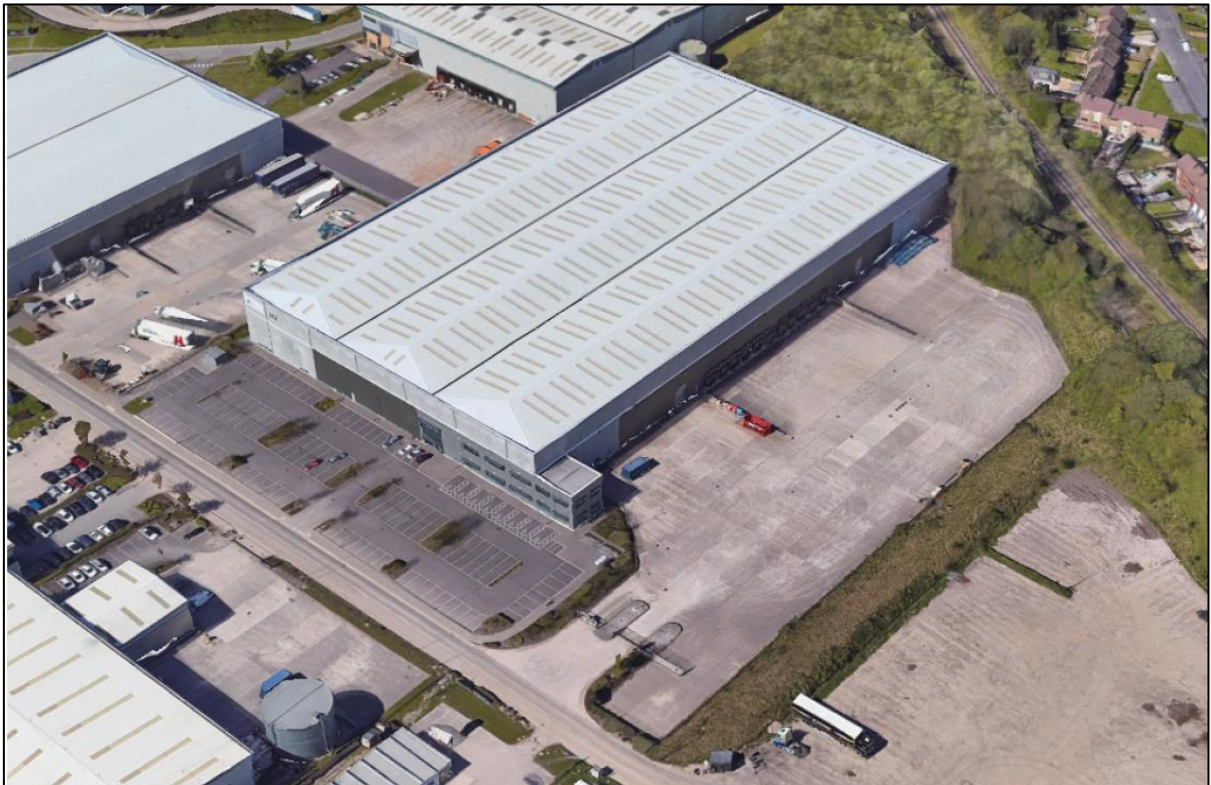
Figure 2: Existing access and warehouse at the Site
