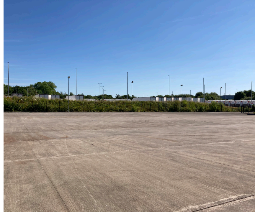
Existing service yard.
