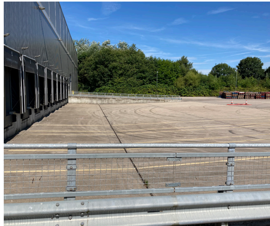
Image looking north of service yard.
