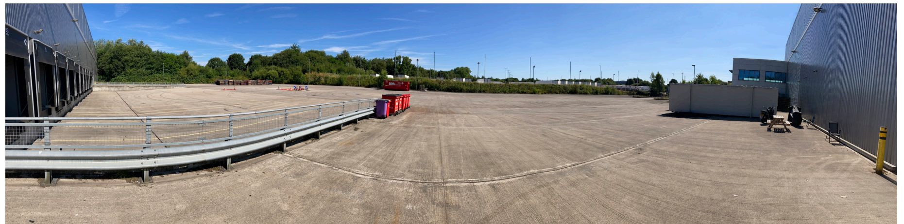
Photo looking at the service yard where majority of the works will take place.
