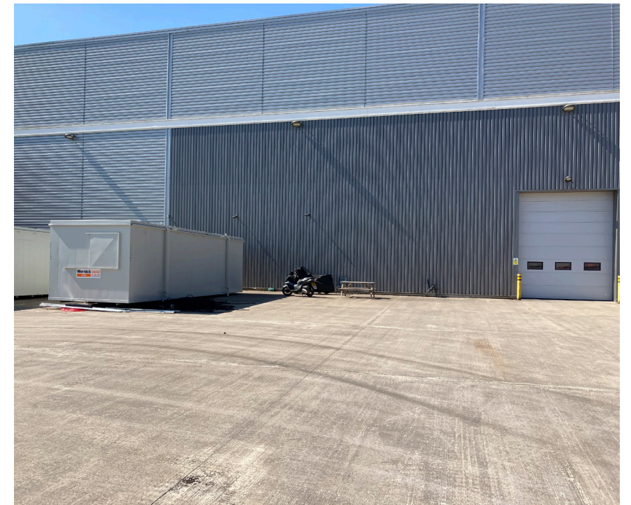
Image looking at building elevational treatment.
