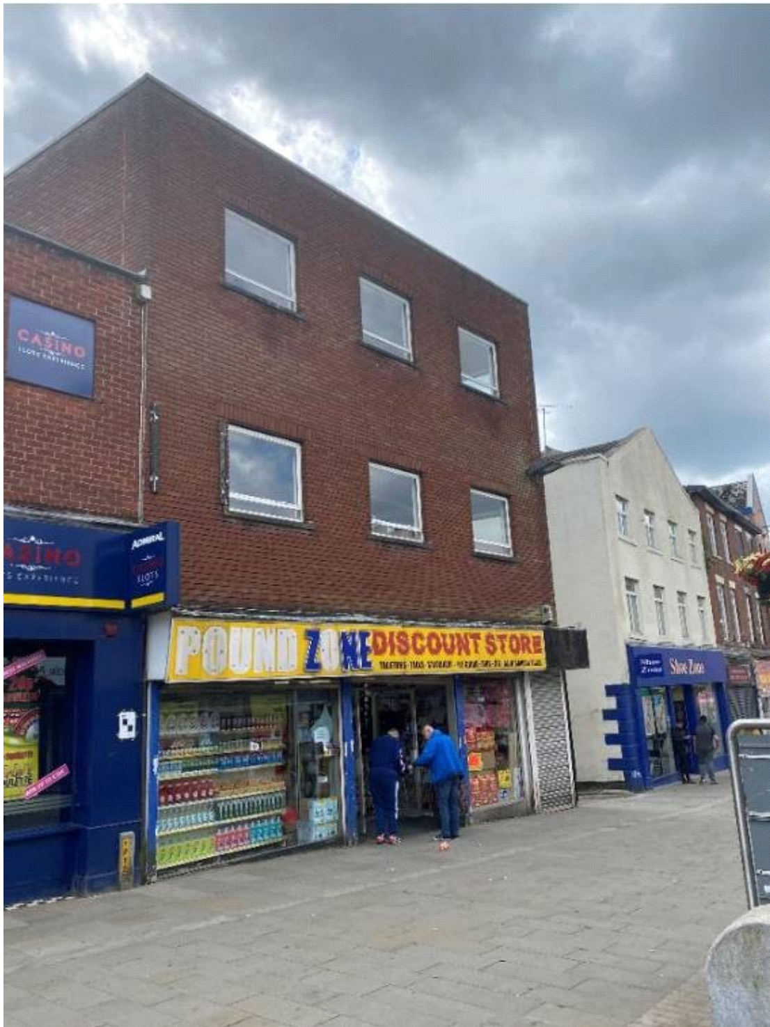
Photograph indicating the street elevation of the existing building.
