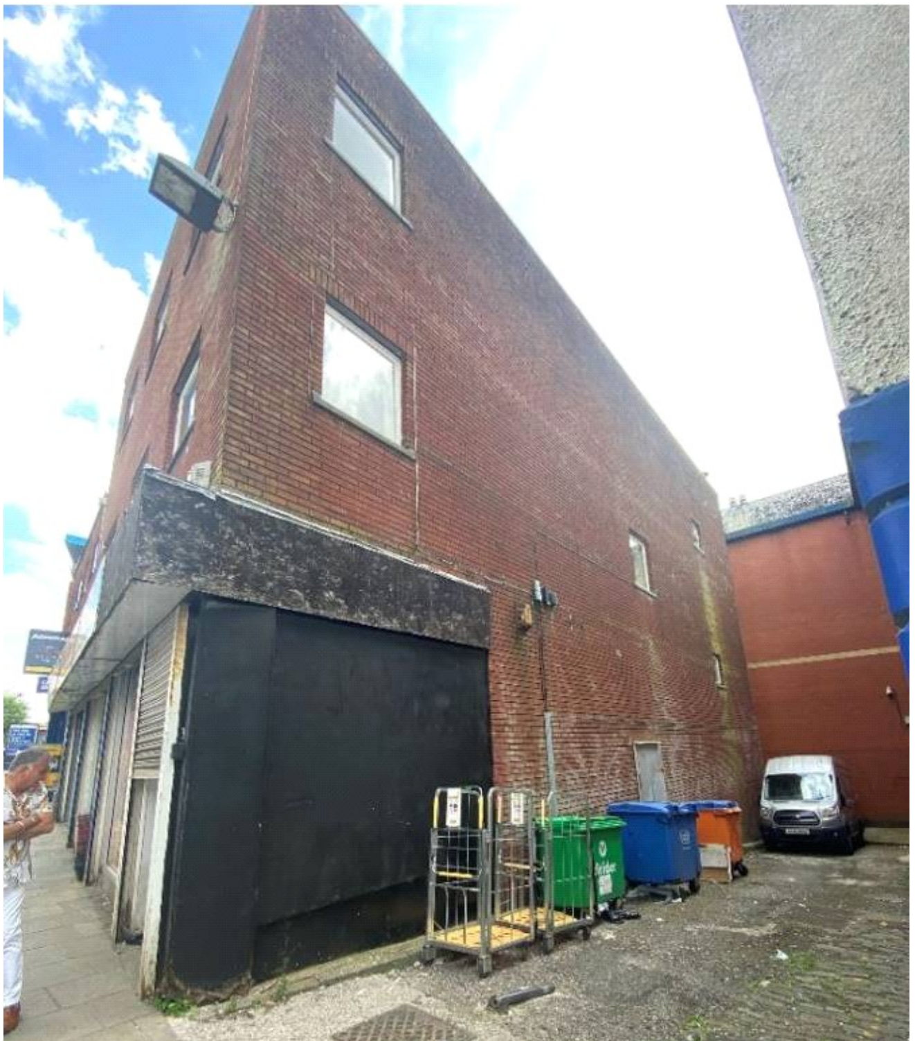
Photograph indicating current bins and loading area.
