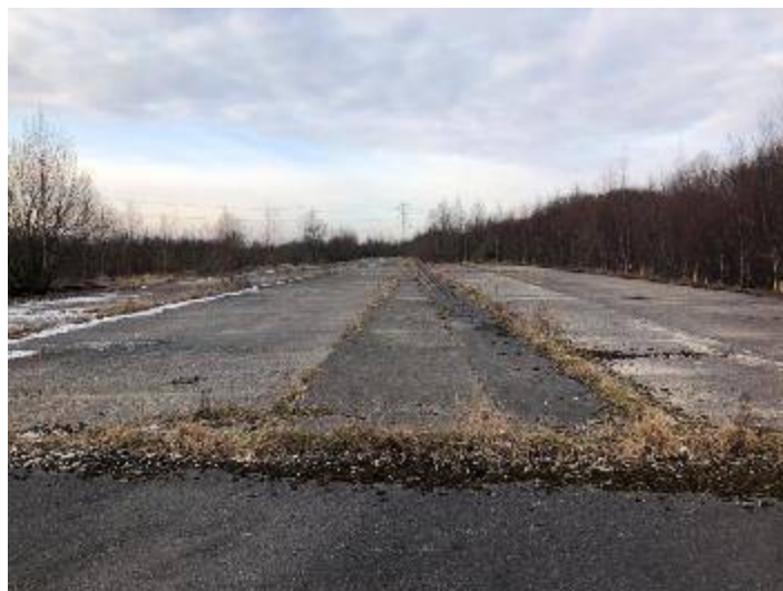
PLATE 2 SHOWING AREA OF HARDSTANDING
