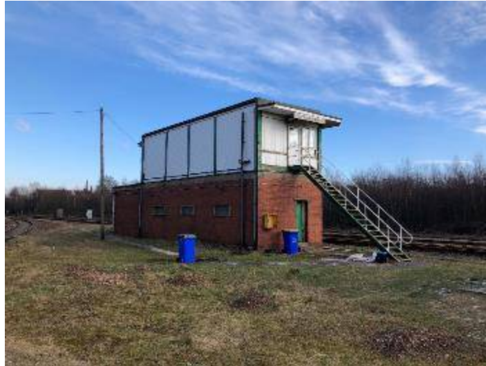
PLATE 1 SHOWING SIGNAL BOX BUILDING
