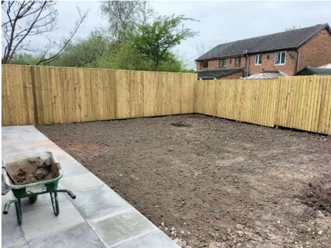
View south west across Plot 7 rear garden.
