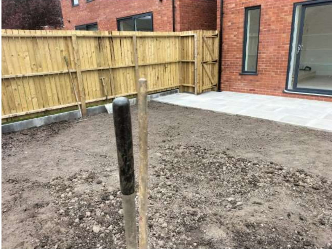
Plot 3 rear garden, looking north-west across the garden.
