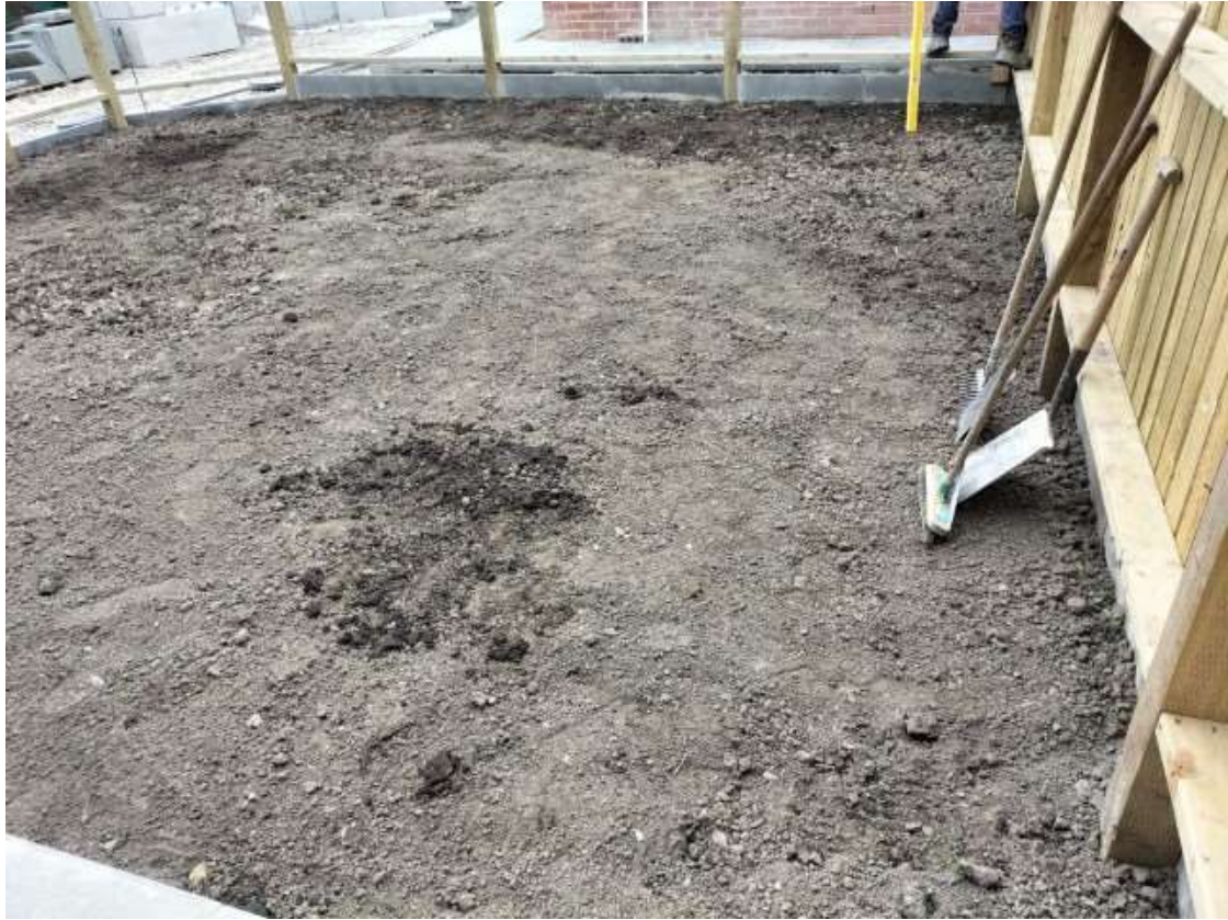
View south across Plot 3 rear garden area.
