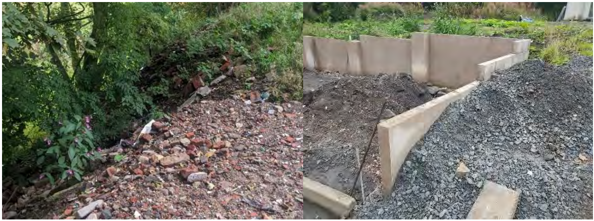
Figure 3: Photographs showing the topography of the northern site section dropping off steeply, looking northeast (left photo) and of the 2m retaining wall along the western boundary (right photo)
