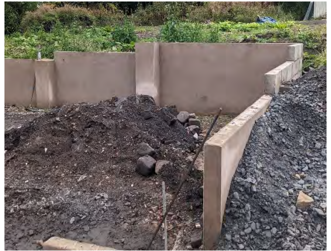
Figure 2 – A retaining wall along the western site boundary, looking east.
