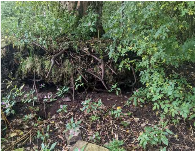
Figure 7 – Steep slopes with associated land slips and established trees in the northeastern site section, looking east.
