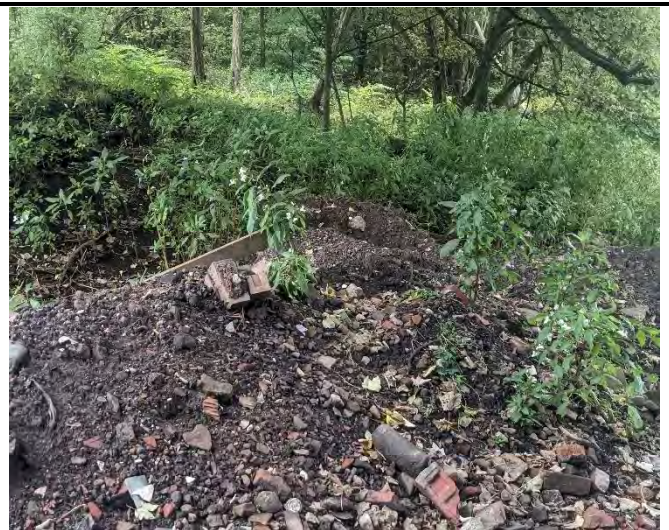
Figure 6 – On-site heaps with landslips visible in the distance, looking east.
