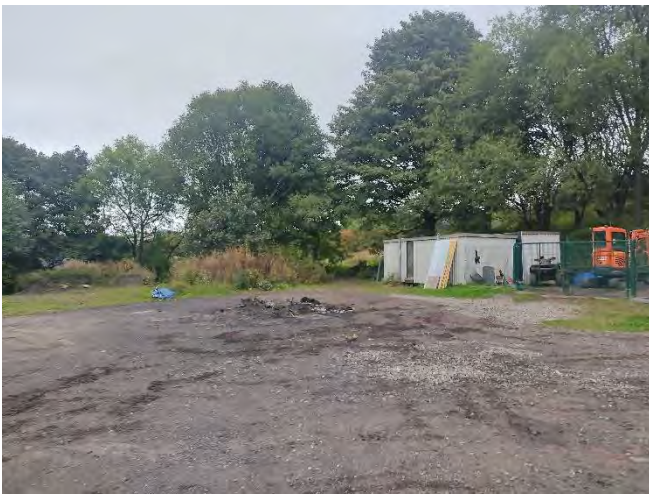
Figure 1 – The central and northern site sections, looking north.
