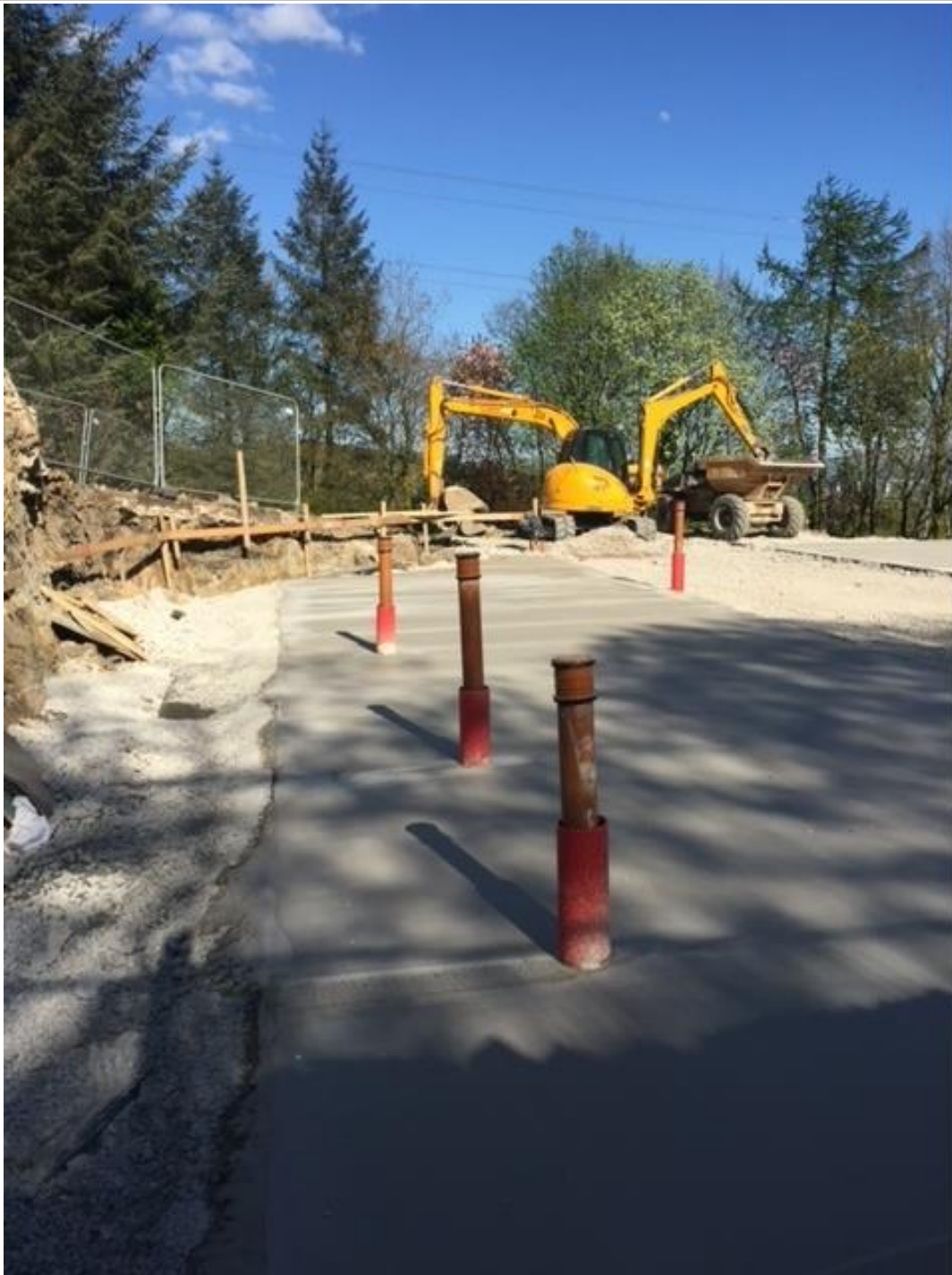
FIGURE 7 INSTALLATION OF CONCRETE SLAB
