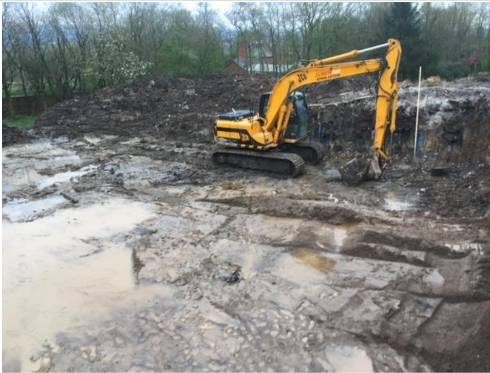
FIGURE 1 EXCAVATION OF NATURAL STRATA TO DEVELOPMENT PLATFORM LEVEL
