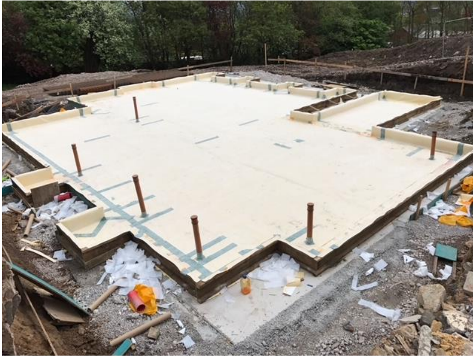
FIGURE 9 INSTALLATION OF MEMBRANE
