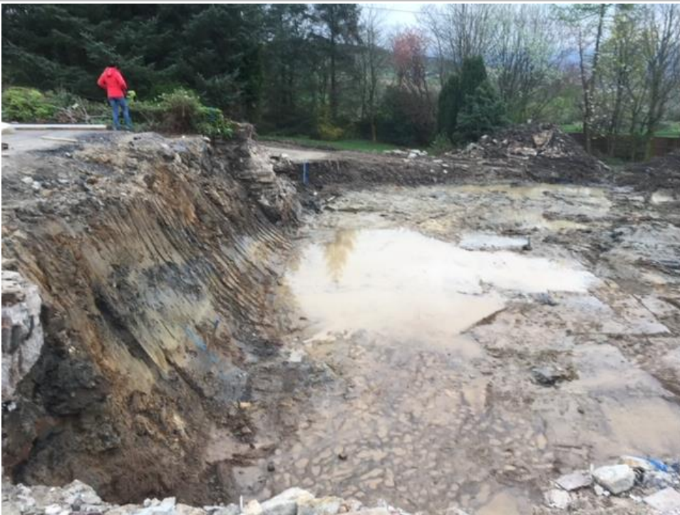
FIGURE 2 EXCAVATION OF NATURAL STRATA TO DEVELOPMENT PLATFORM LEVEL
