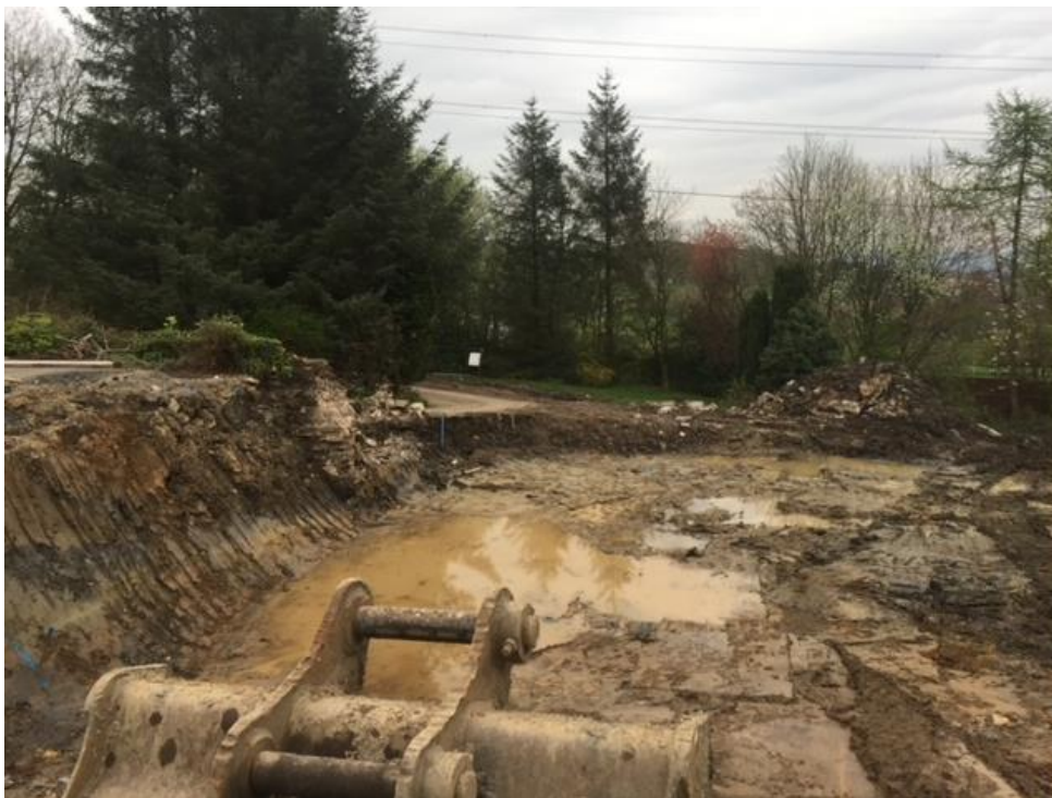
FIGURE 4 EXCAVATION OF NATURAL STRATA TO DEVELOPMENT PLATFORM LEVEL
