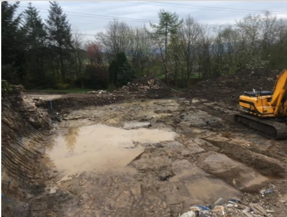
FIGURE 3 EXCAVATION OF NATURAL STRATA TO DEVELOPMENT PLATFORM LEVEL
