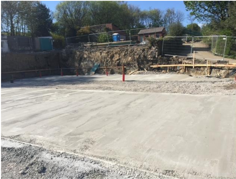
FIGURE 6 INSTALLATION OF CONCRETE SLAB
