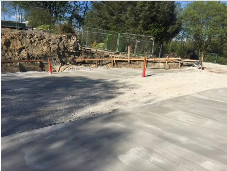
FIGURE 6 INSTALLATION OF CONCRETE SLAB
