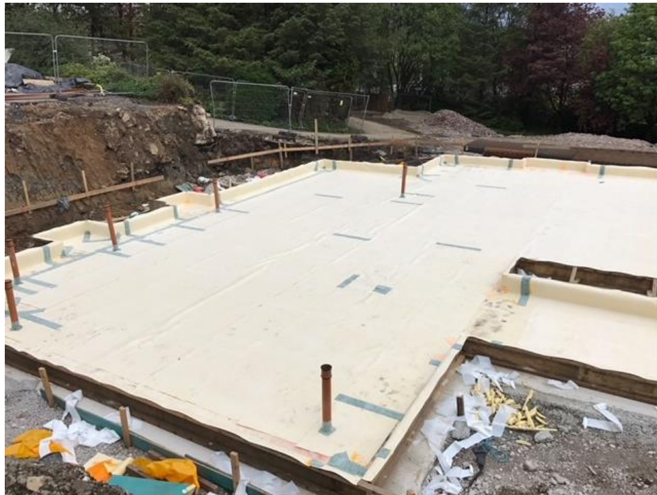
FIGURE 10 INSTALLATION OF MEMBRANE
