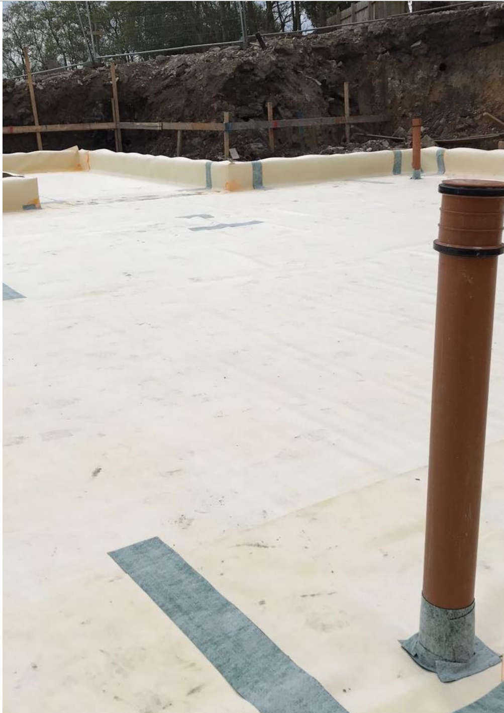
FIGURE 8 INSTALLATION OF MEMBRANE
