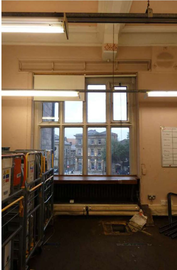
F6c. One of the east windows.
