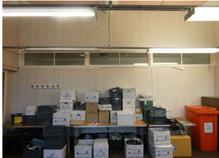
F6c. View west, the inserted partition cuts accross historic features.
