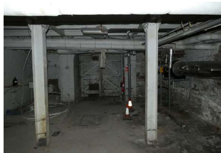
Cast-iron structure in the basement.
