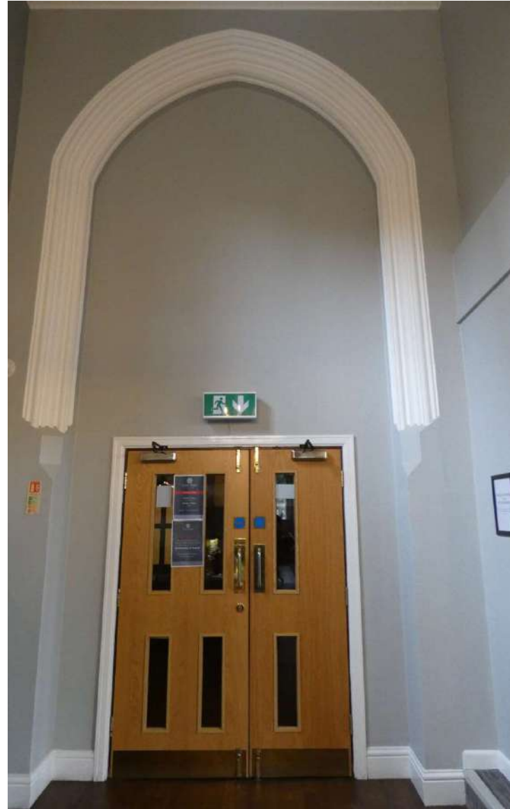
G6. Door in north wall to G2h.
