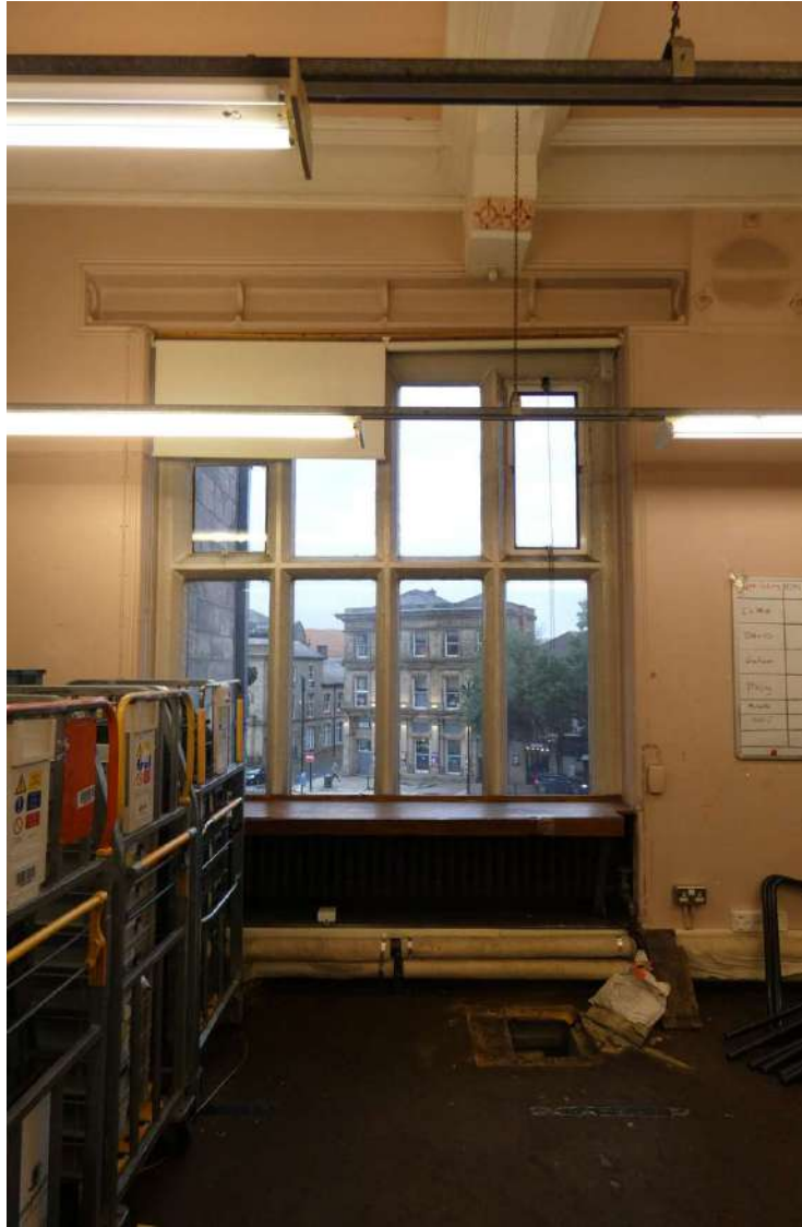
F6c. One of the east windows.
