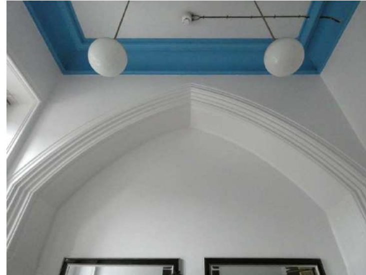
F6f. Filled arch to N.
