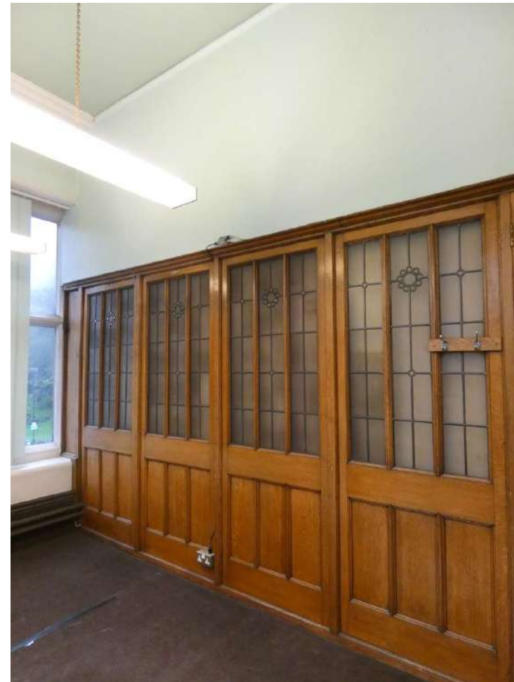
F6d. Partition inserted accross window mullion.
