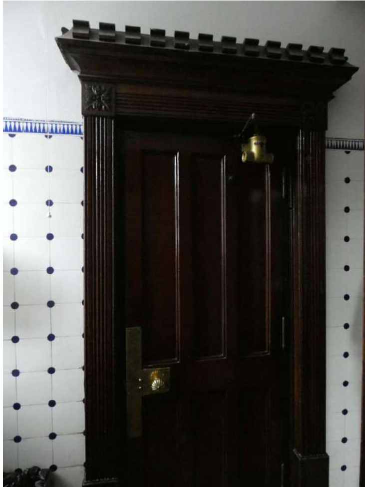
F6f. Original door and architrave.
