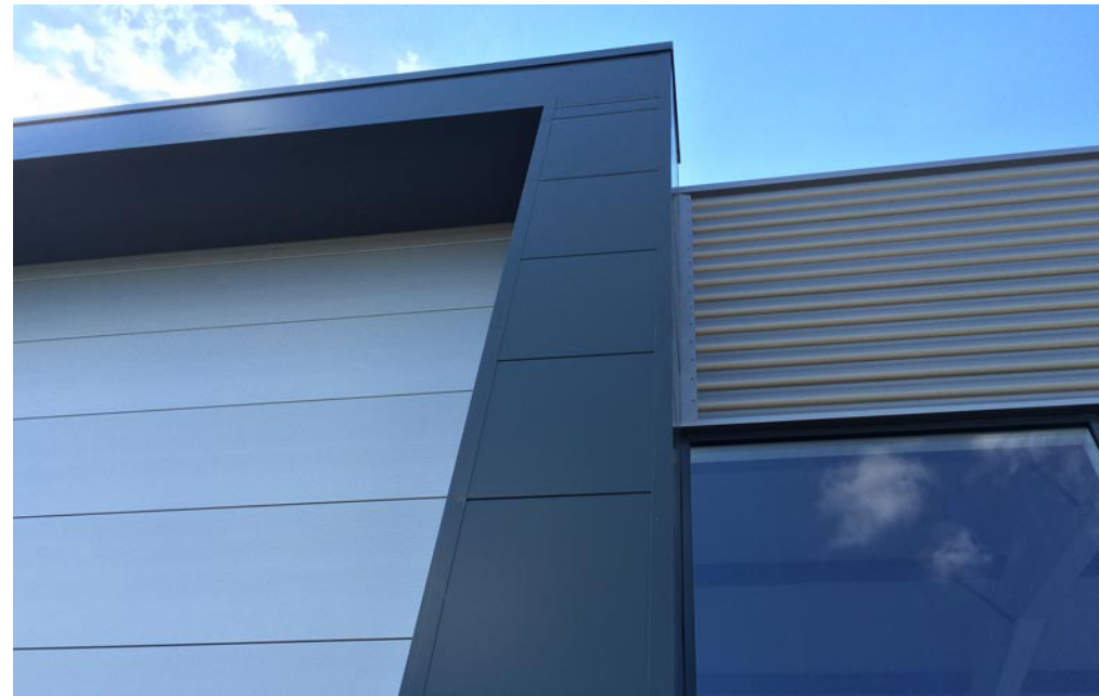
Above: Flat panel cladding to office areas with deep reveals provide a contrast to the adjacent horizontal profiled cladding
