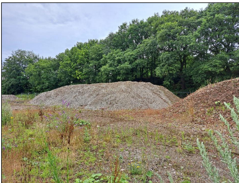
Photograph 12 showing the spoil heaps on site
