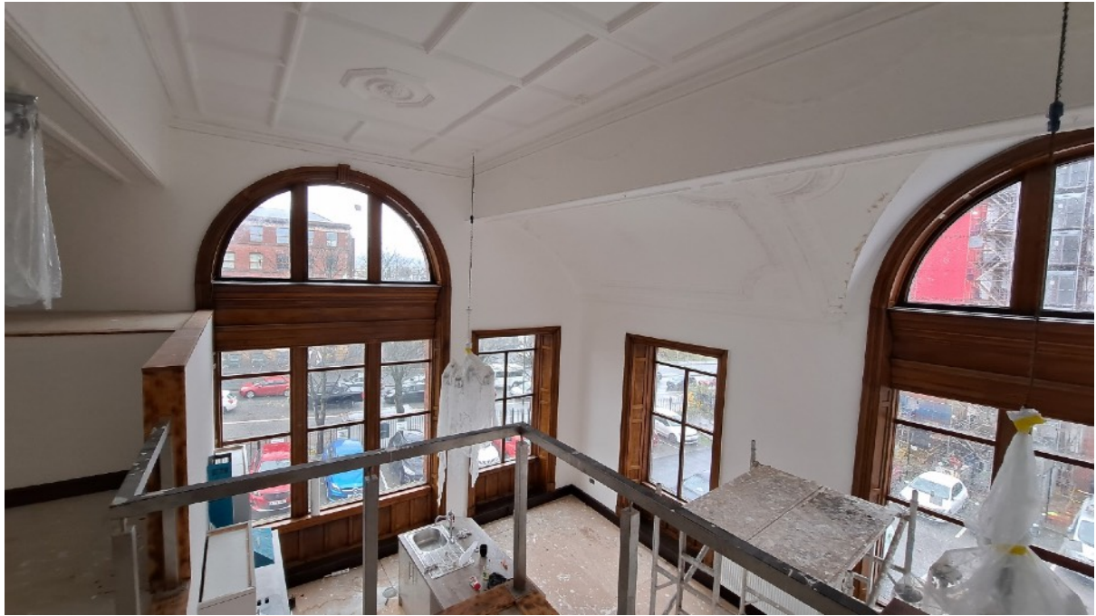
Plate 56: The full height of the Board Room has been used in Apartment 13 with the introduction of a mezzanine floor
