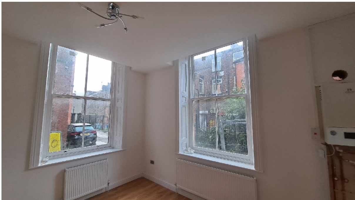
Plate 31: Former office that was converted to form toilets (G16 and 17). Partitions removed to form Room 6 of Apartment 4. Retained window and surrounds with bulkheads, but apparently altered, and panels removed
