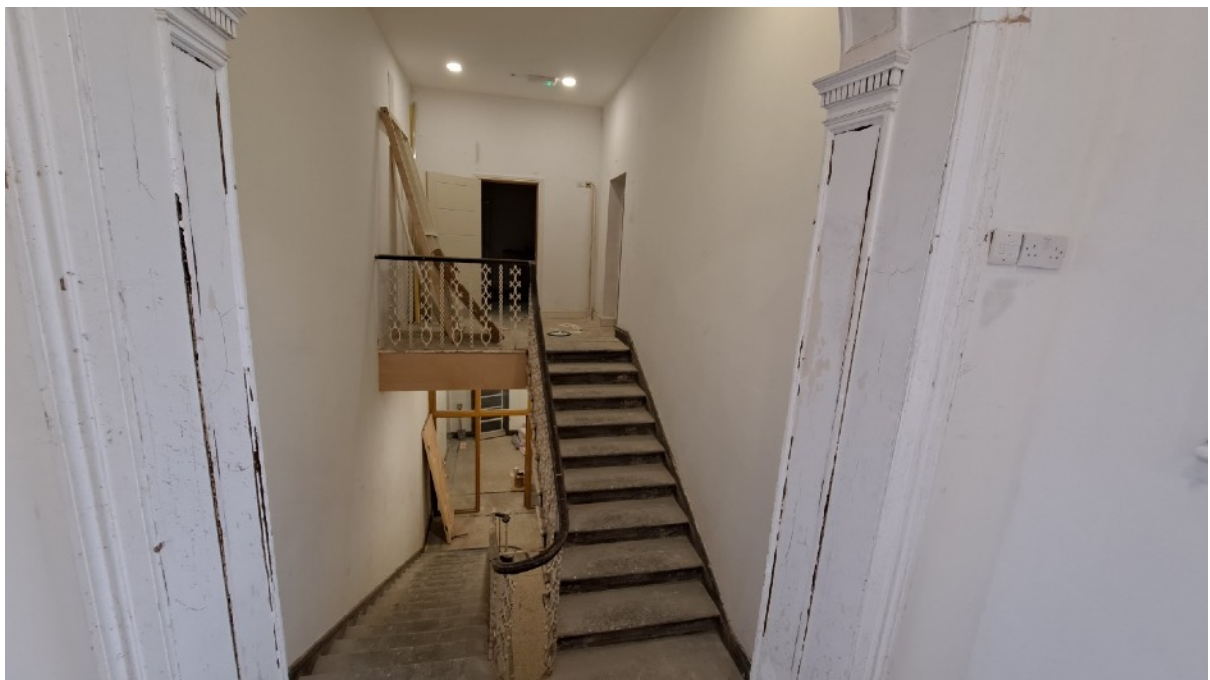
Plate 37: Looking to the upper stairway and the landing (F6), now forming CF01
