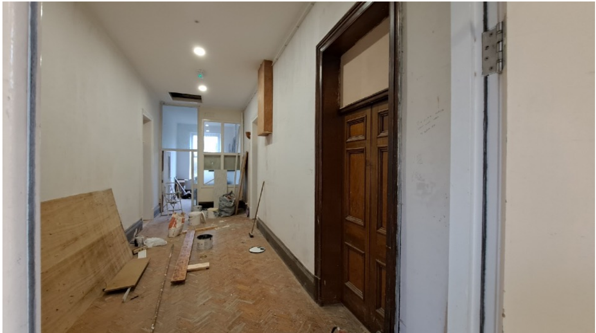
Plate 47: The corbelled arch leads to the access corridor to the Board Room (F13), now CF04. High quality finishes including skirting and door surrounds have been retained with original Board Room door
