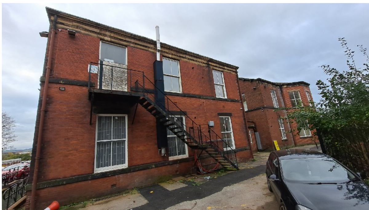
Plate 6: The rear elevation of the extension looking south-east
