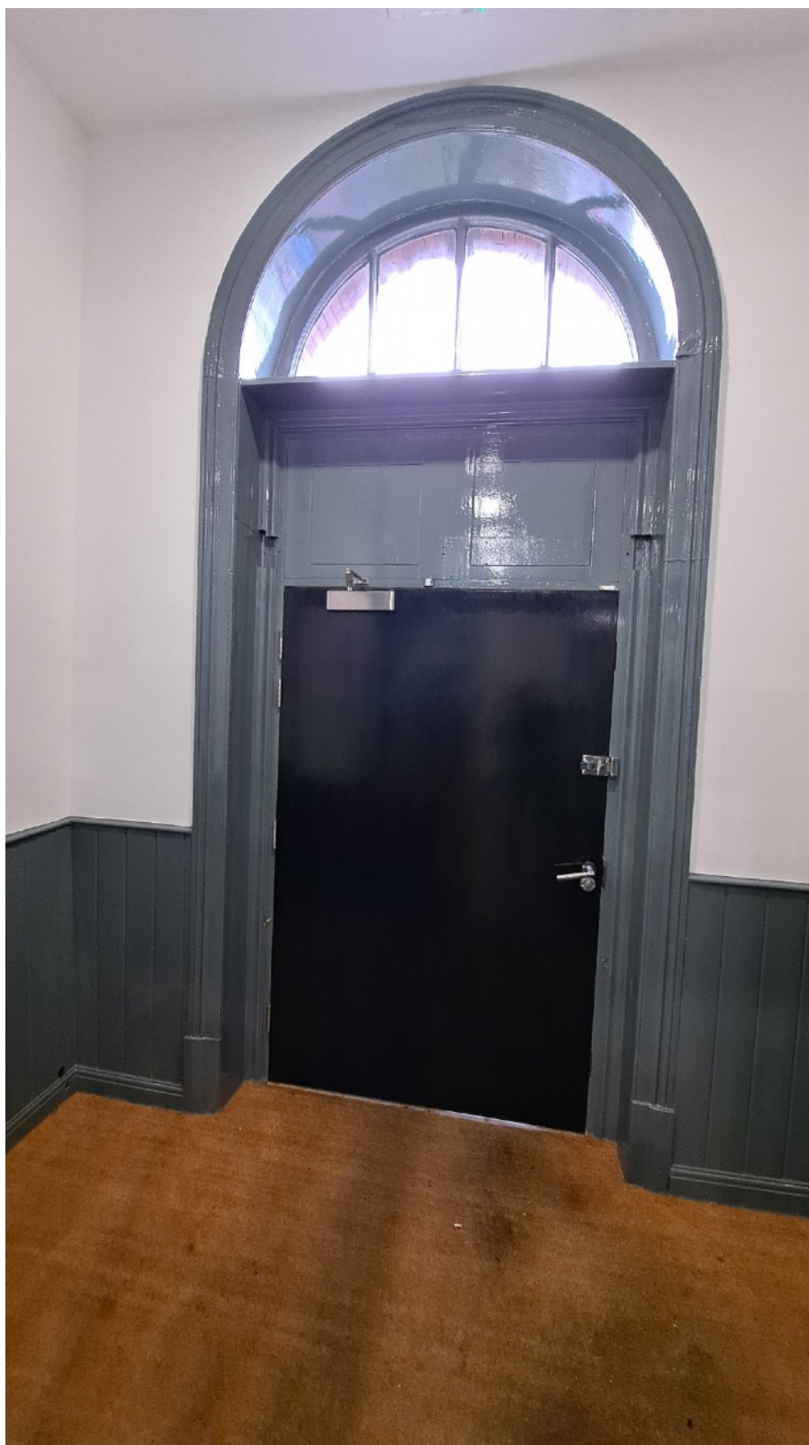
Plate 32: Main entrance to extension with retained door surround and fanlight but replaced door. The vestibule retains its match boarding to dado. Formerly G23 now CG05
