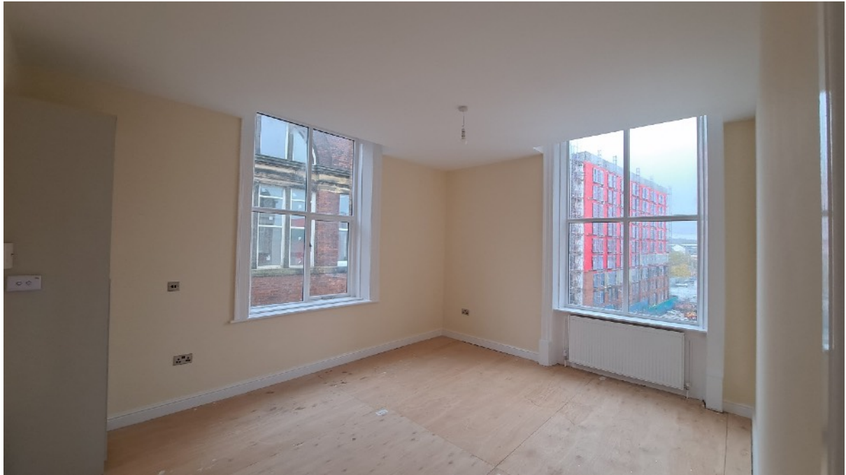
Plate 42: Former bedroom (F7) now Room 2 Apartment 10 with partition to form corridor. Original window surrounds and panel with new frames and bulkheads
