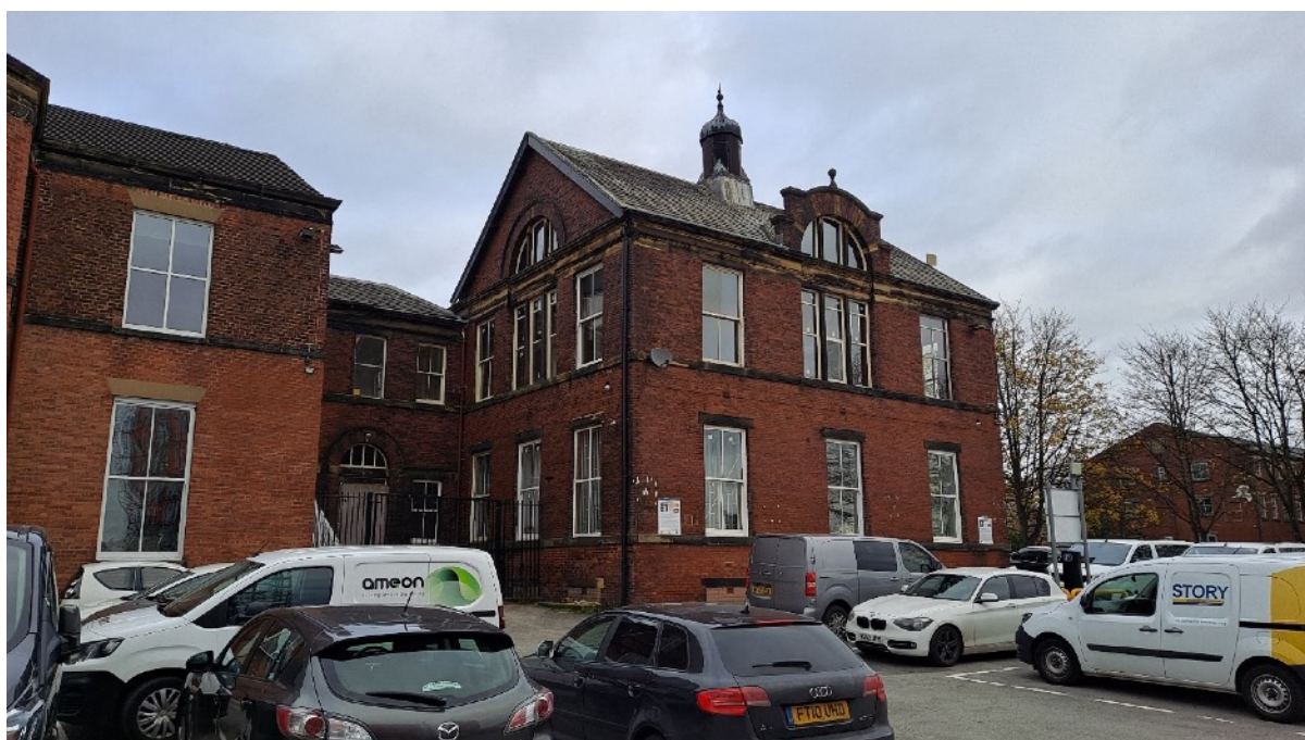
Plate 10: The extension from south-east with house and link building to left
