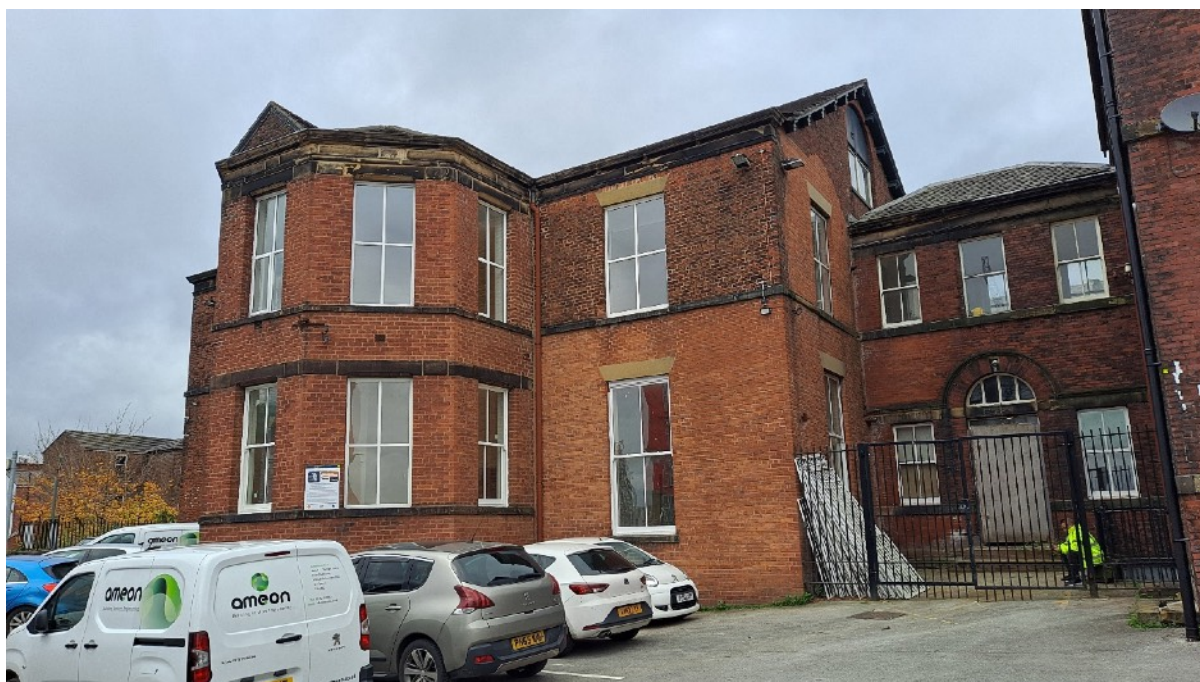
Plate 9: The house from north-east with link building to right
