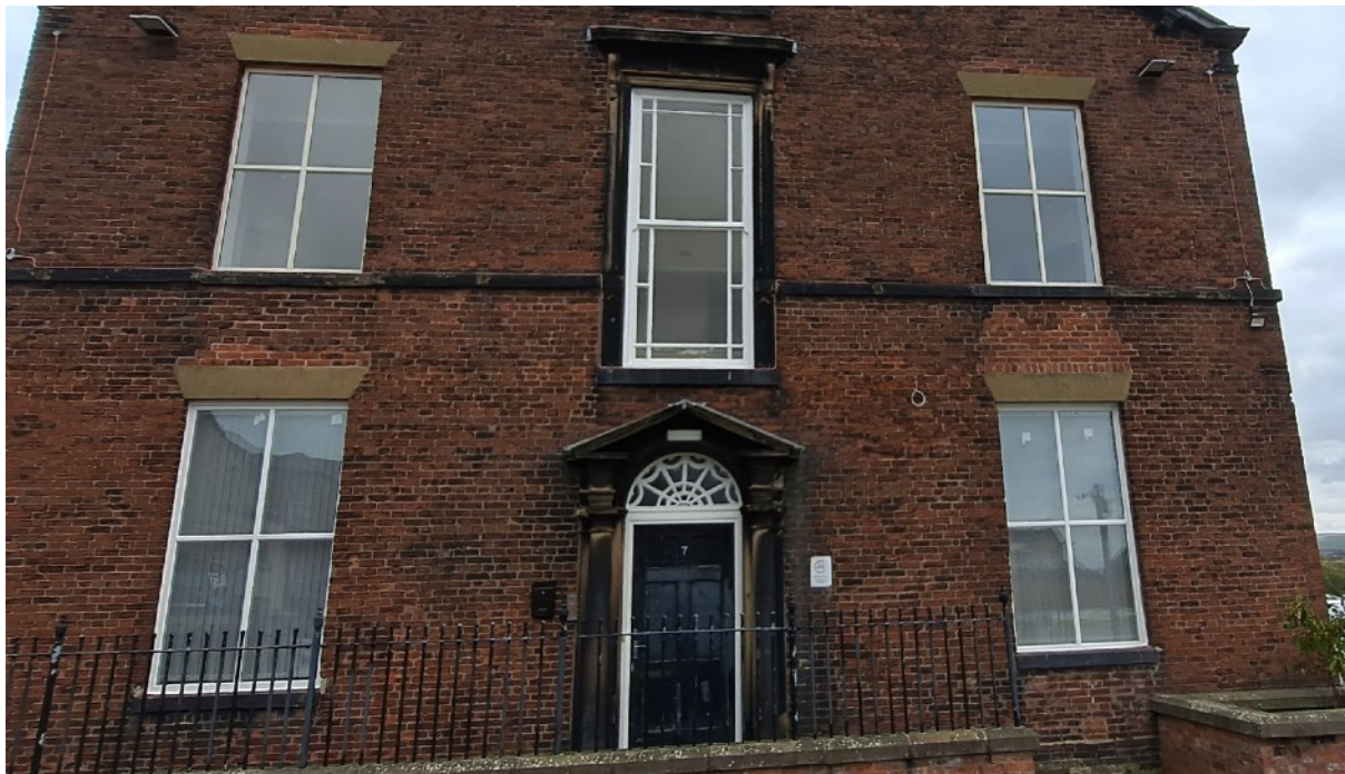
Plate 14: The main entrance to the house with attached Doric columns, fanlight and open pediment. Above is a large window with stone architrave, consoles cornice and marginal glazing bars that would have lit the first floor central corridor.
