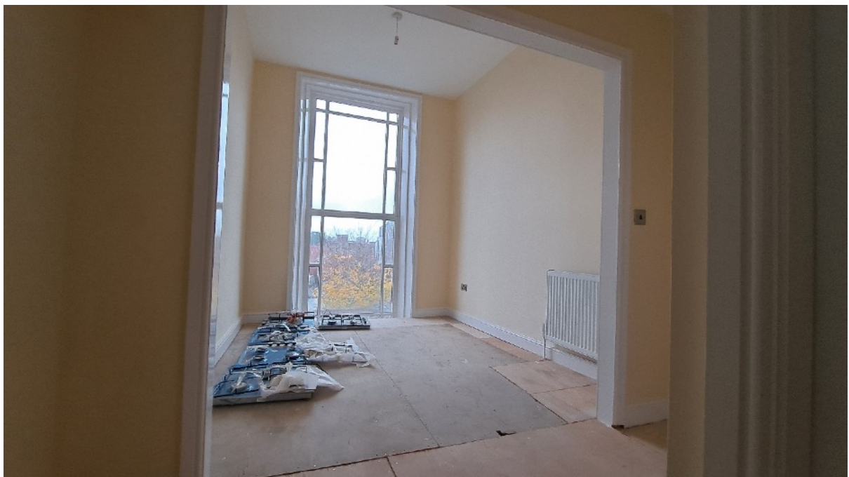
Plate 39: Former F11, an inserted staircase to the front of the building, now altered to form Room 1 Apartment 9. The original window with marginal glazing bars has been retained in its original surround
