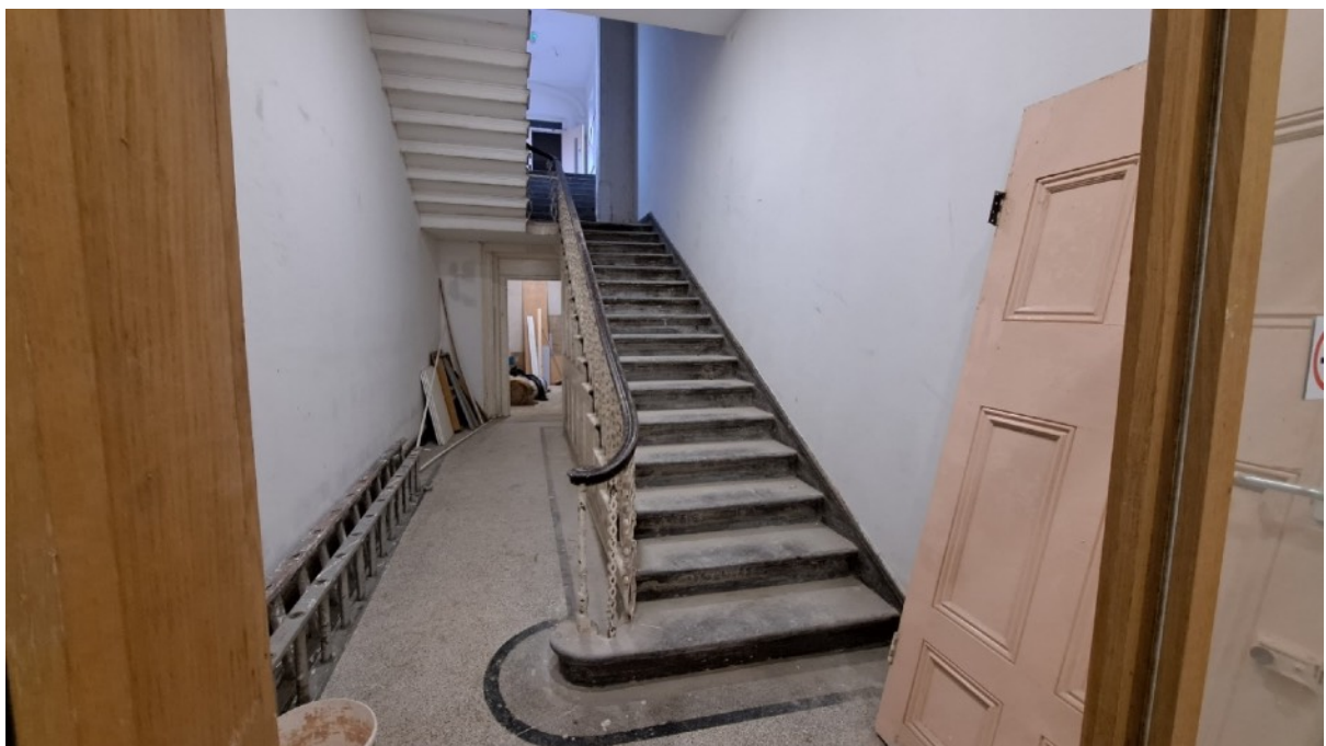
Plate 35: Original cantilevered stone stair with flag landing, cast iron balustrade and mahogany handrail, now part of CG02
