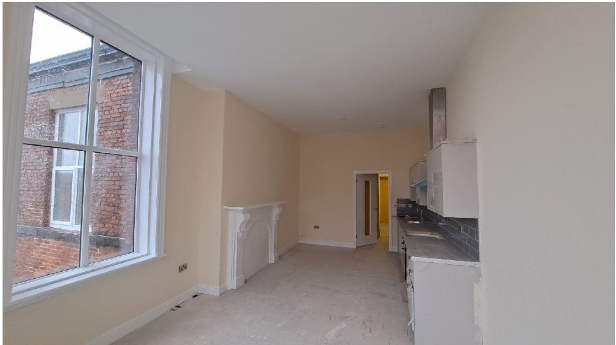
Plate 43: Former bedroom (F8) now subdivided to form Apartment 10, Room 5 above retains a fireplace. Modern windows in original surrounds have bulkheads
