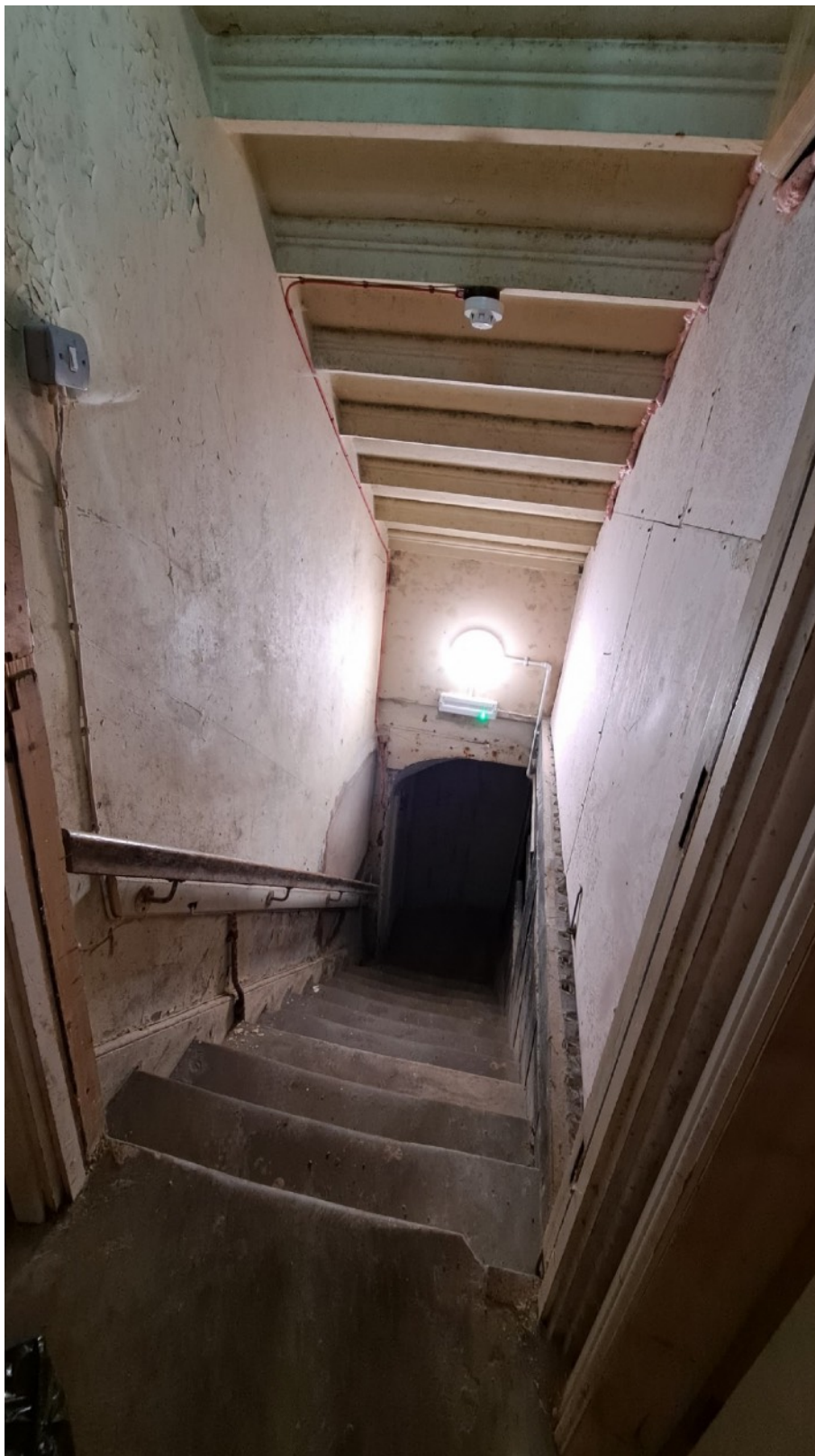
Plate 15: To the rear of the original house the stairs from CG02 to CB02. They are brick with stone flag treads and an original board partition to the side.
