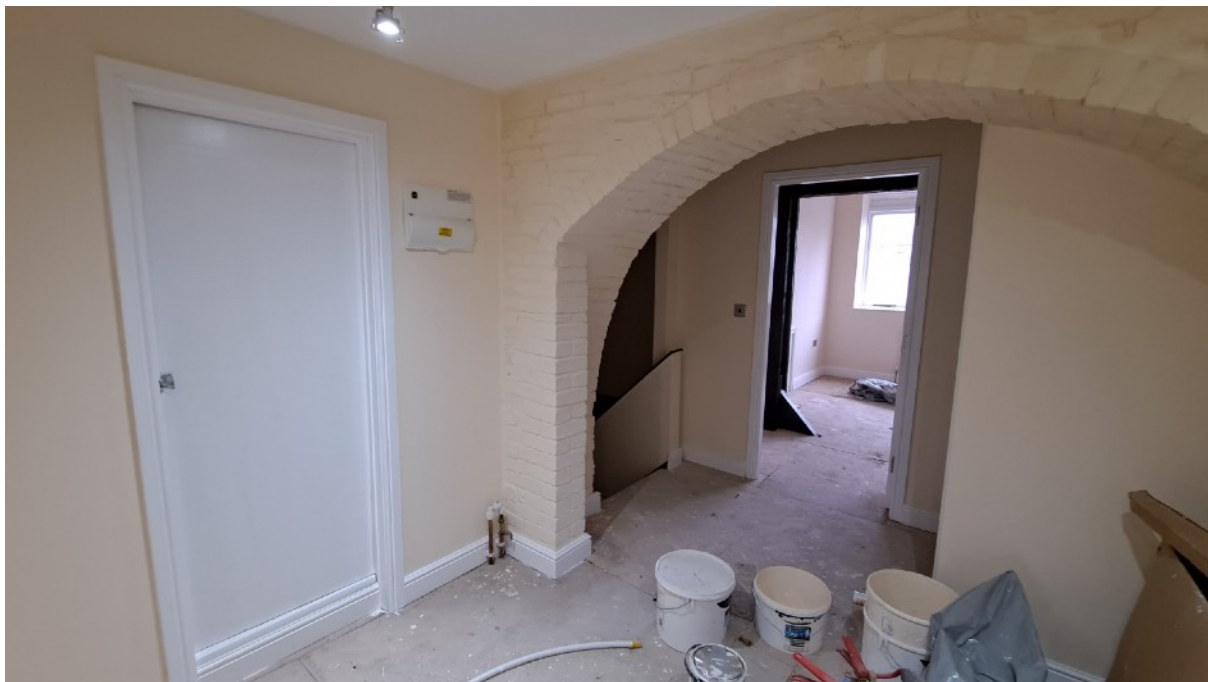
Plate 53: The attic stair, centre, leads into what is now Apartment 11, formed in the attic space
