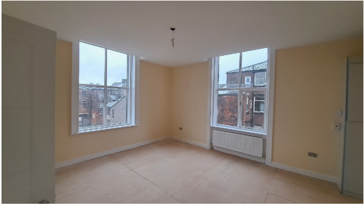
Plate 38: A former principal bedroom (F1) with retained window surrounds and panel with bulkheads. Now Room 3 of Apartment 9
