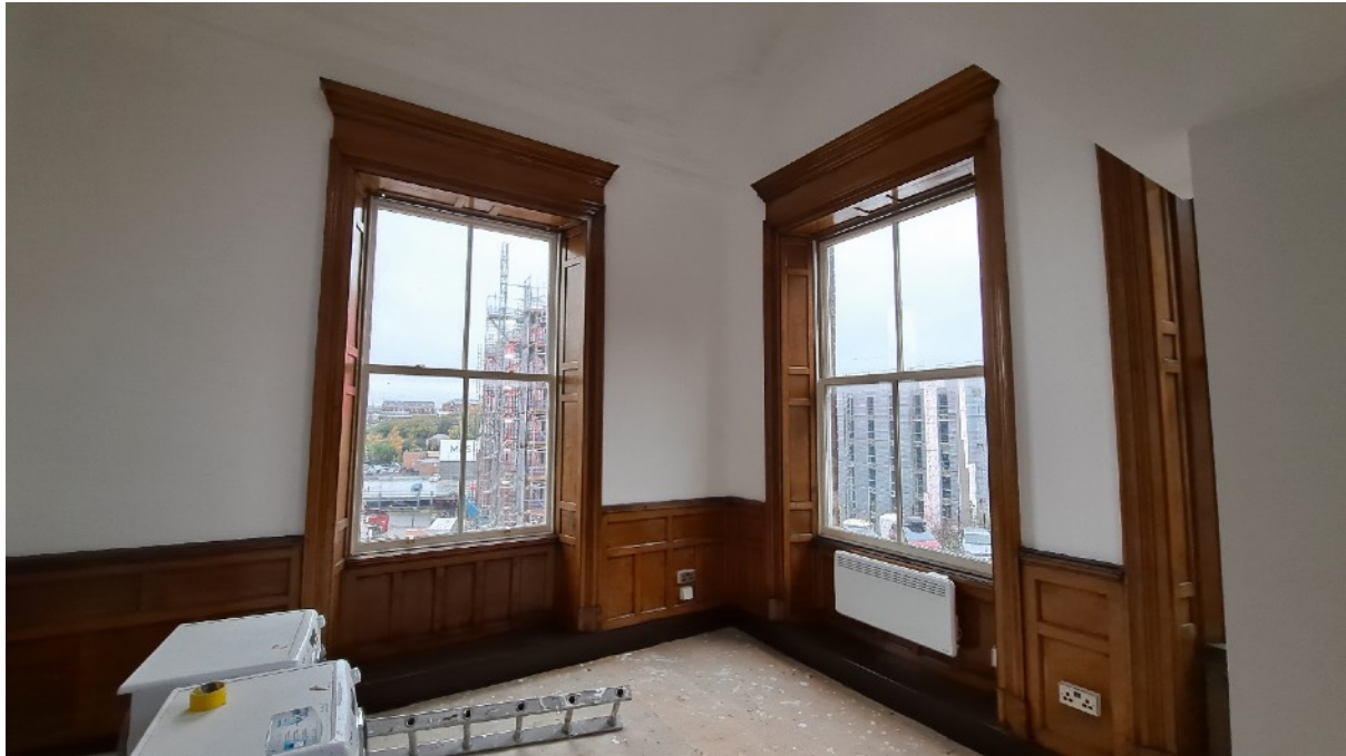
Plate 52: As with Apartment 13 original features have been retained in Apartment 12 but some windows have been replaced
