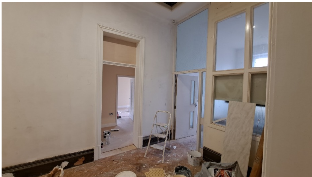
Plate 48: To the right the Manager's Office, with the original door surround retained for the entrance to Apartment 14 to centre
