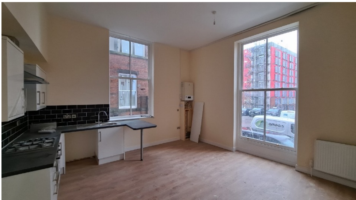
Plate 25: Originally a service room (Rooms G5,6 and 7) to G8, this room has had later subdivisions removed and now forms Room 2 of Apartment 6. It retains an original sash window and is accessed by a reopened doorway
