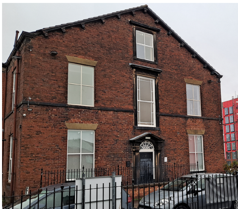
Plate 8: Main elevation of house from south. A typical gabled front to a Late-Georgian townhouse
