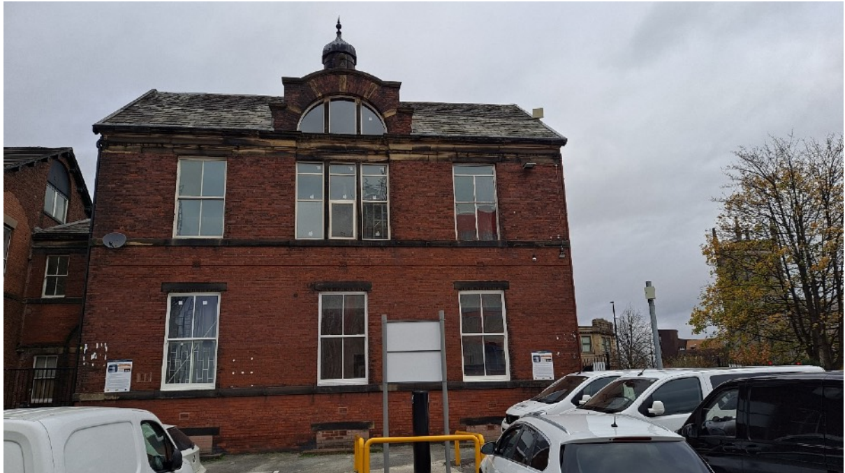
Plate 11: The extension building looking west
