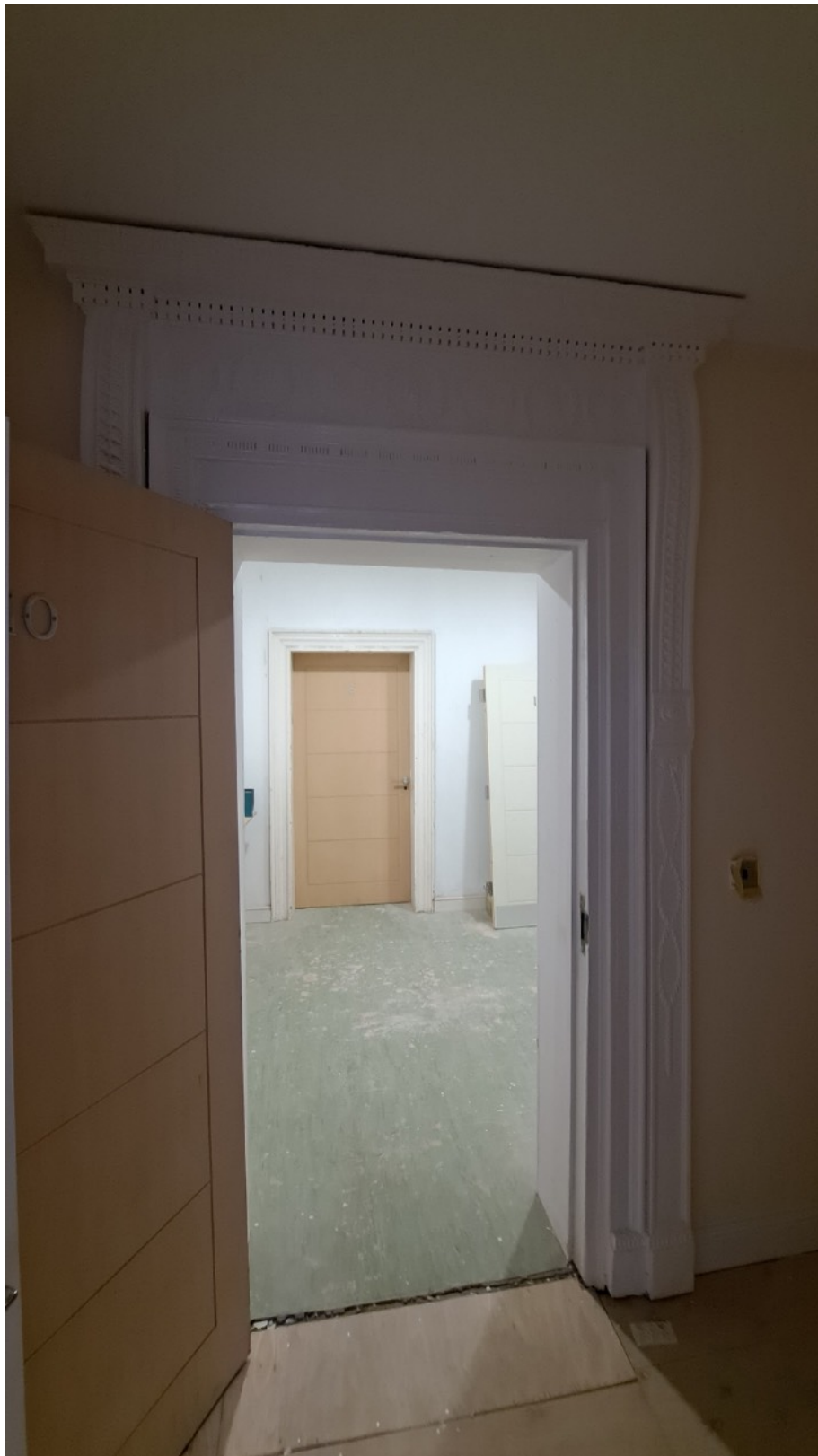
Plate 44: The original doorway to Apartment 10 has been retained, however, the six-panel door is replaced with a modern fire door
