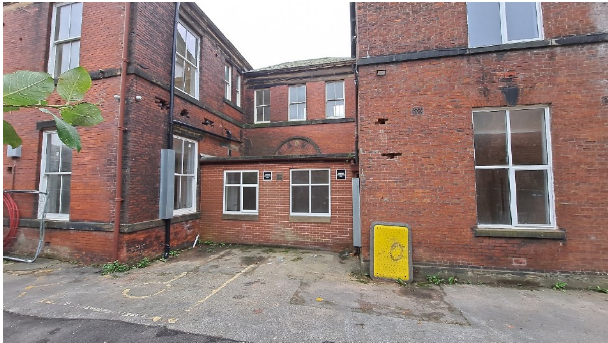
Plate 13: The link building from west with extension to left and house to right
