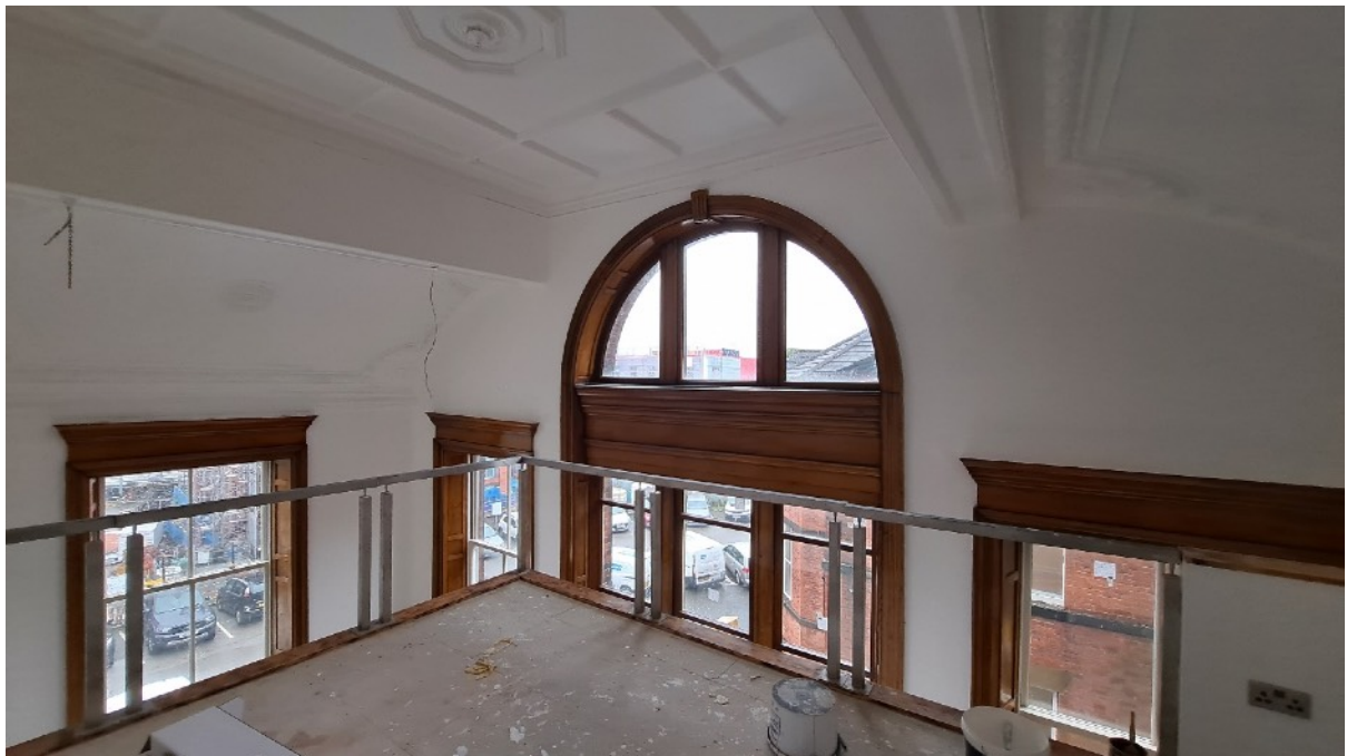
Plate 57: At the southern end of the Board Room (F22) a similar approach to Apartment 13 has been used to form Apartment 12
