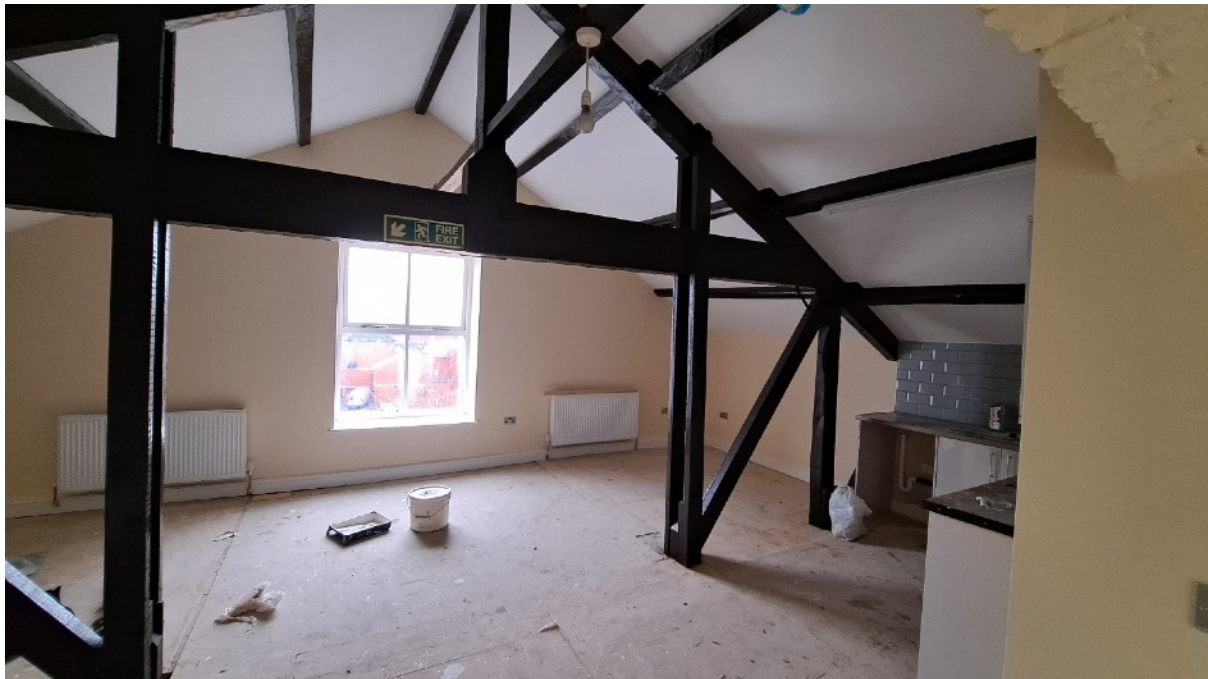
Plate 54: Room 4 of Apartment 11 is lit by the window in the front gable of the house
