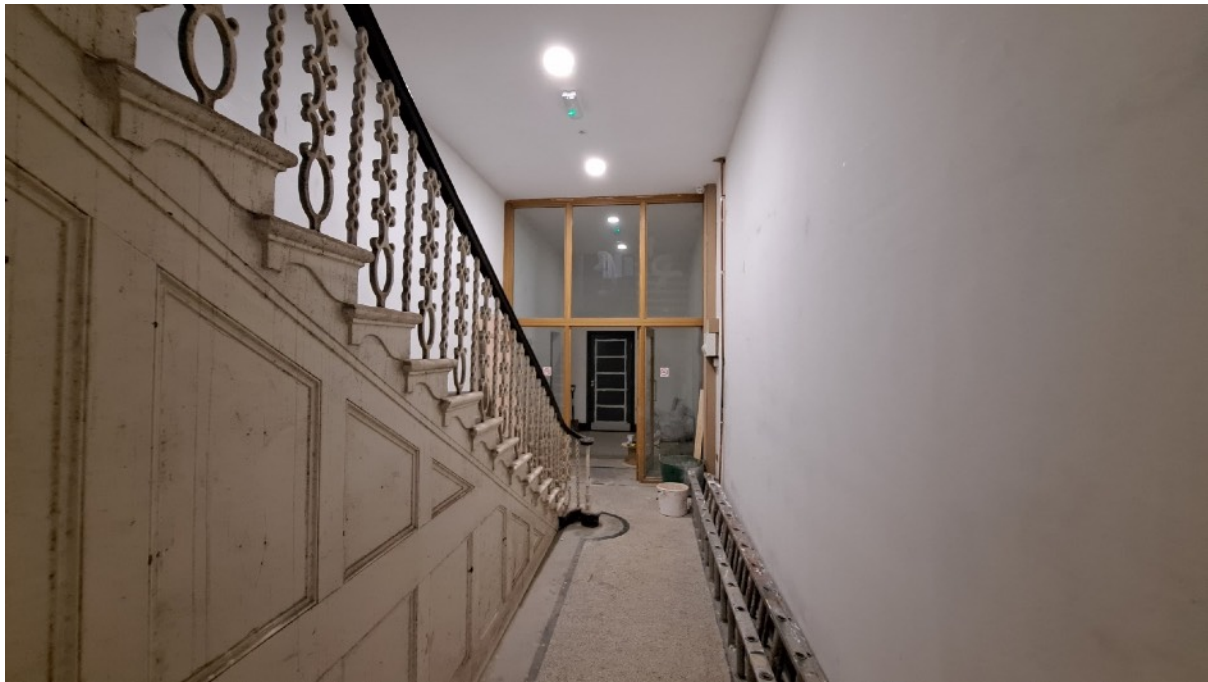
Plate 27: Formerly Room G4, the stairwell looking back along what would have been the central corridor to the house. Inserted plaster ceiling conceals original detailing, but scagliola floor retained. Now CG02
