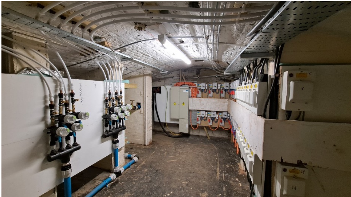
Plate 17: In general, the basement rooms, storage and service rooms are unaltered. Although the former storage room B5 now contains electrical equipment it appears to have retained its earlier bins.
