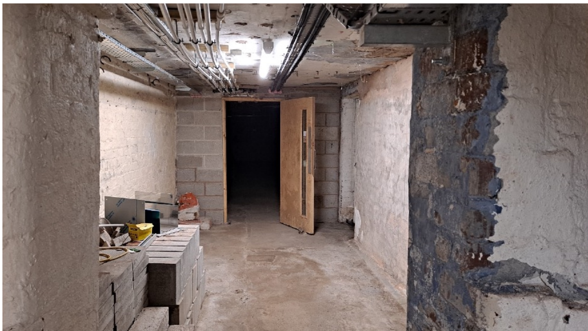
Plate 18: With the building of the extension the central basement corridor was carried through to the rear with Room B11. Another inserted wall now forms CB01 and CB10.
