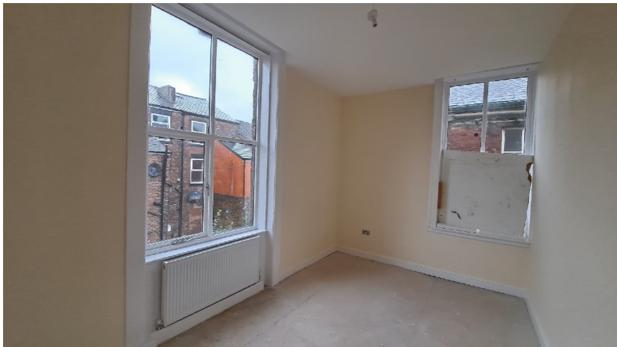
Plate 41: Formerly F3, subdivided to form stair to attic, now Room 4 Apartment 8 accessed through reopened historic opening. Original window surrounds and panel with new frames
