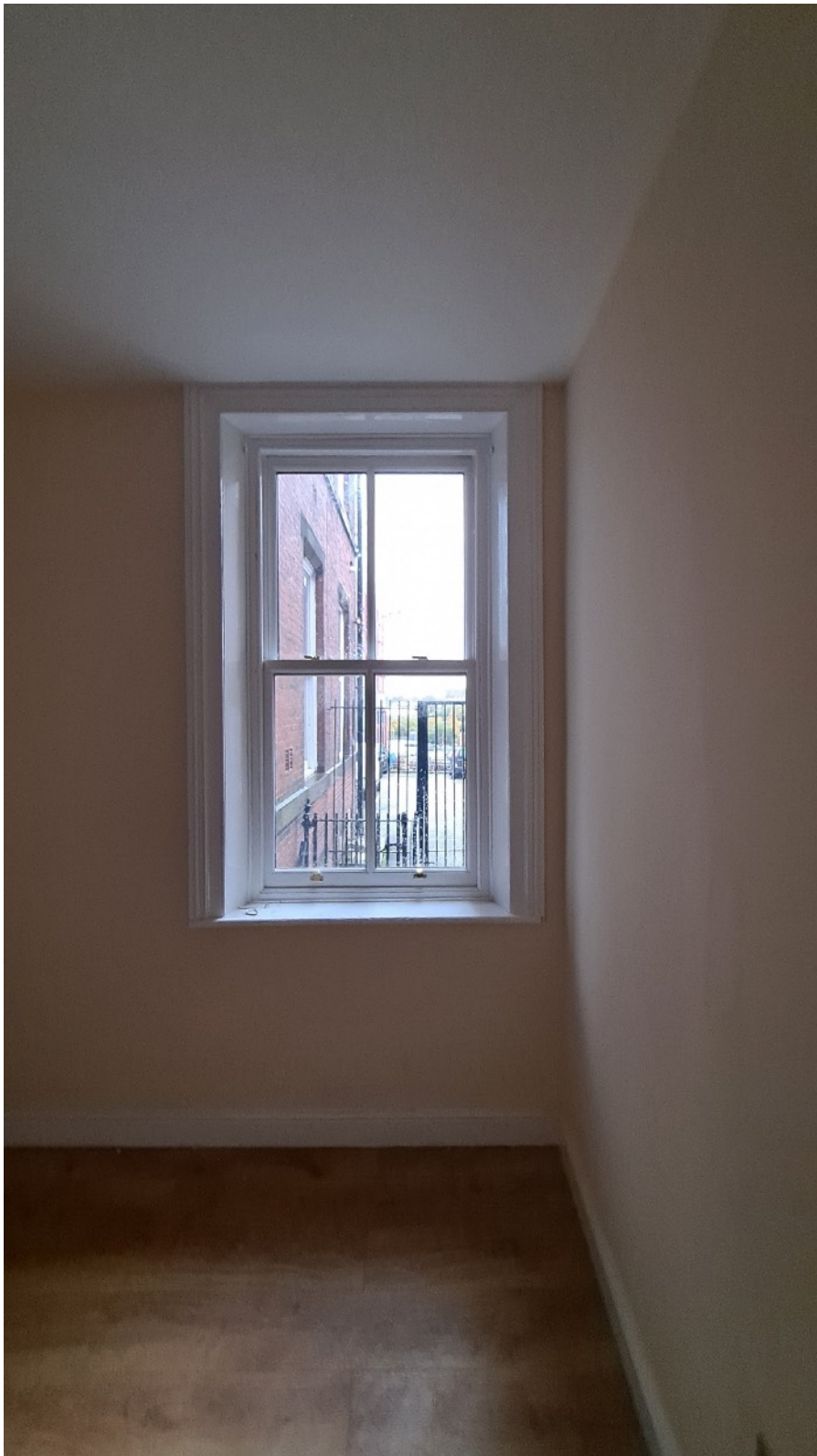
Plate 29: Sash window in original surround in Room 4, Apartment 4 formed by inserting wall to right to block G14
