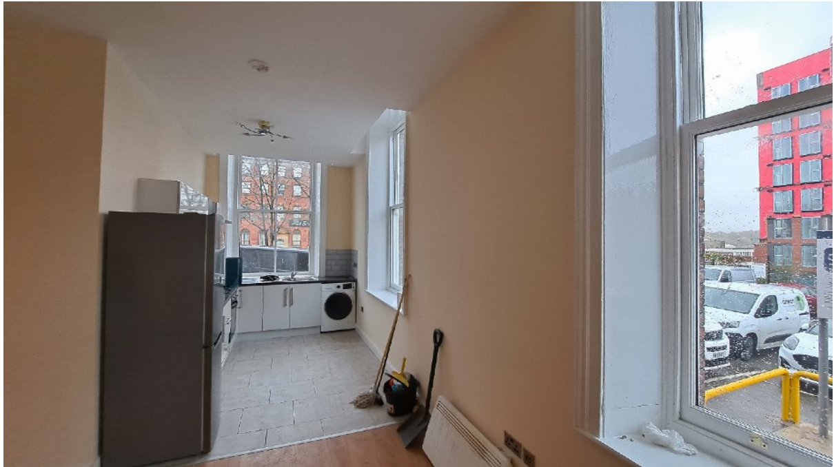
Plate 34: Formerly a suite of rooms (G25 to 31) formed from the subdivision of the probable waiting hall, now reconfigured to form apartments 2 and 3. Room 4 of Apartment 2 shown above with retained window surrounds with bulkheads
