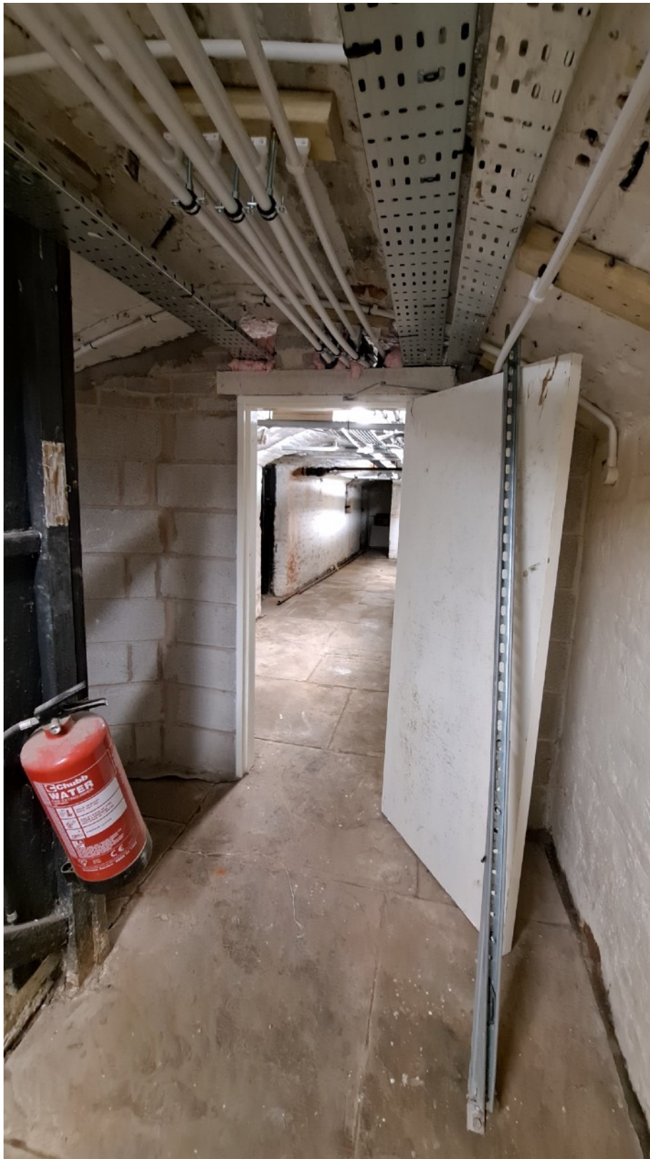
Plate 16: At the bottom of the stairs an inserted wall now forms CB01 and CB02 from the original B10.
