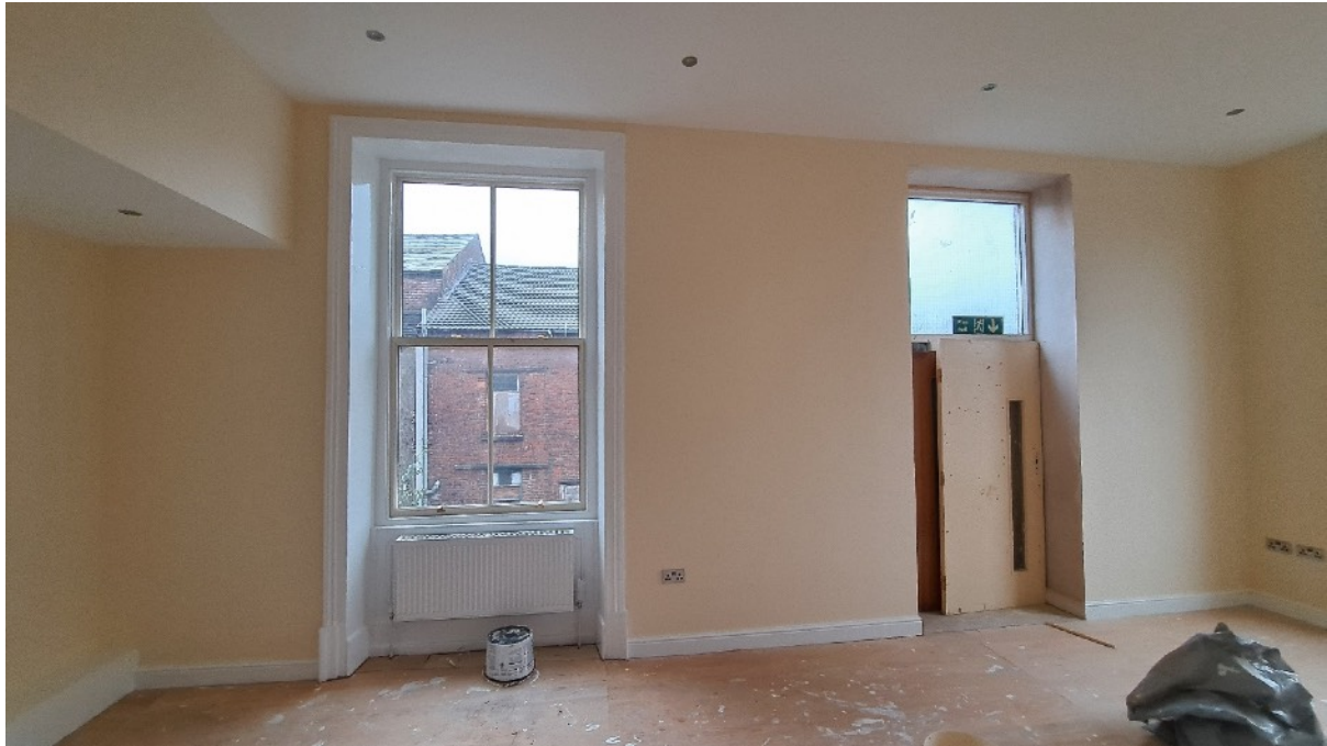
Plate 50: Former offices F16, 17 and 18 have had partitions removed to form Room 4 of Apartment 14, but the space has been subdivided to form Rooms 1 and 5
