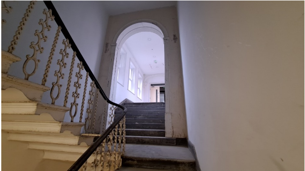
Plate 36: The opening to the link building first floor corridor CF03, possibly formed from the original stairlight at the rear of the house
