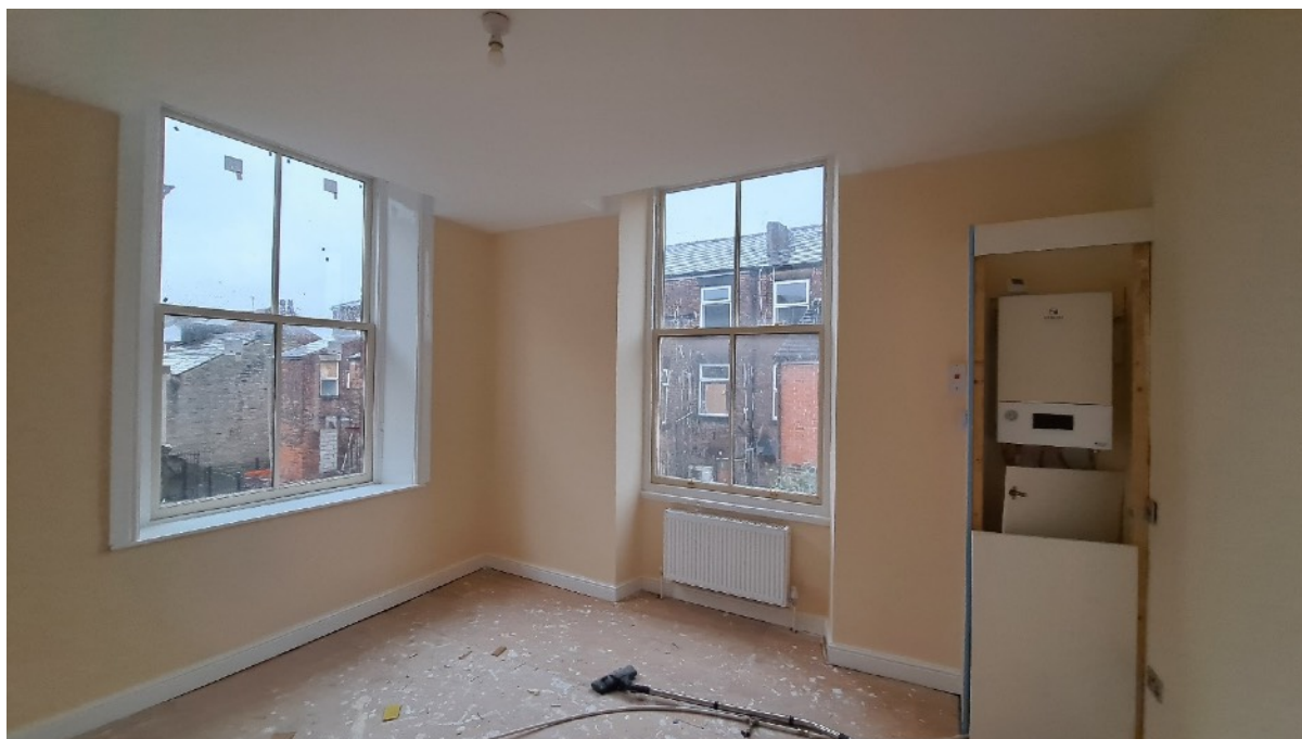
Plate 49: Former toilets (F14 and 15) with partitions removed to form Room 3 of Apartment 14. Window surrounds retained with modern windows
