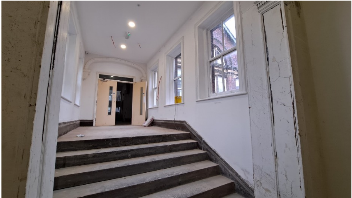
Plate 46: The Link passage and stair (F12), now CF03, was the original access to the Board Room and retains original features, although the corbelled arch has a modern inserted partition and door. Modern windows in original surrounds
