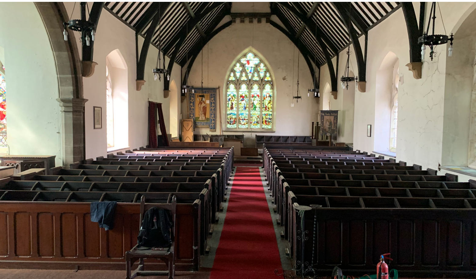
Figure 6 View East-east down Nave
