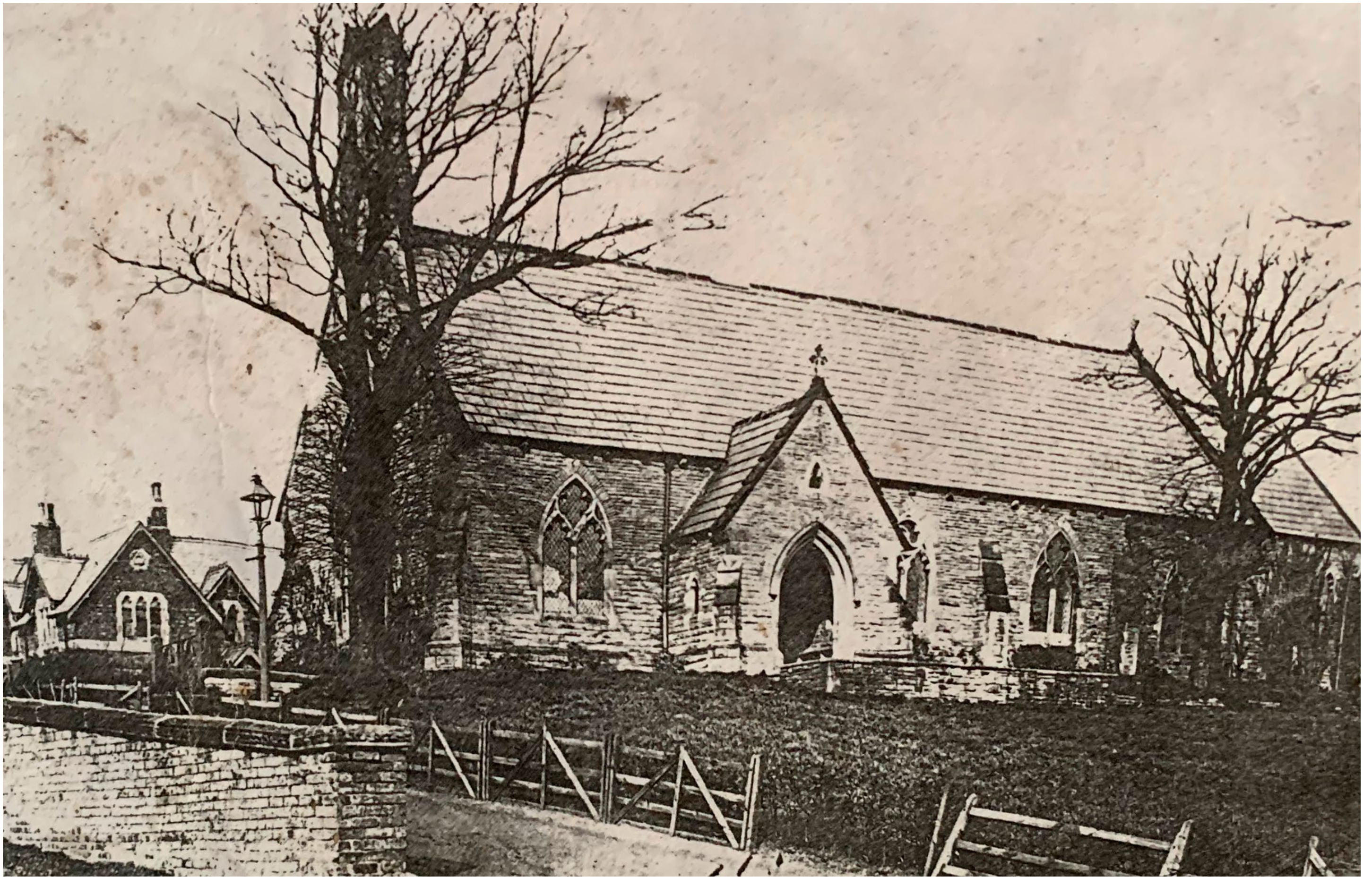
Figure 12 Historic Photograph of Holy Trinity, August 1899
