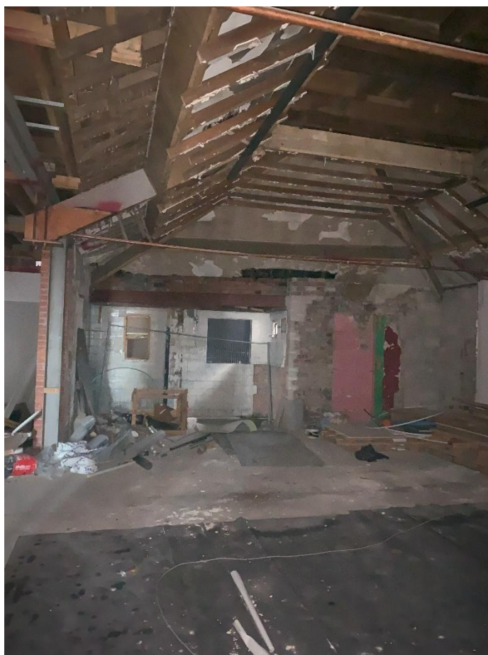
Figure 2.6: Internal view of the two storey rear element.
