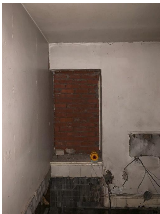
Figure 2.6: Subdividing wall abutting a bricked up window.
