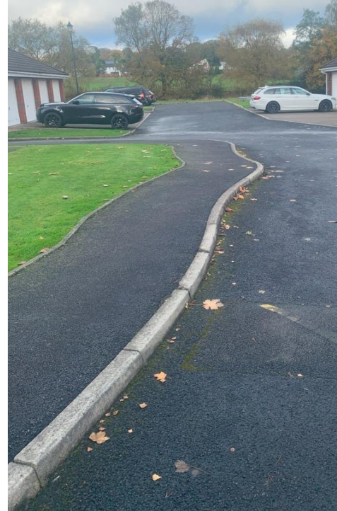
Photograph 6: Bamford Mews Existing Footway
