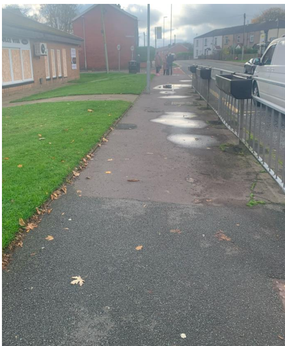
Photograph 7: Norden Road Existing Footways (facing south)
