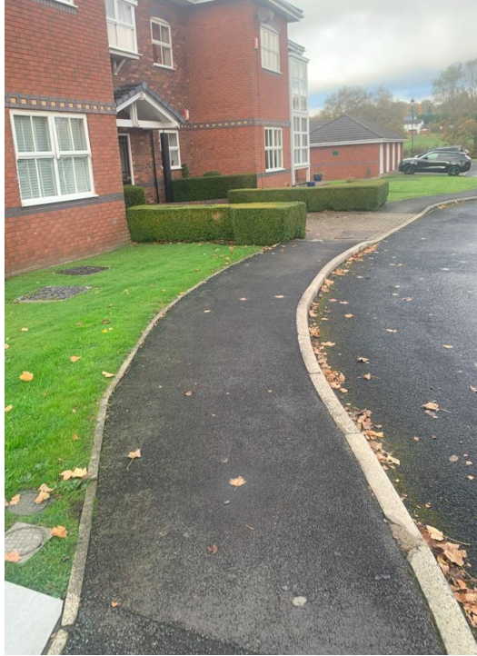
Photograph 5: Bamford Mews Existing Footway
