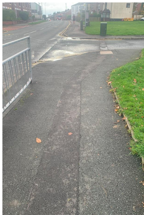
Photograph 8: Norden Road Existing Footways (facing north)
