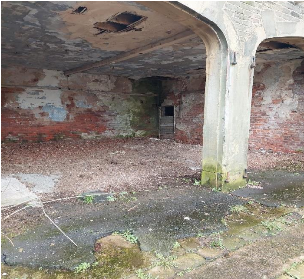
Photograph 1: Under open barn building
