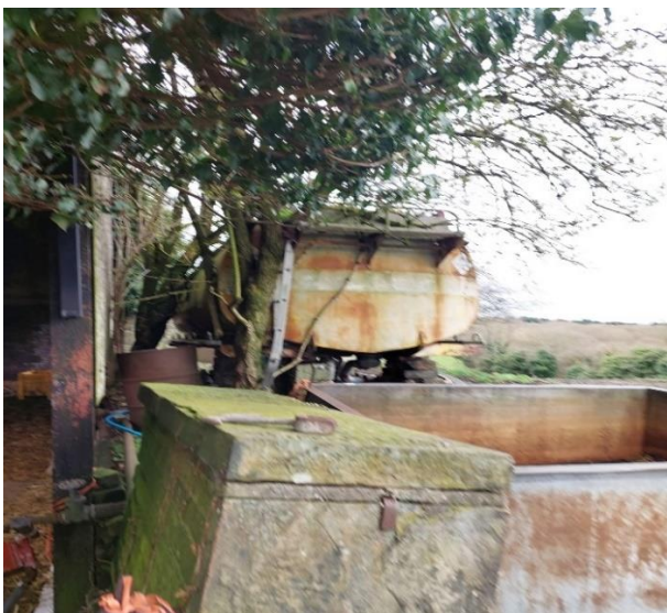
Photograph 5: Fuel tank adjacent to south side of new barn
