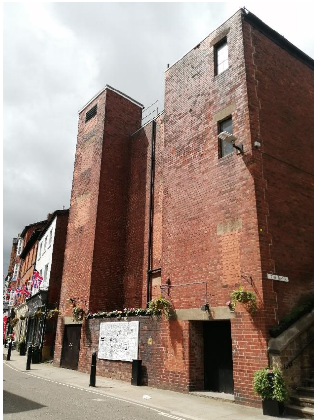
Figure 2.6: Baillie Street frontage.
