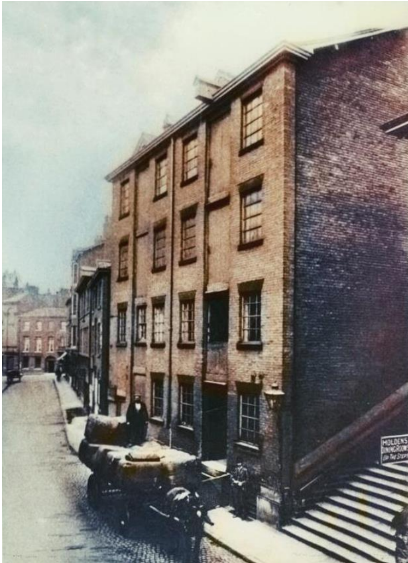
Figure 2.3: Image showing the Baillie Street elevation. Understood to be 1902 when the building was in use as a warehouse.
