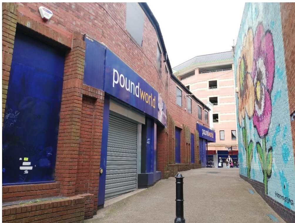
Figure 2.7: Eastern elevation taken from The Banks.
