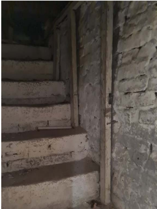
Wall between workshop and lounge
