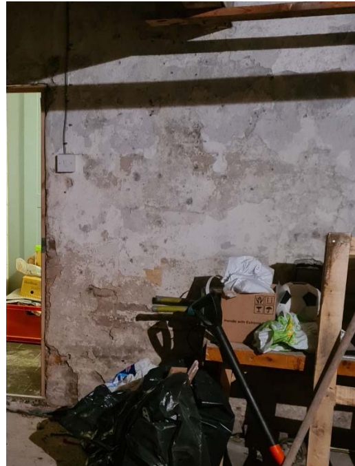
Wall between workshop and storage
