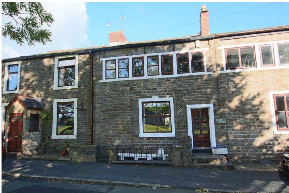
View of the Front (West) Elevation
