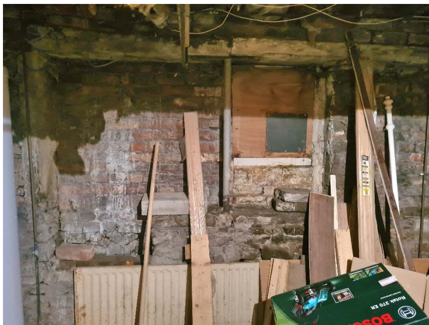
Extent of bricked up rear door
