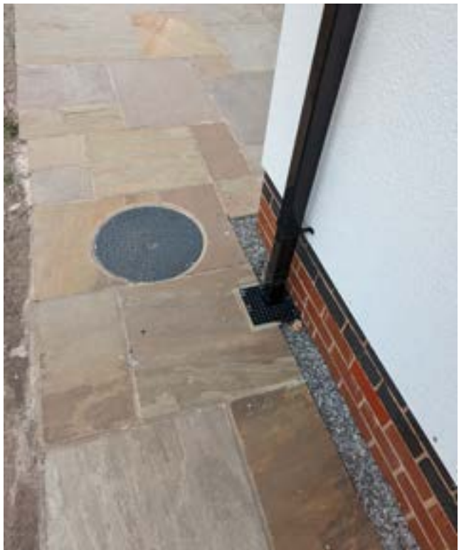
Existing drainage inspection chamber
