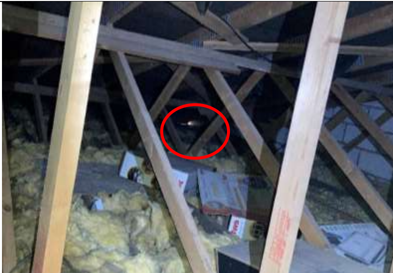
Figure 13: Showing cross laid timber structure in internal void 1 and daylight permitting into the void through the southern elevation.
