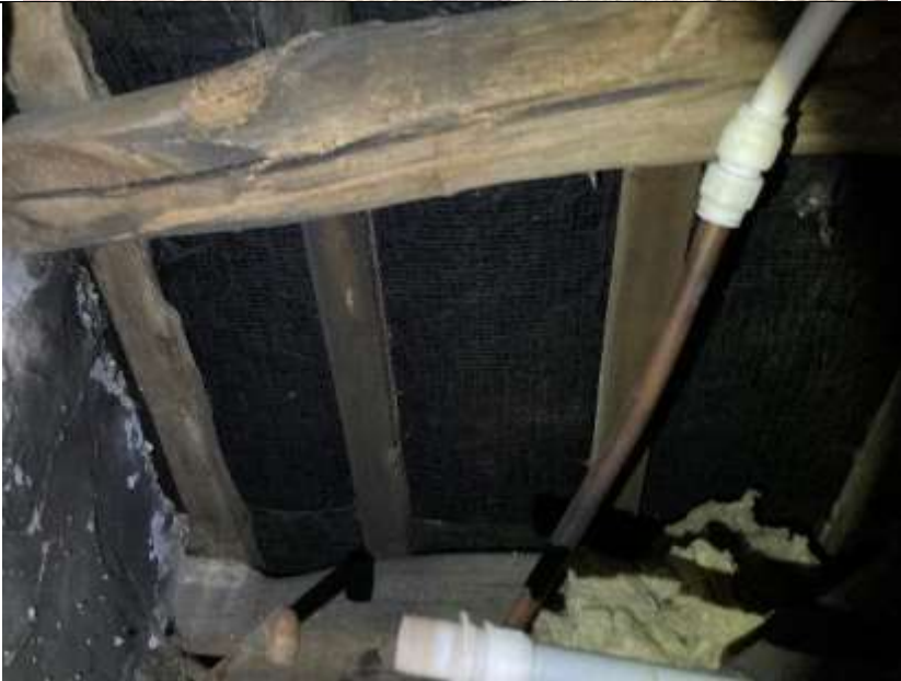
Figure 16: Showing the log timber ridge structure present in loft interior 3 and 4.
