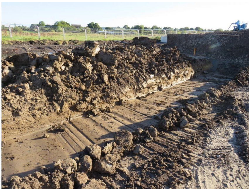
Plate 9: Watching brief trench, looking north-east (no scale)
