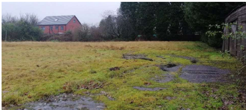
Plate 11: Existing Moss Covered Tarmac
