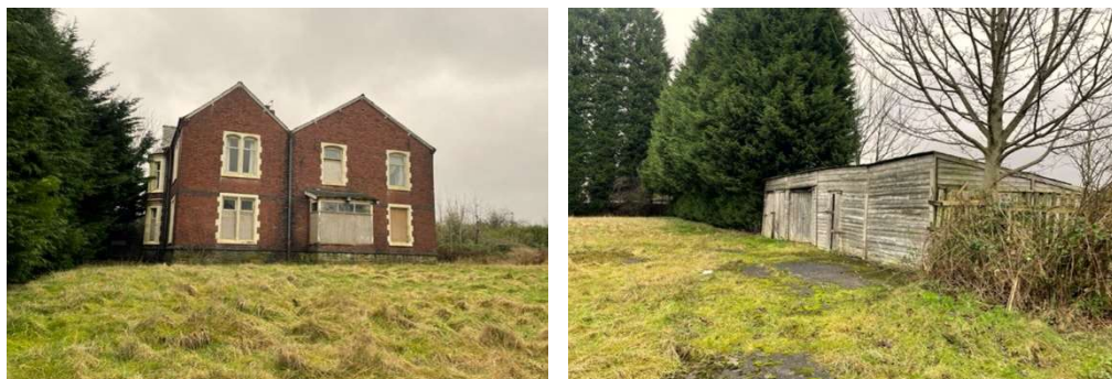
Plate 9 & 10: Existing Dwelling and Garages
