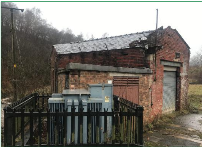
The south elevation of the structure
