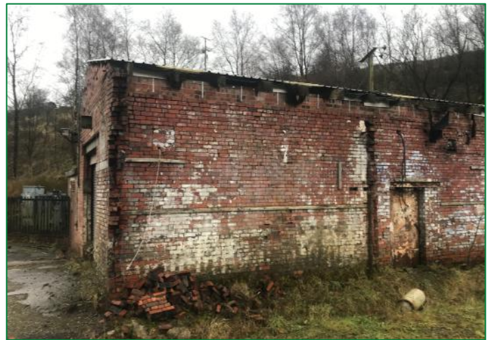
The north elevation of the structure
