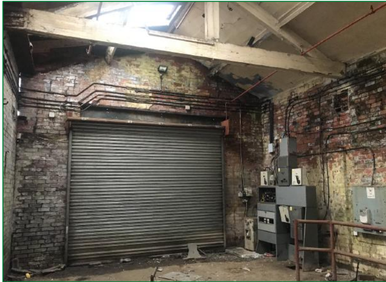
The interior of the structure
