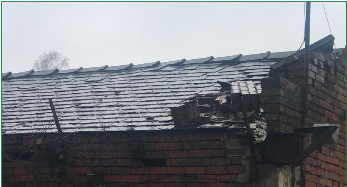
Slates on the southern side of the roof
