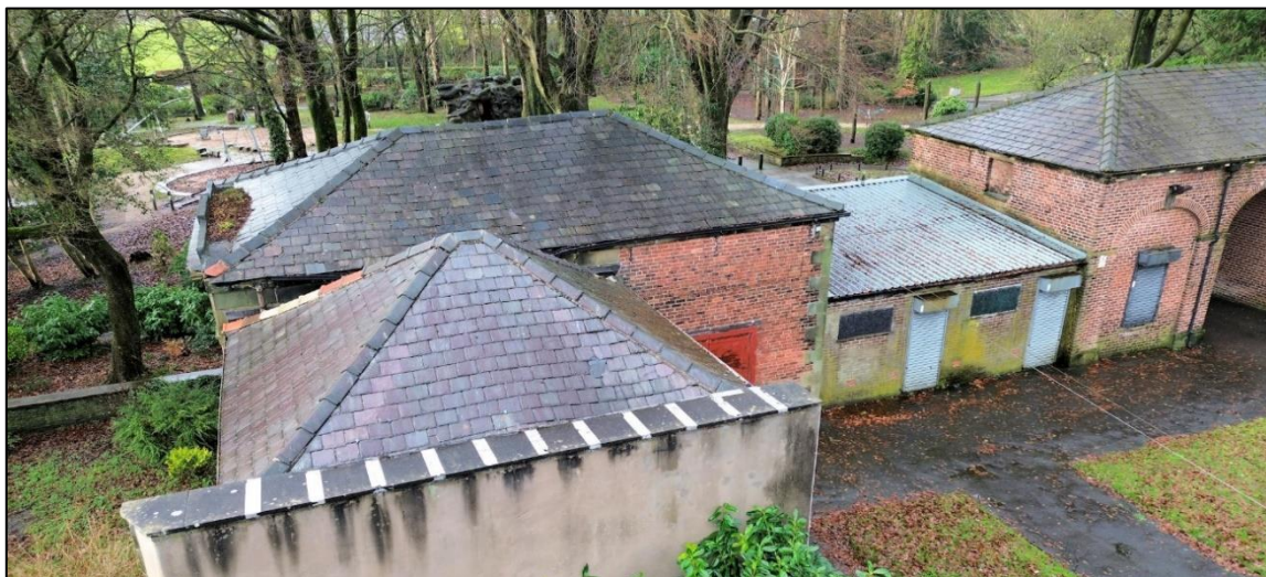
Plate 3: General view of the roof of the buildings to the west of the site.
