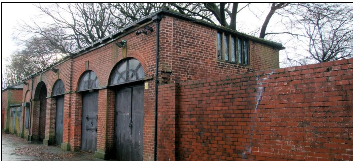
Plate 10: The brick and stone blockwork walls themselves were generally intact.
