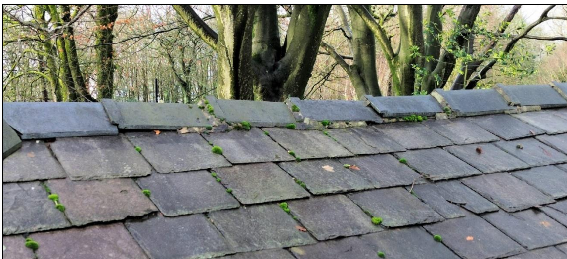
Plate 4: The roof ridges were intact but had gaps beneath the tiles that offered roosting opportunities.
