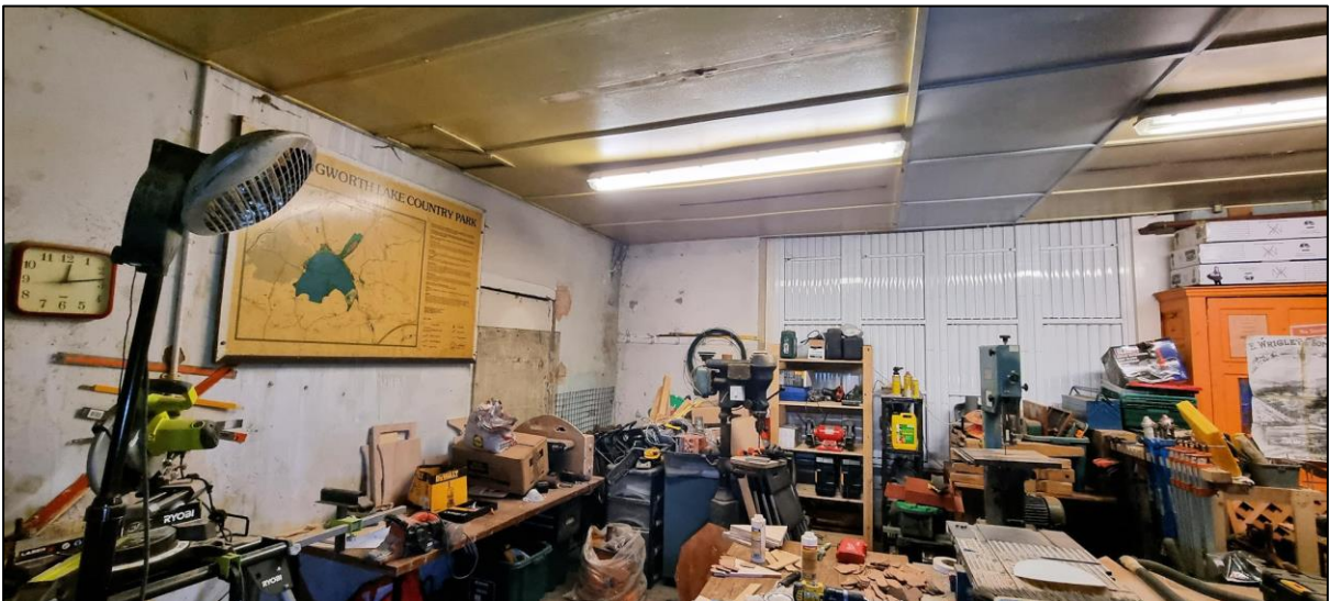
Plate 24: Similarly, the suspended ceiling of workshop was intact.
