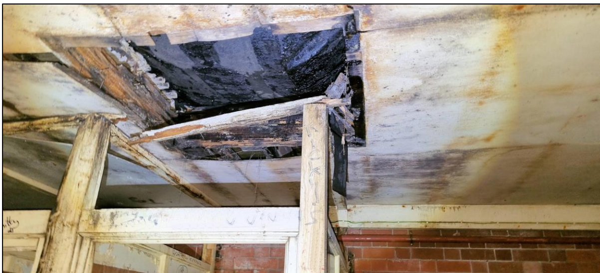
Plate 19: The underside of the roof of the toilet block was not visible due to the plastered lath ceiling.
