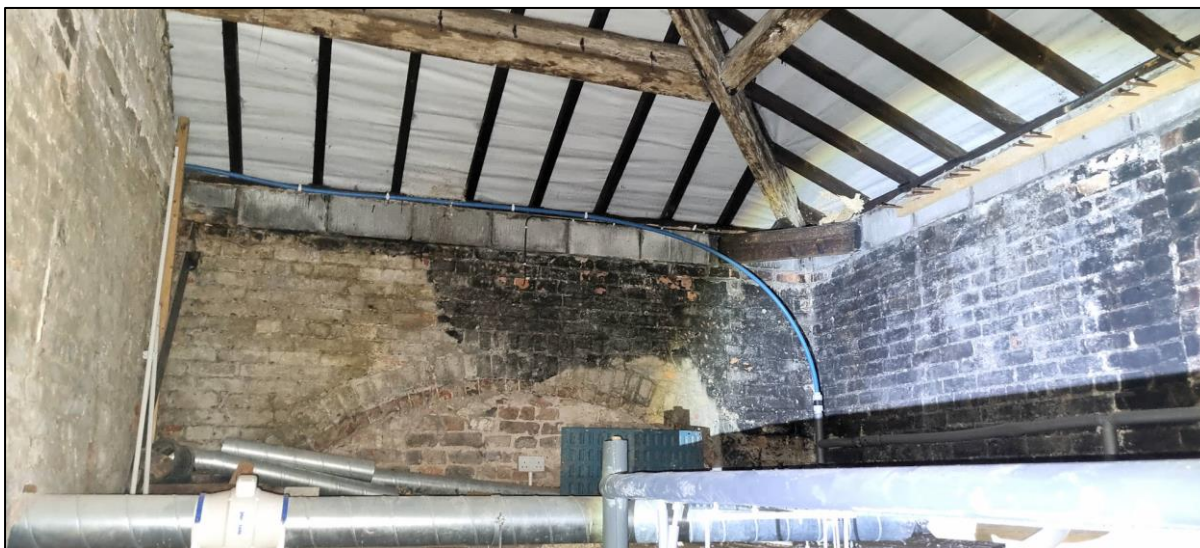
Plate 16: The southern end of the Playbarn had a roof void open to the roofing timbers and membrane.
