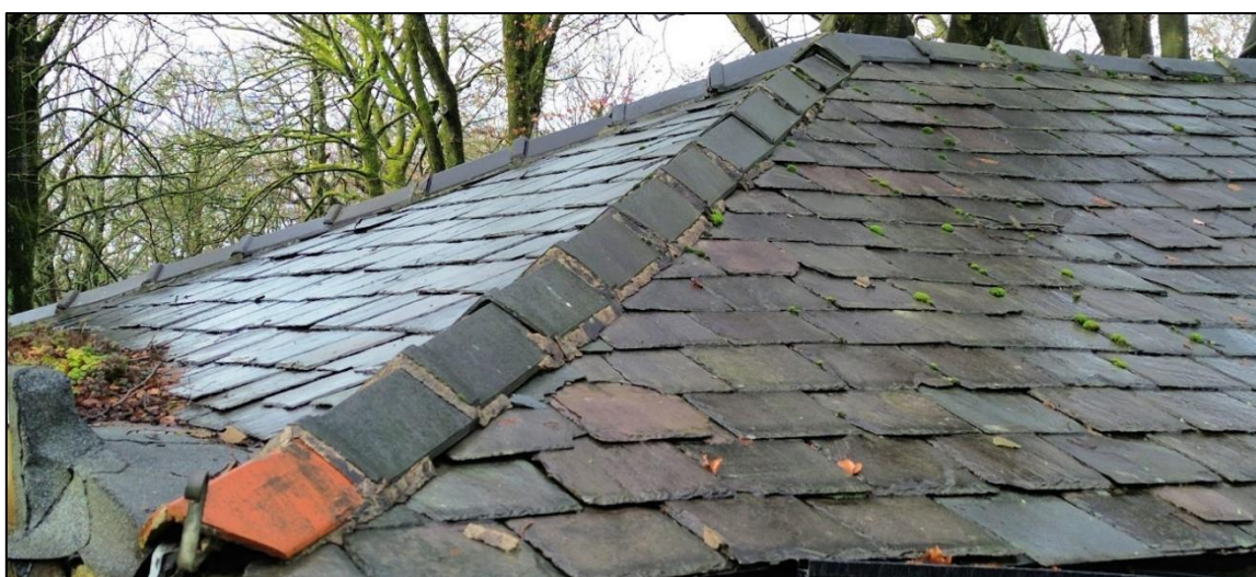
Plate 5: Similarly, the hips had small gaps apparent offering potential.
