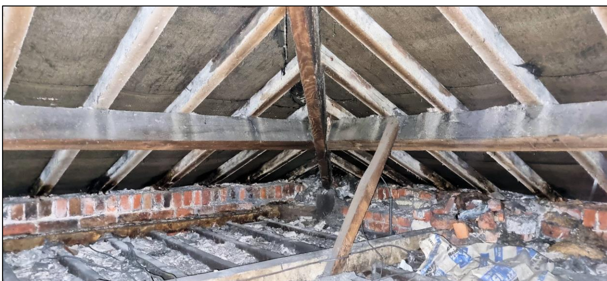
Plate 17: In the west pavilion the roofing timbers and roofing felt were exposed.
