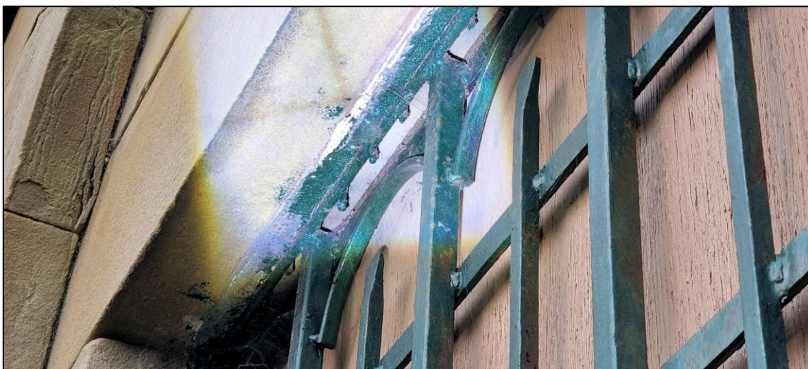
Plate 14: The window and frames had no significant gaps and offered no roosting or access potential for bats.
