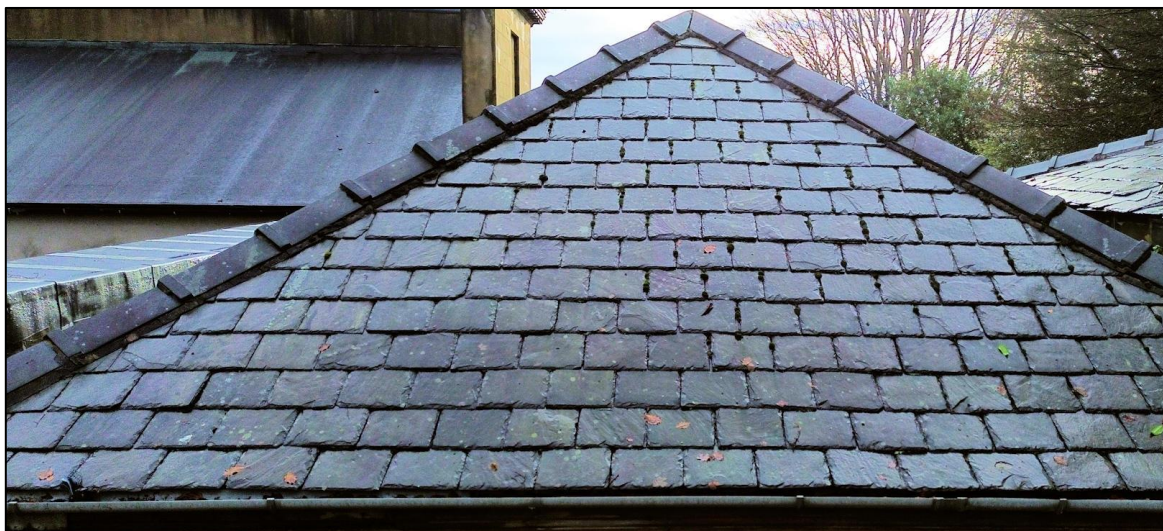
Plate 6: Many of the pitches were intact with no slipped or missing tiles.
