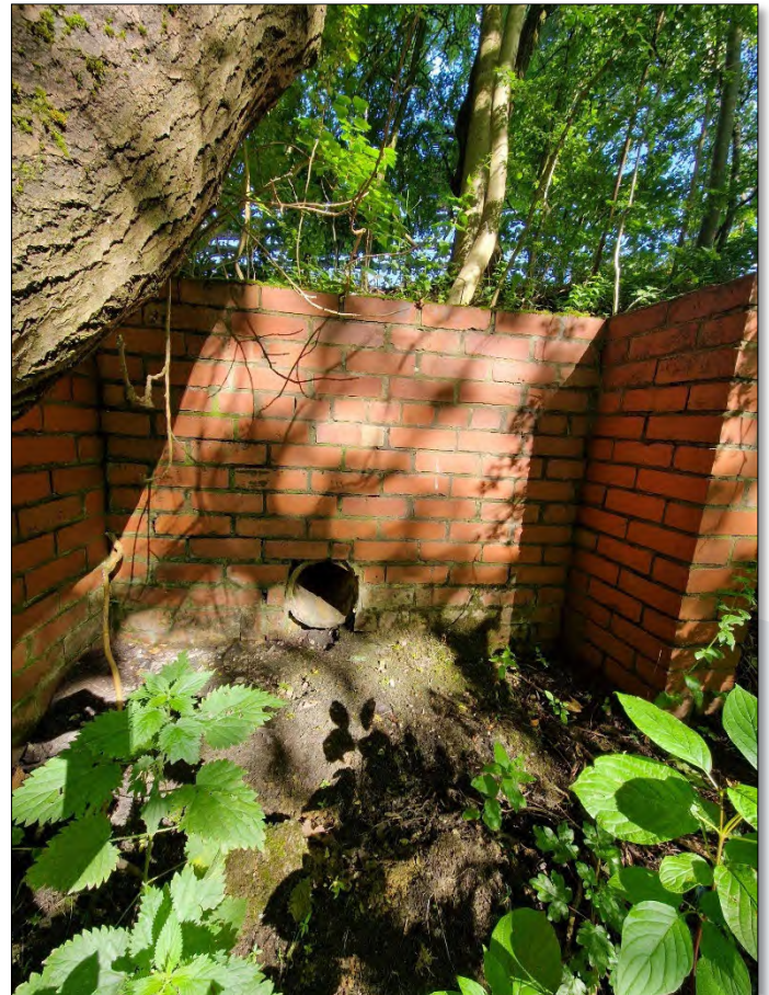
Pond Inlet Headwall
