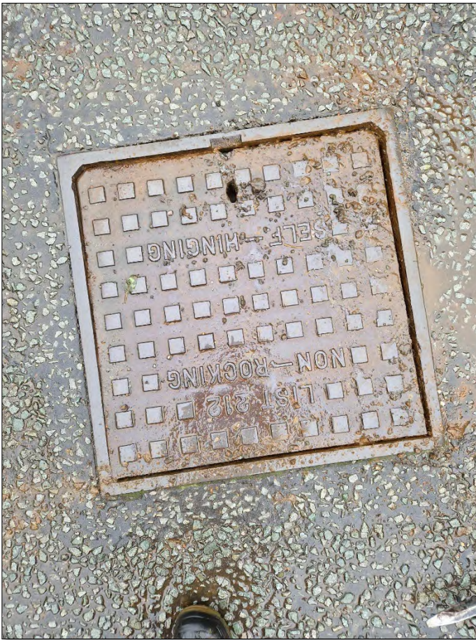
MH2 Cover Condition View
