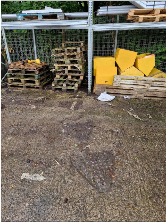
Petrol Interceptor Location View
