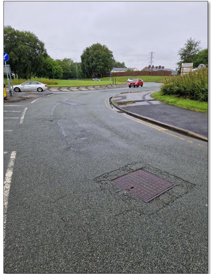
Manhole S8 Location View
