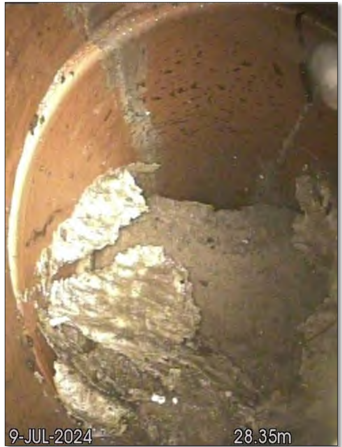
PI Upstream Pipe Condition View
