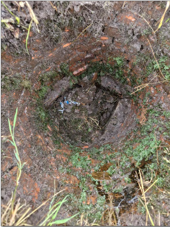
MH3 Internal View During Clearing
