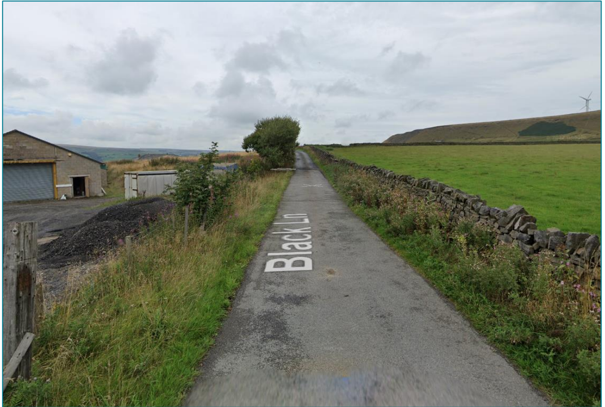
Figure 2.4: Existing condition of Black Lane
