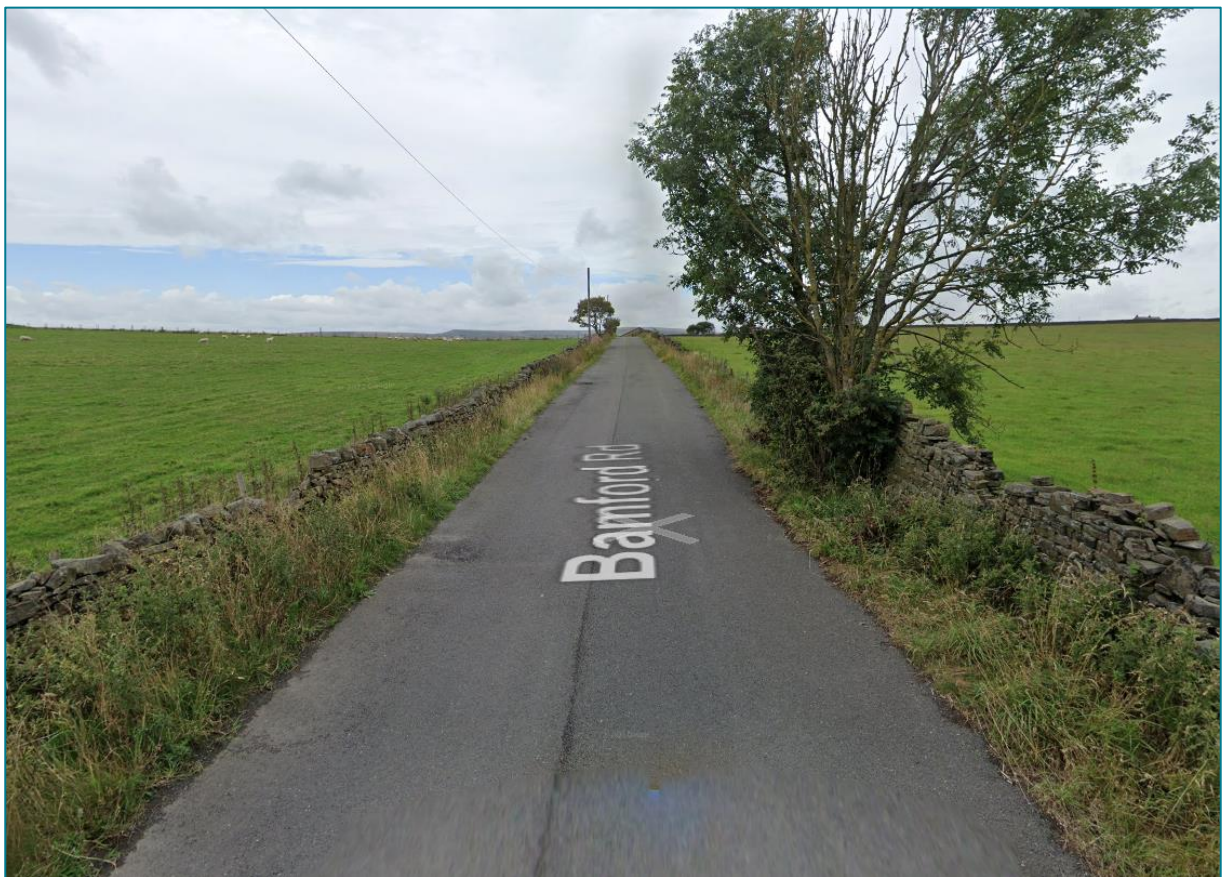
Figure 2.3: Existing condition of Bamford Road
