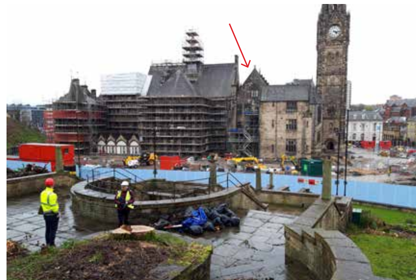
4.5 Location of Roof R2d on South-East Elevation
