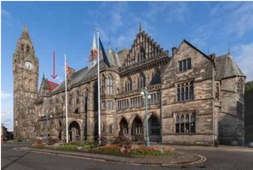
3.2 Location of roof R2d
