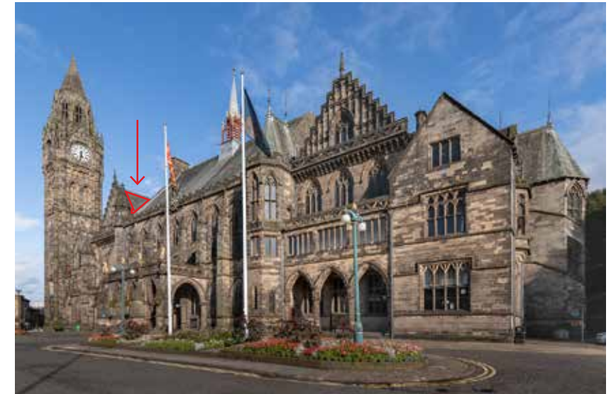
4.4 Location of roof R2d
