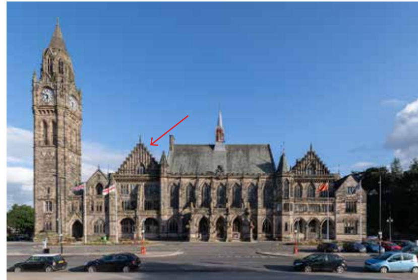
4.3 Location of roof R2d on North-West Elevation
