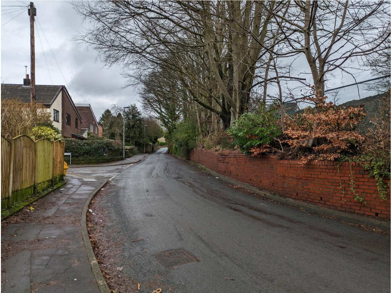
A view of the retaining wall and the trees along Marland Old Road.
