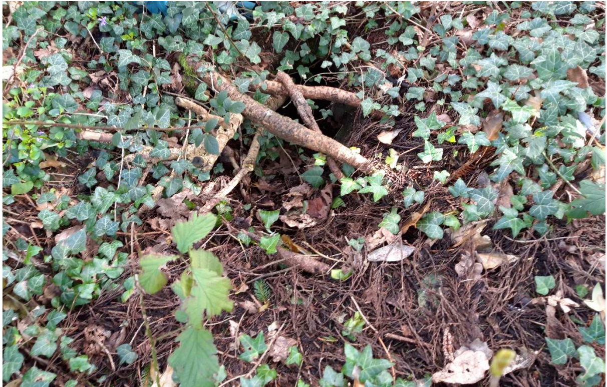
Photo 1: Inactive mammal hole on the southern boundary.
