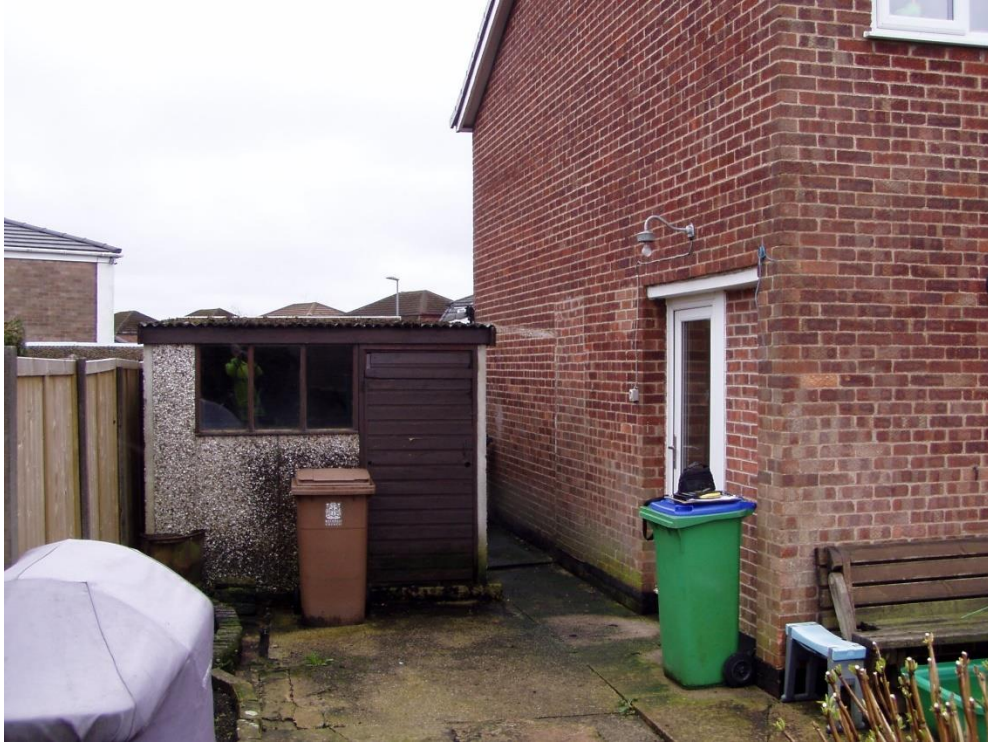
Side of property (viewed from rear).
