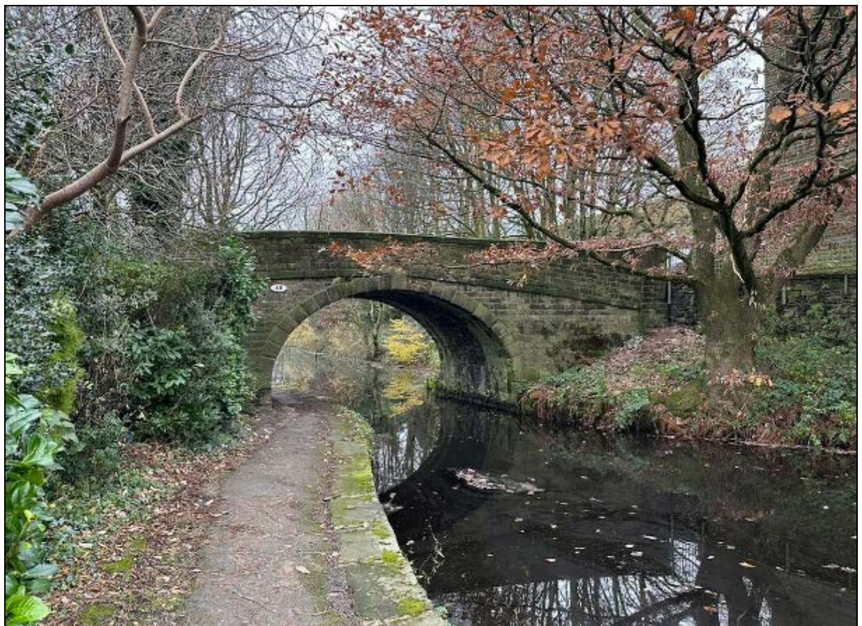
9. The bridge, viewed from the towpath northeast of the Lock House
