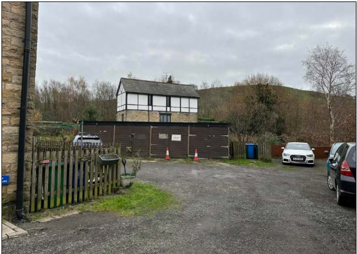
8. The building viewed from Brook Street to the north
