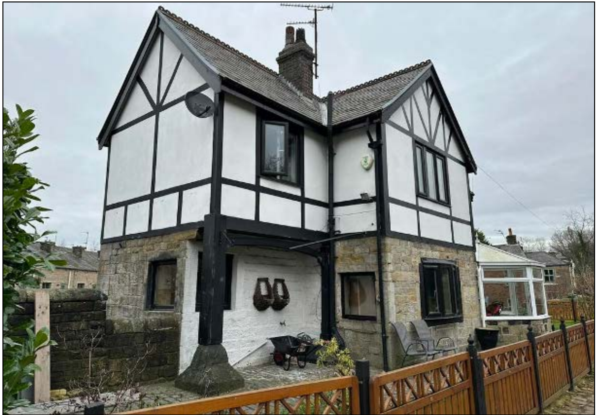
5. The property viewed from the west, showing jettied first floor left of projection
