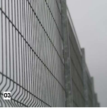
03 BOUNDARY SECURITY FENCE Typical Paladin Fencing: The perimeter of the service yards will be provided with 2.4m high paladin fencing. Post and panels to be black finish. Fences to be suitably set back from vehicular areas to reduce risk of accidental impact. Fencing / landscaping to be co-ordinated such that a maximum gap beneath fence is 100mm.
