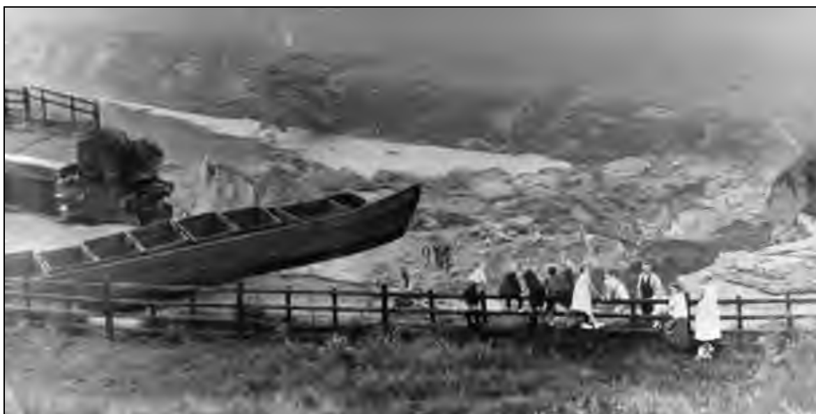
Figure 2-4: The 1936 canal breach from the North Bank
