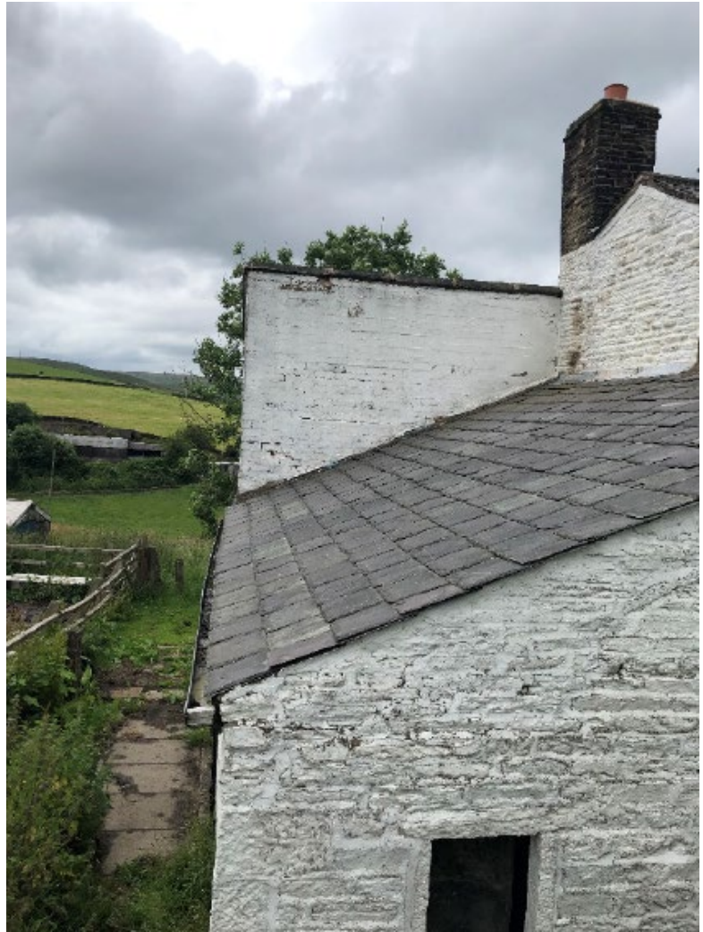
Workshop building; note the quoin stones on the external corner.
